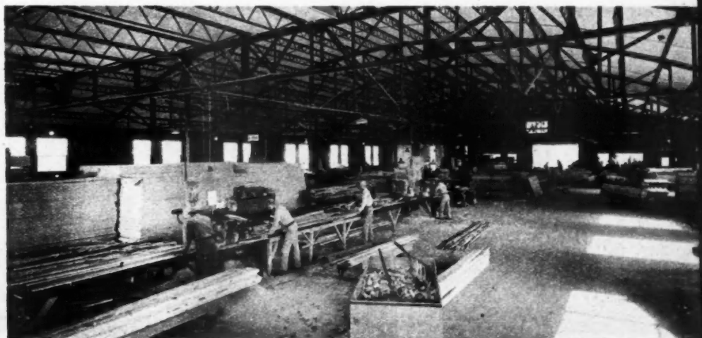
UP to five houses per day can be precut and panelized in this modern 90x215-foot clear span steel and masonry building
