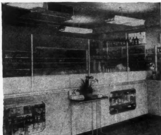
Connie's Prescription Shop, 1209 North Walker, Oklahoma City, Oklahoma, is kept comfortably cool in summer, warm in winter by the Servel All-Year Gas Air Conditioner . C. J. Masterson, proprietor, reports, "Our Servel Conditioner has been 100 per cent satisfactory."
