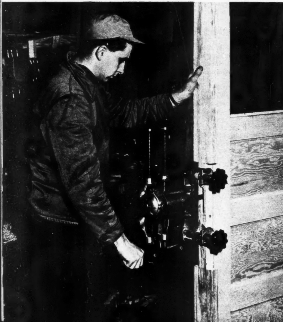
CARPENTER routing recesses for butt hinges on door using adjustable templet for position
