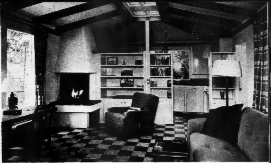
LIVING ROOM shows demising roof supported by 4x6-inch beams around a central panel. Each room has a similar structural ceiling. No plaster is used, wall and ceiling tint applied direct to inner face of concrete
