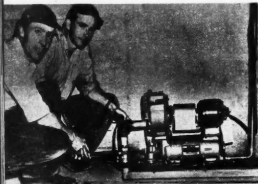
THIS Gould Balanced-Flow pumping unit is installed in each house to supply water
