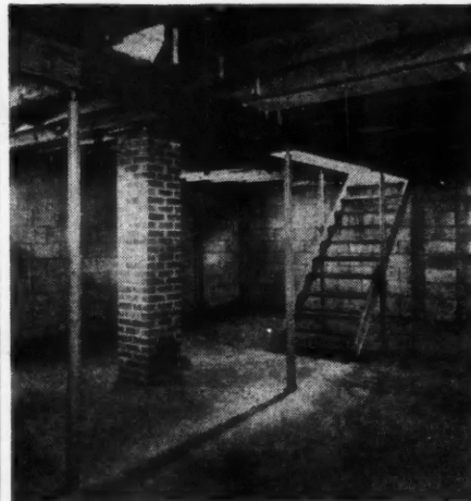
TEL-O-POST, used for bracing of beams and joists in basements of homes
