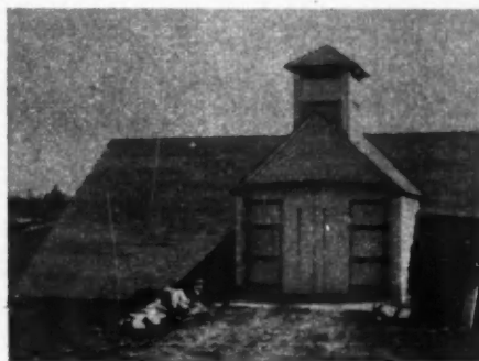
LOFT entrance for stacking potatoes at high levels. The cupola admits fresh air into the storage area for good ventilation
