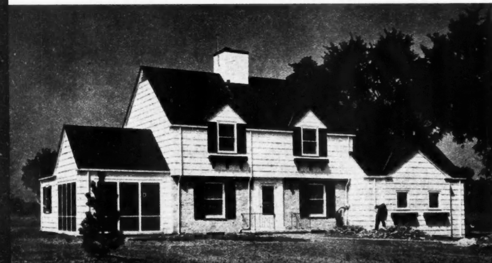
TYPICAL colonial exterior and plan with center entrance arrangement. Exterior walls are covered with wood shakes painted white and a veneer of stone on first floor front. Ample provision is made in this two-story and basement house for all activities. Emphasis is placed on the garden view by using large glass areas in rear windows
