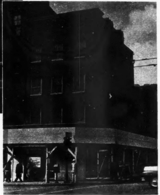
OLD building in its original condition
