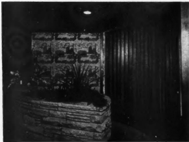
STONE plant bed and Mexican cedar louvers at basement stairhead
