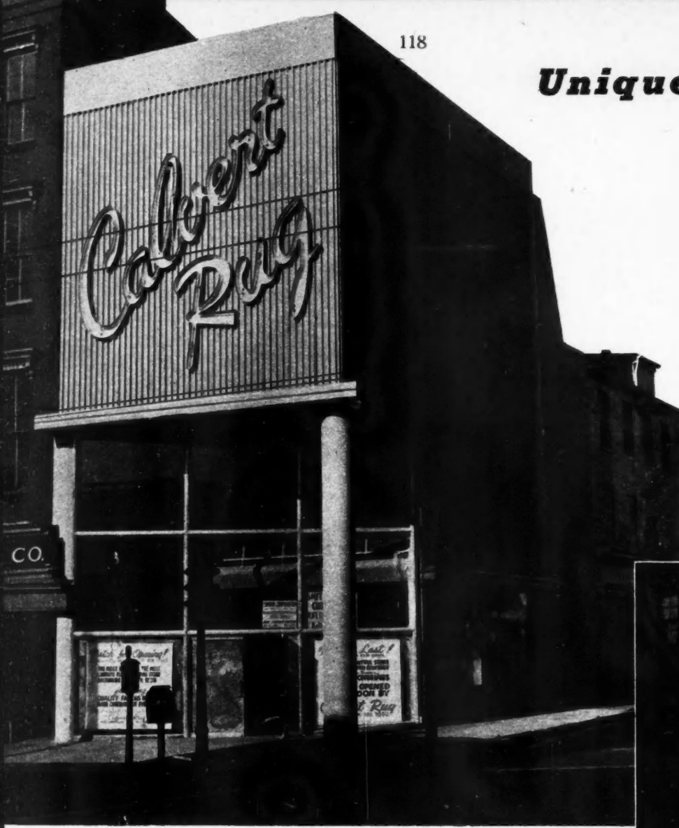
NEW portion of building shown with work in progress. Old part at right
