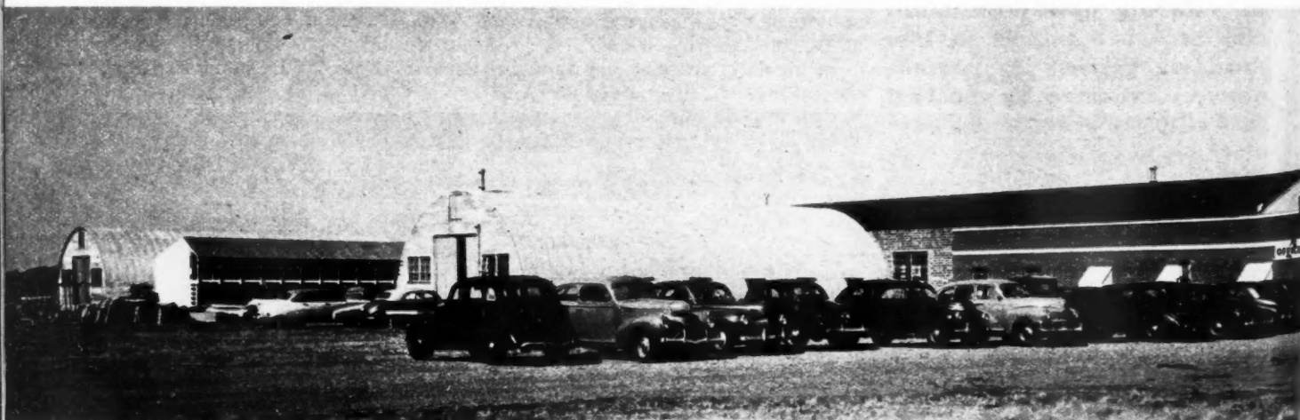
MODERN fabricating plant with building material warehouses and lumber sheds on eight-acre tract adjacent to Midwest City
