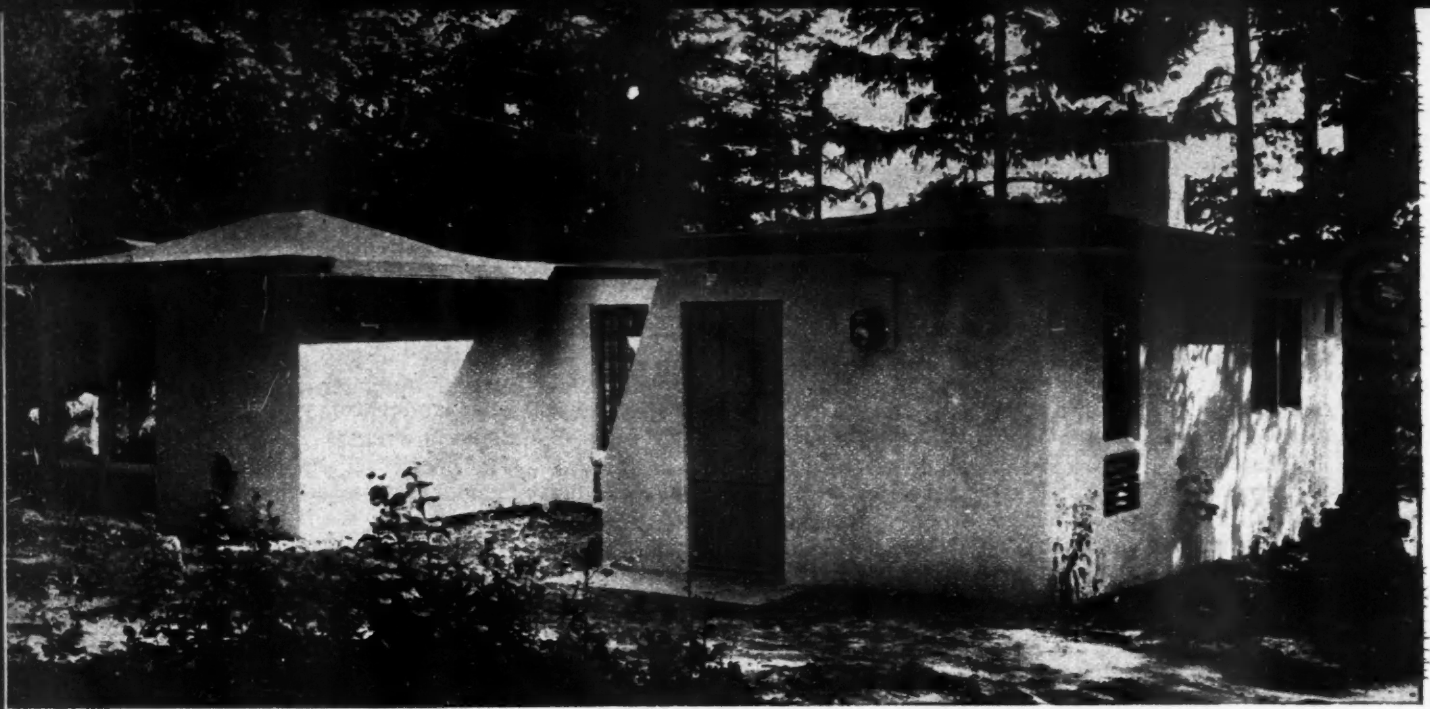
LIGHT-WEIGHT, insulating concrete forms roof, walls and floor of house, one of four pioneered, designed and built by Burt Smith
