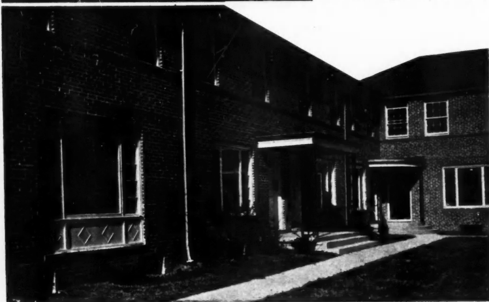
IN the process of completion, the 12-apartment house building is shown in detail view at left. This building is being constructed by the Broad-Waverly Corp., a subsidiary of the Creith Lumber Co. On the opposite page, is a complete view of the apartment building. The overall arrangement combines three basic units together to form one structure
