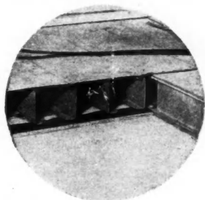
Here the panels form a plenum chamber for radiant heating
