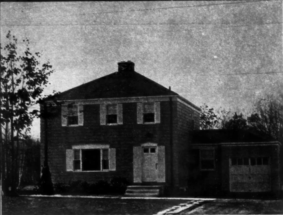
A HIP ROOF is used to vary exterior of the single floor plan used in Sutton Park
