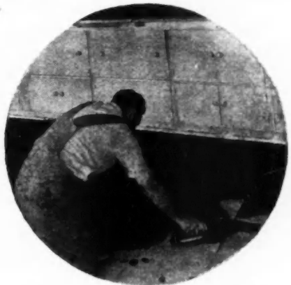
Spread the mastic and it's ready for linoleum
