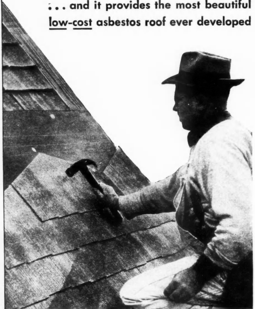
5. Easily Applied on Ridges —Special Hip and Ridge shingles supplied in exactly the same textured grain, the same beautiful, weathered appearance and colors as the main roof shingles.
