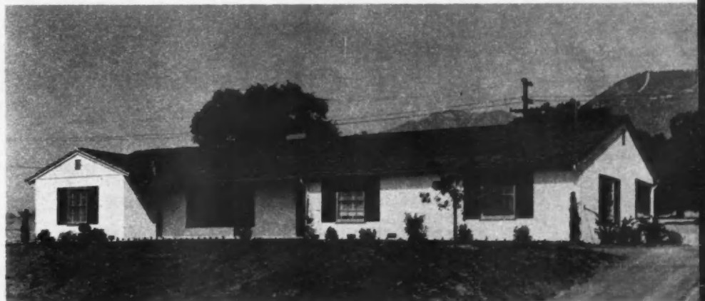
ANOTHER house typical of those turned out by the Bryan organization at minimum cost
