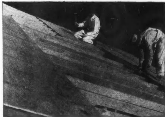
Panels of 3/8" Plyscord sheathed the roof, were covered with hand-split cedar shingles.
