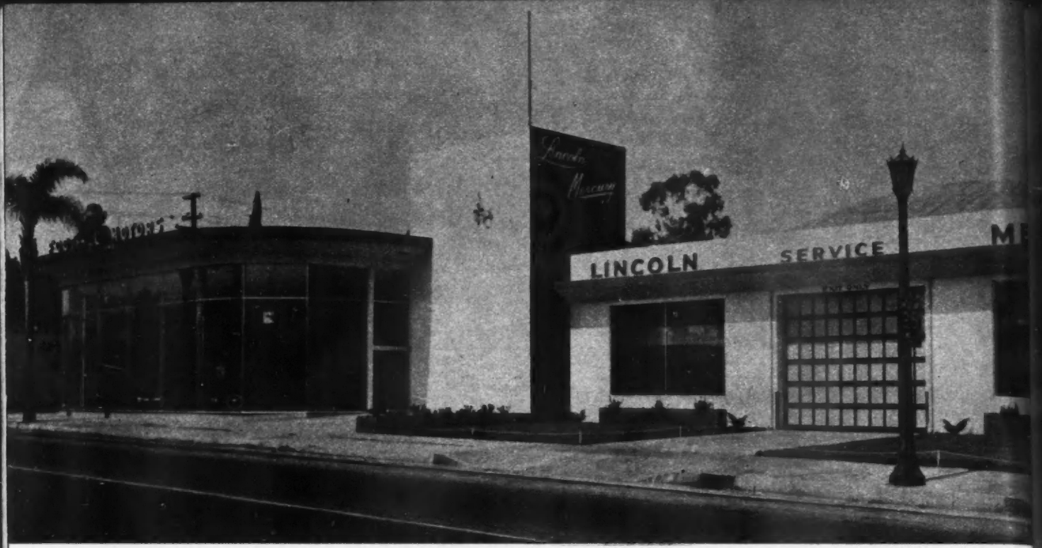
HUGE plate glass windows, 16 feet in height from floor to ceiling, surround the spacious automobile display room
