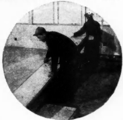
In fast—two men quickly lay the interlocking panels
