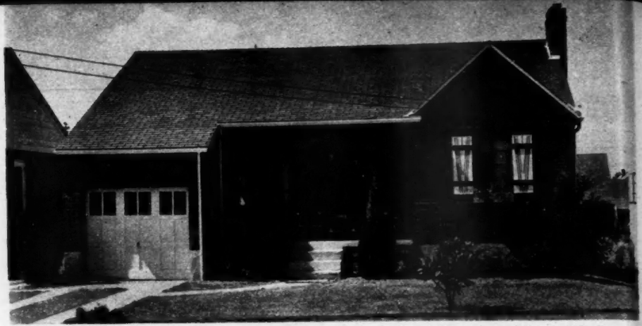
THIS small home was built in Cincinnati in 1941. Table below shows the builder's cost
