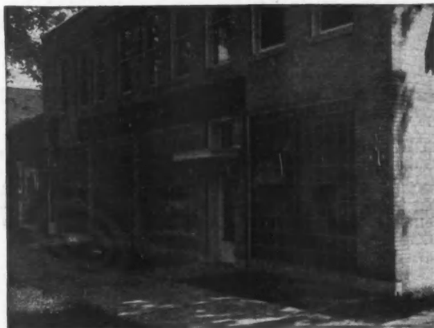
4. Wide panels of Insulux assure workers of much needed privacy, while ventilation is provided by small, clear-vision fenestration. Only occasional soap-and-water maintenance is necessary with Insulux.
