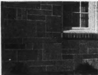
Dunstone (multiple-sized Dunbrik) creates new styling in masonry— note random ashlar wall above. Dunbrik is standard size brick with rare eye appeal.
