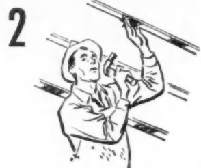
2 Nail Upson Fasteners to furring strips, 8" apart.
