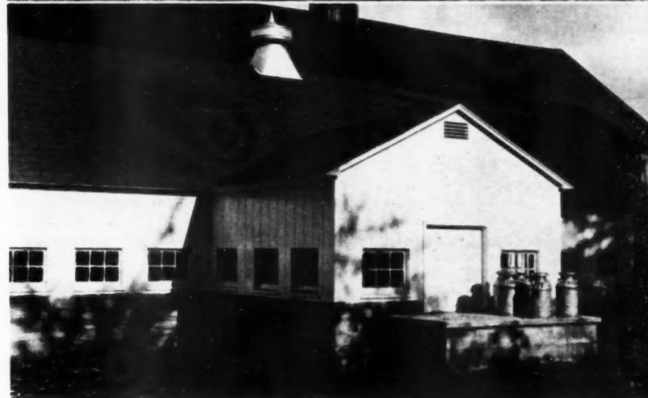
TOP picture shows how feed carrier is lowered to trailer. Above, is shown handy arrangement for loading platform at milk house. Note roof vent. Below left, is stairway to overhead feed storage. Stairs are on counter balance and recede into ceiling when not in use. Below center, shows close-up of roofed-over walk between milkroom, parlor, and shipping platform. Below right, is milk cooler, arranged close to loading platform
