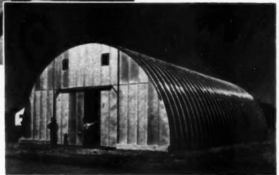
THE house at left was especially designed for the use of aluminum clapboard siding and aluminum roofing. The round-roofed building below illustrates one type of an all-aluminum general utility structure
