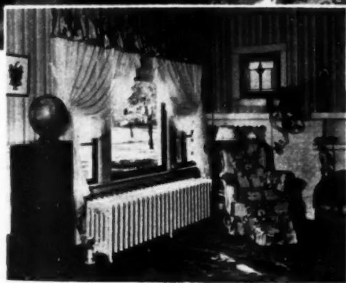
"BEFORE" and "after" photographs show replacement of a radiator with radiant baseboards
