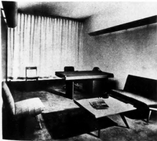
WALL on right is covered with a resin-impregnated Fiberglas mat cemented to plasterboard. Ceiling is fabric of glass yarns
