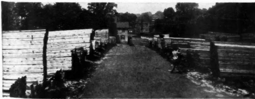
FULL stock piles of lumber are already evident in some localities
