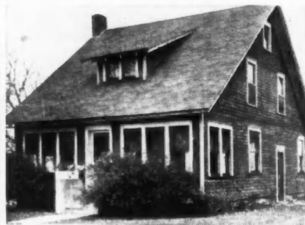
BEFORE aluminum roofing was added to home
