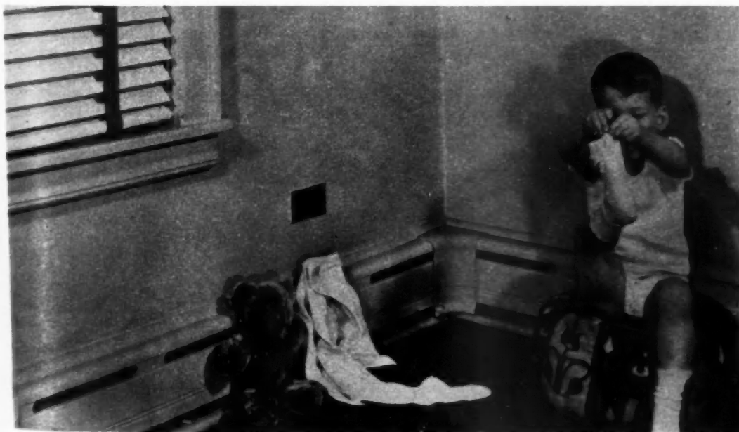
ANOTHER type radiant baseboard panel which might use either steam or hot water as the heating medium
