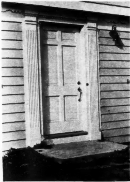
ENTRANCE detail of one of Chapdelaine's houses. Millwork for such entrances and exterior moulding is done in his own shop
