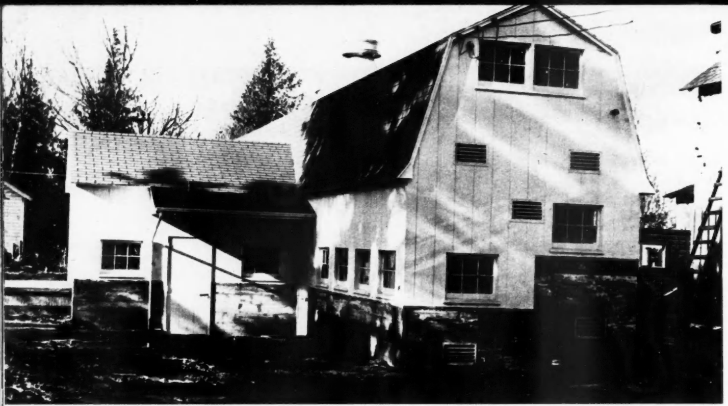
STANDLEY Graham's new compact milking parlor is designed to keep down material costs. End of the parlor is only twelve feet wide. Note the roofed-over walk for three entrances
