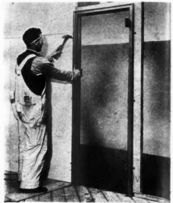
AETNA door frame assembled in one piece
