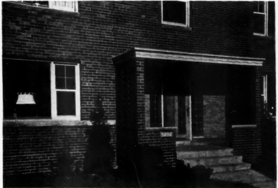
COMBINATION of patterned brick and glass block produces an effective entrance motif
