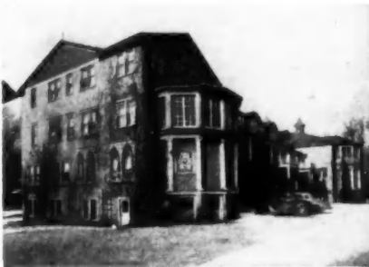
The Practical Bible Training School now heats and supplies hot water to dormitories, classrooms and apartments with nine G-E Oil Boiler units.
