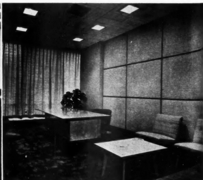
ON WALL at right, a black and white fabric of Fiberglas and cotton yarns is mounted over a glass fiber blanket on wood panels
