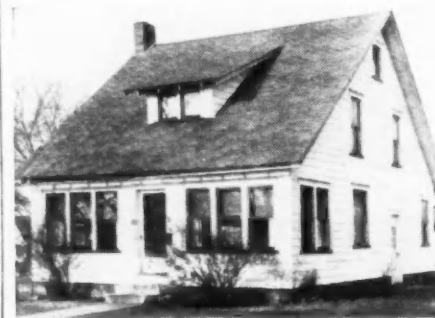
AFTER adding aluminum roofing made by National Aluminum Products Co., Canton, Ohio
