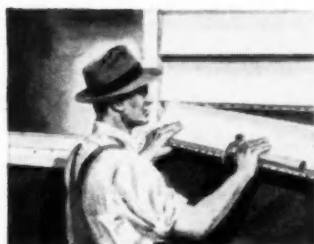
Applied from top to bottom, each section locks with a spring action, assures weather tightness, no rattles.
