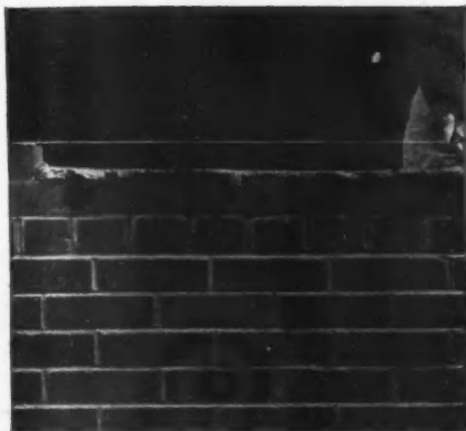
The mortar should be spread over a few brick only.
