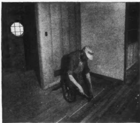
Subflooring—5/8" Plyscord. "No squeak or noticeable deflection," say the owners.
