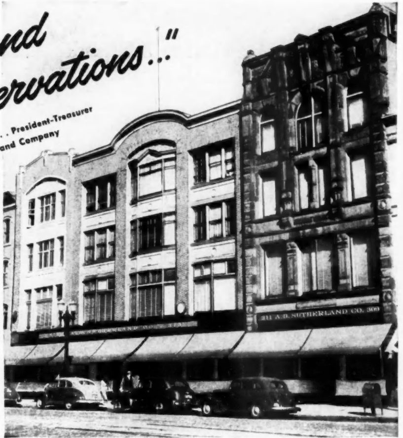
Both A. B. Sutherland Company's buildings are heated by the same G-E Multiple Installation. For greater economy the buildings were zoned into 3 heating sections.
