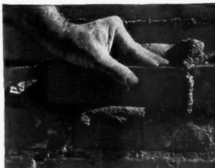
Then the brick should be shoved into this deep bed of mortar.
