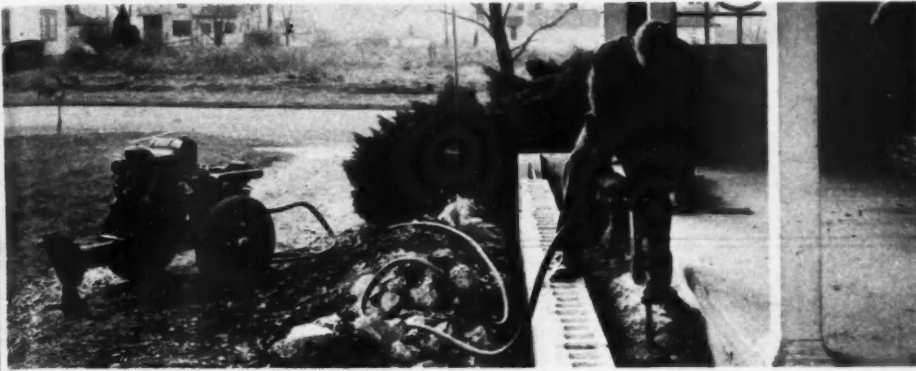
THIS light, easily portable Pac-Air compressor is big enough to operate a jackhammer, or paving breaker, digger, tamper or other air tools heavy enough to fill the small builder's needs. This is an especially valuable piece of equipment for use around remodeling jobs. Made by Ingersoll-Rand
