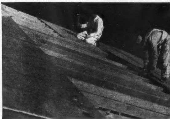
Panels of 3/8" Plyscord sheathed the roof, were covered with hand-split cedar shingles.
