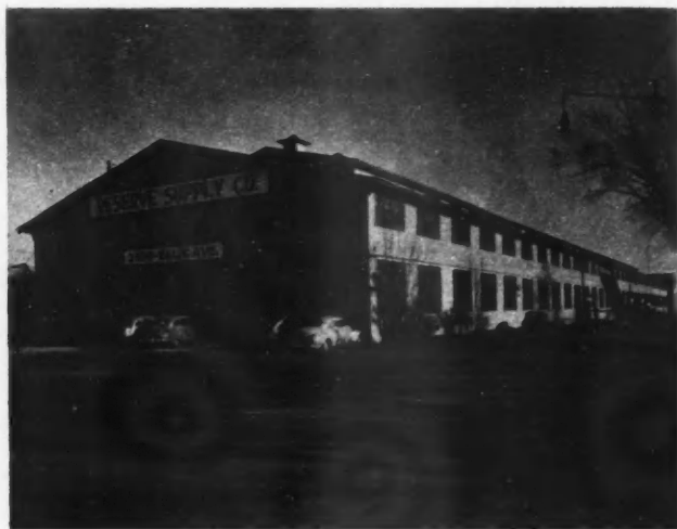
1. THIS 600-foot long warehouse accommodates the $10,000,000 annual business of Reserve Supply Co., St. Paul, Minn. In 1947 more than 1,600 boxcars of building materials were unloaded in addition to large shipments which arrived by motor truck. The firm serves 1,500 dealers in five states
