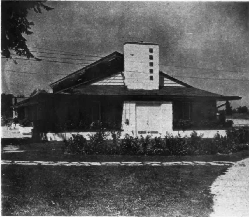
END view of the tourist cabins shows the clerestory windows above the roof line
