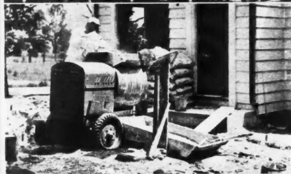
THE NEW Whitman Power Buggy is shown pouring foundations. It also hauls sands, bricks, dirt, and tools. It is easily maneuvered in and out of tight spots
