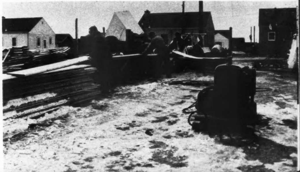
THIS compact Homelite dual voltage generator can be moved quickly from job to job, providing electric power for tools beyond the electric power lines
