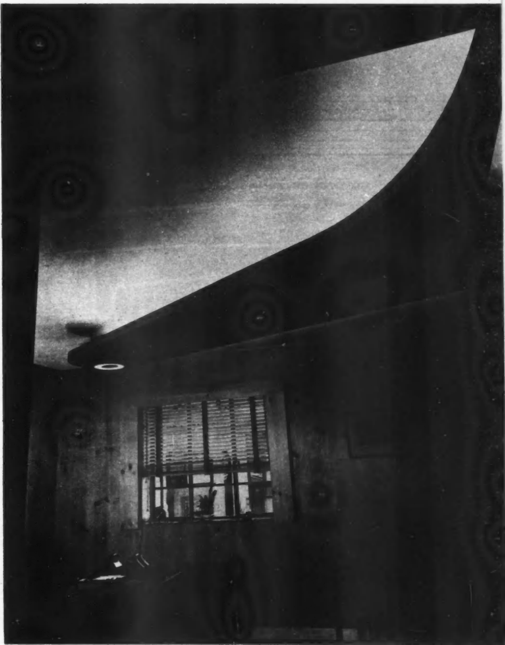
STORE or factory offices can be finished like this—knotty pine and Weldtex ceiling
