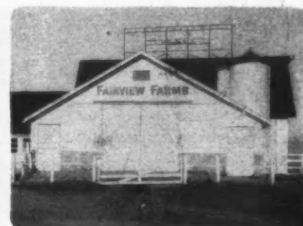
6. Stock barns, silos and other farm structures subject to high humidity.
