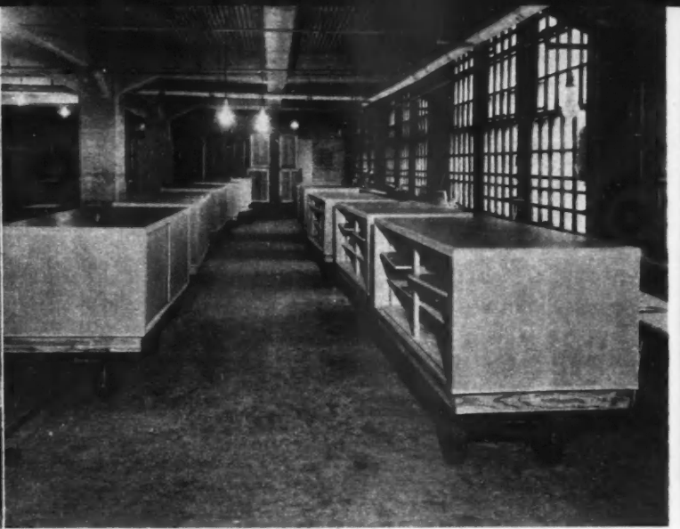
LEFT, rough frames for cabinets over which plywood will be applied. Right, semi-finished cabinets ready to install in store
