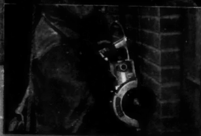
SKIL Saw is easy to handle on scaffolding or ladders. Note the operator is cutting out loose mortar before tuck pointing.
