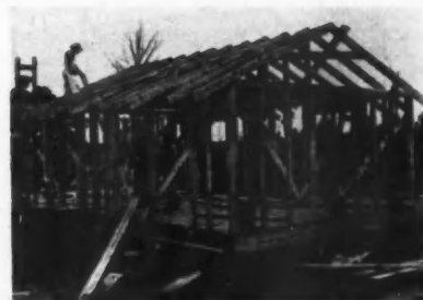
FRAMING erected in one work day
