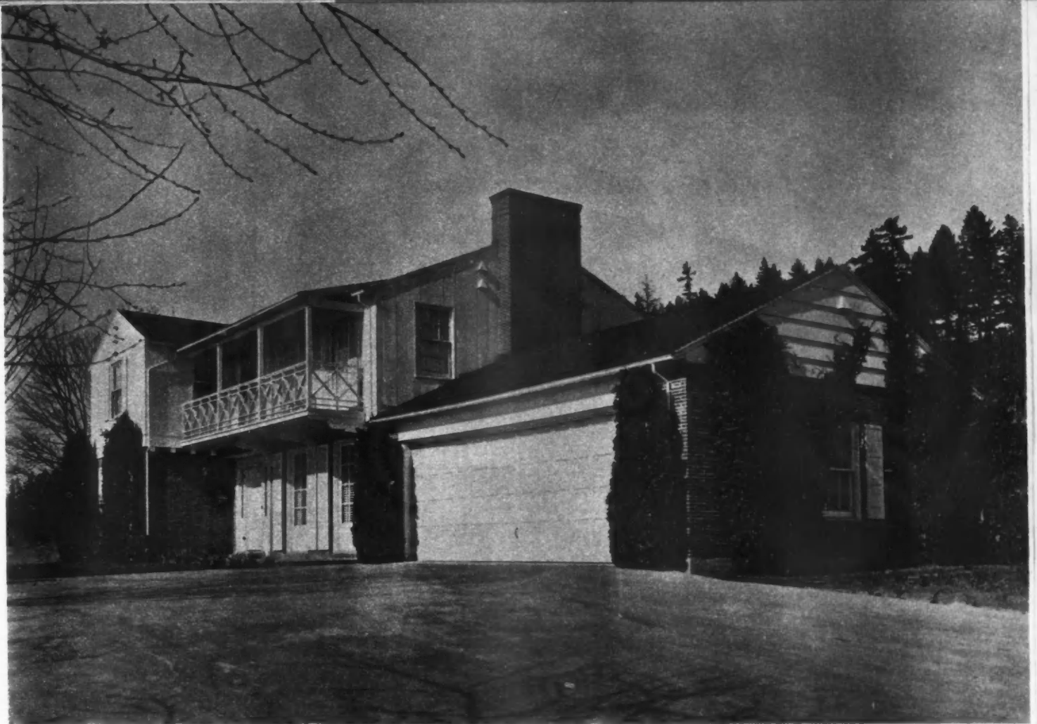
MONTEREY-style balcony of Blair home overlooks the Columbia river. Notice contrast of Roman brick and cedar siding
