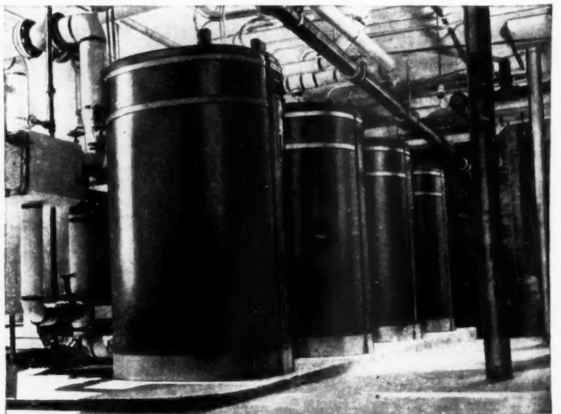
Compact G-E Oil-Fired Boilers save plenty of space. Their cleanliness, attractiveness permit use of basement for display rooms or additional working space.
