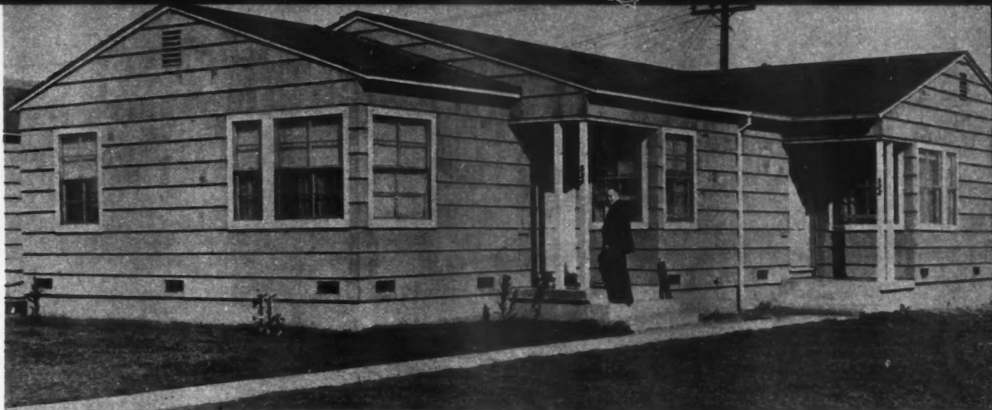
THE simple lines of the exterior clearly express the function and character of this duplex house
