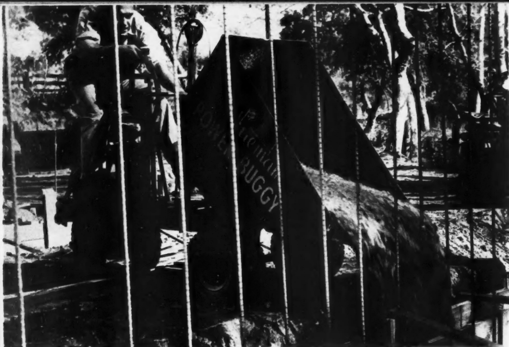
THE NEW Whitman Power Buggy is shown pouring foundations. It also hauls sands, bricks, dirt, and tools. It is easily maneuvered in and out of tight spots
