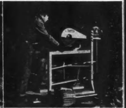
CLIPPER Mfg. Co.'s masonry saw cutting roof tile on a building job
