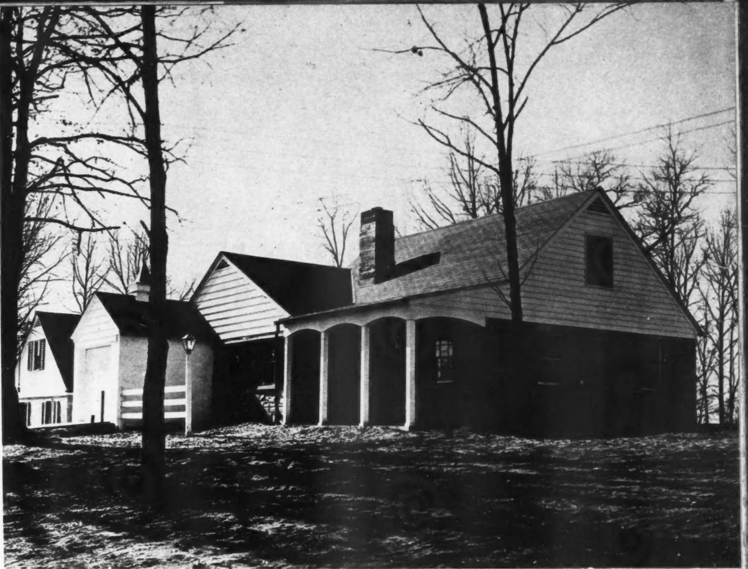
PHOTOGRAPH above and floor plan below of typical house in Indiana Limestone Co.'s housing development for employees. Note unplanned limestone veneer walls with stones of varying heights and colors to give pleasing appearance
