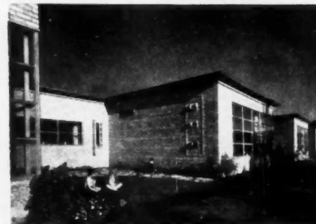
FOR FIRE SAFETY
