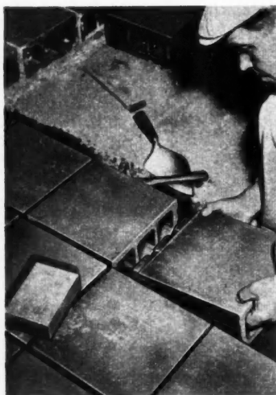
LEFT: Connection between perforated ducts and channels in floor blocks is made with open-bottom block as shown above. Right: By tilting block slightly, sleeves slip easily into preceding block. Ordinary mortar is used to bring blocks to exact alignment
