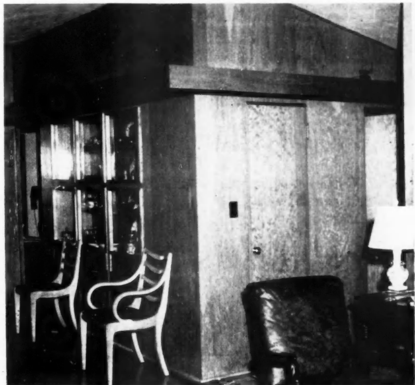
STORAGE walls are plywood. The clothes closet and china closet are framed with 2x2 members. Karlen and Steinmann rarely permit cross walls to be load-bearing
