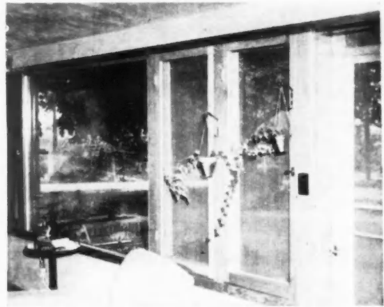
BOTH double glazed picture windows and casements were used in Malkow home. Trim over windows and door is plywood. Mullions were cut from 4x6 timbers
