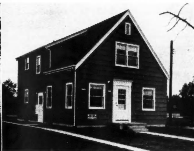
DUPLEX , built for NHW demonstration in Milwaukee by Alfred J. Weter, has the appearance of a single family home. It has two separate gas-fired furnaces. Front door serves the first floor occupants, while side entry serves the second floor. Each bedroom has an ample closet and there are two smaller closets in the hallway next to the bathroom. Second floor kitchen is directly above first floor kitchen and bathrooms are similarly placed to economize on plumbing and piping. Sold for $16,500
