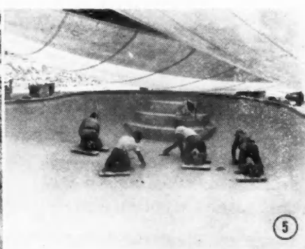
INITIAL digging of pool sites (1) is done with bulldozers whenever practicable. (2) Hand digging is needed to smooth final contours. (3) Steel mesh is set in place, ready for application of concrete. (4) Gunitite method of applying concrete. Man with hook pulls out steel in order that concrete may be distributed under it. (5) Silicite, manufactured by Paddock and consisting of silica sand and cement, is final plaster coat. Color is white, surface is smooth, and it gives the water a brilliant turquoise blue appearance
