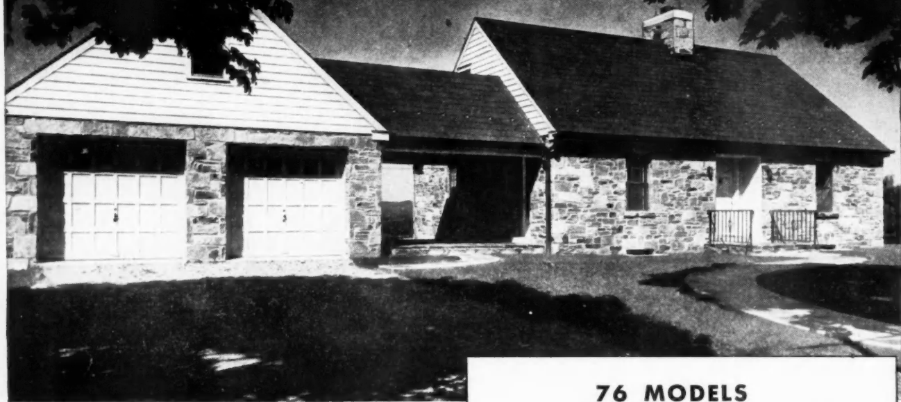
This lovely residence, the home of Mr. and Mrs. Forrest Beyer at Red Hill, Pennsylvania, is equipped with a dependable Spencer Heater. Architect: Charles M. Talley, Telford, Pennsylvania. Heating Contractor: Paul Schlicher, East Greenville, Pennsylvania.
