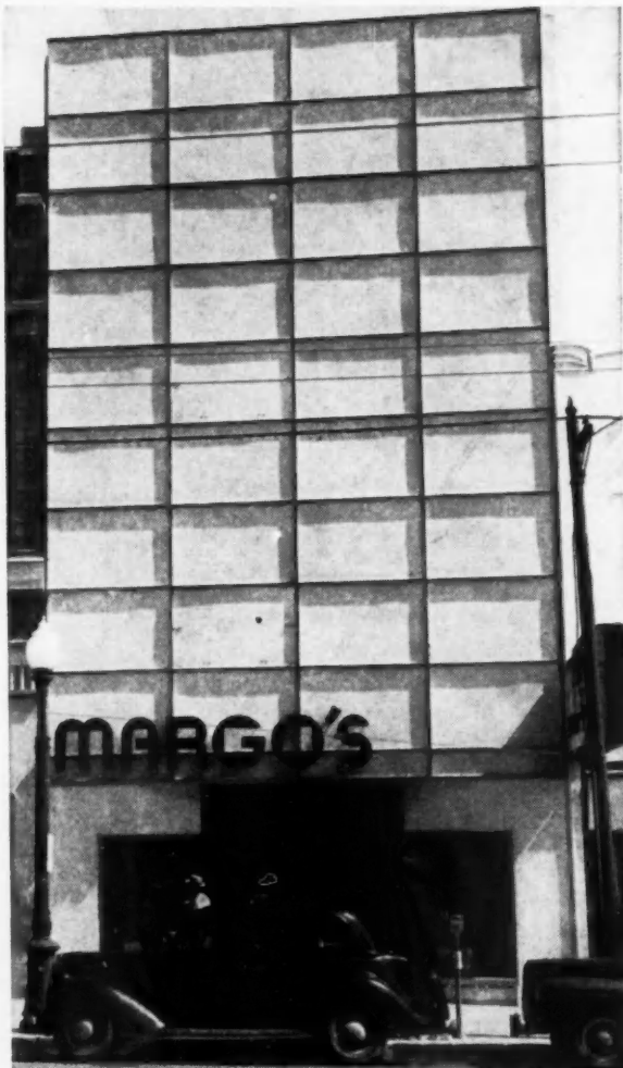
Attractive store front modernized with \frac{3}{8} " thick "Century" APAC. White & Prinz, Dallas, Texas, Architects.
