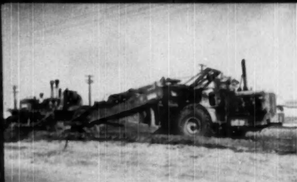
BIG Terra Cobra does original grading of site
