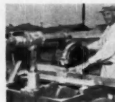
COMET table saw is used for cutting studs and headers
