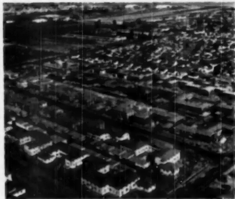
AIR VIEW of firm's 301-apartment project
