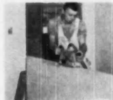
PORTER-CABLE sander takes care of finish work on door
