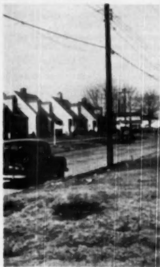
proceed during winter months when slabs could not be poured over frozen ground
