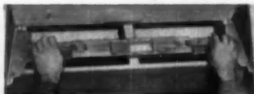
Measuring tread or riser
