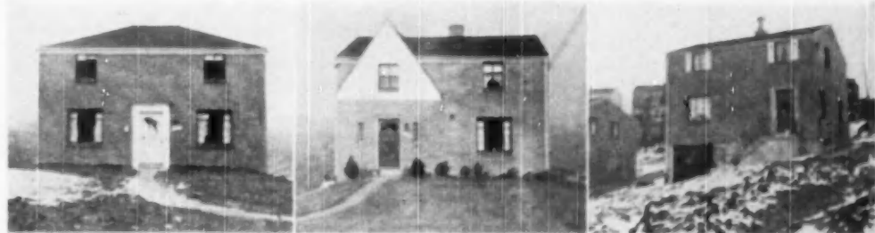
THREE houses spring from a basic plan which is similar except for position of the stairs. One stair is placed at centre, others at rear
