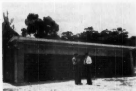
FOUR-VEHICLE garage built of rammed-earth at Australian experimental station. Side and back walls are rendered with bituminous emulsion to protect earth surface; front pillars are cement-faced; and roof is covered with bituminous sheeting
