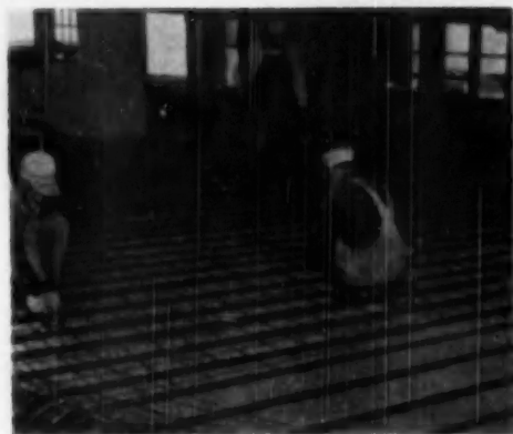
THESE radiant heating pipes rest on a vermiculite concrete slab. Workmen are placing reinforcing mesh for a concrete topping
