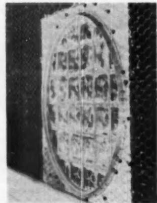
GLASS blocks form square, facing plywood
