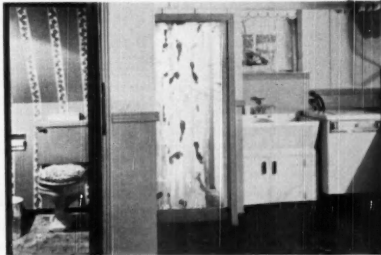
PLUMBING fixtures in basement add convenience for laundry, quarters or workshop
