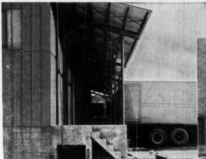
LOADING DOCK (LEFT) AND CAR PORT (BELOW) UTILIZING STRAN-STEEL AVAILABLE FRAMING.
