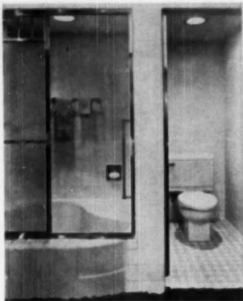
THE UTILITY of this bathroom arrangement is increased by the use of vapor-proof incandescent ceiling lights in compartments
