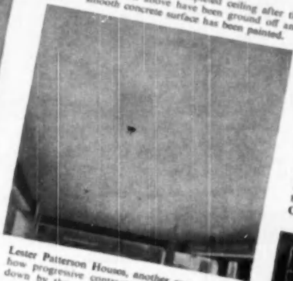
(1) Close-up of a ceiling after the GPX Concrete Forms have been removed.
