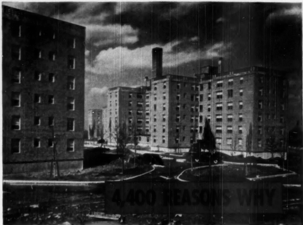
Todt Hill Apartments. 4,400 windows of Alcoa Aluminum manufactured by Starling Windows, Inc. Owners: New York City Housing Authority. Architect: H. L. Feldman. General Contractor: William A. Barboux, Jr.
