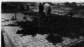
Here SISALKRAFT is shown laid over subfill, with concrete mix being spread over SISALKRAFT and reinforcing rods.
