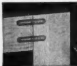
Dowels are used at all important joints.
