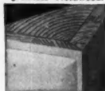
Heavy corner blocks reinforce base cabinets.
