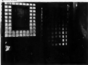
Completed job is light and attractive
