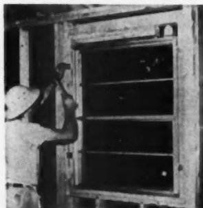
THIS builder's efforts to cut down on the number of parts to be handled in assembling a house resulted in his choice of a factory-assembled window unit complete with screen and storm sash, which can be easily and quickly installed in one operation on the job
