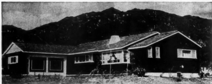
FRONT AND SIDE VIEW of house showing the forecourt created by the L-shaped plan. An interesting feature is the use of bay windows in the kitchen, front bedroom
