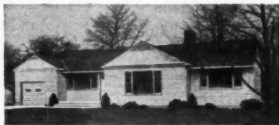
The LFI Method of Construction was used to build the Ranch Home pictured above, from the Akron Builder's own plans
