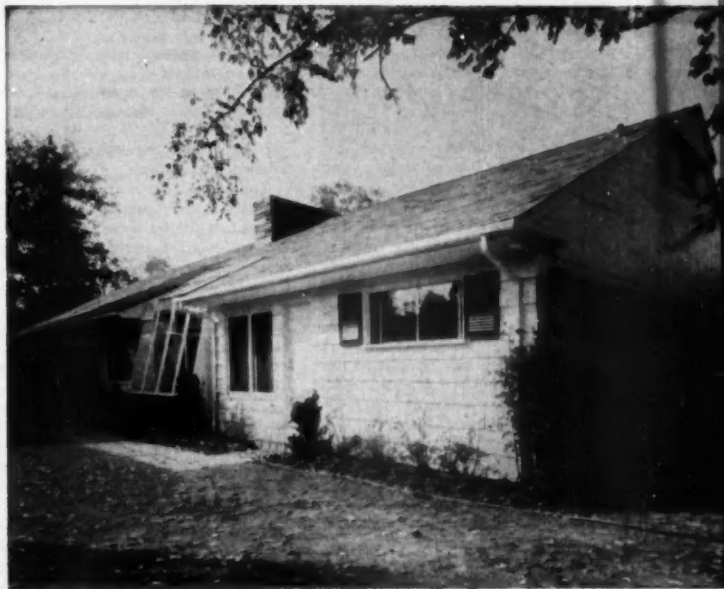
SOUTH side of the house, which is the rear, showing some of the large glass areas located here to take maximum advantage of sun in winter and a garden view in summer
