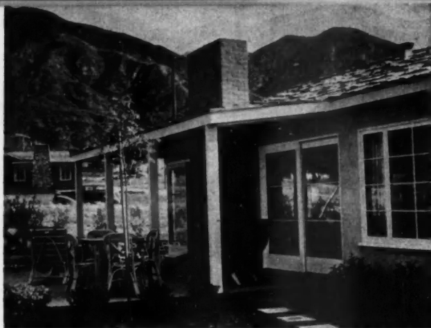
PARTIAL VIEW of rear of house showing covered porch adjoining living room
