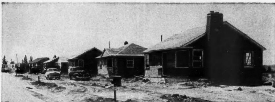
RESIDENTIAL STREET takes shape as Spokane homes replace open terrain. Builders had only to build; mortgage firm did the rest
