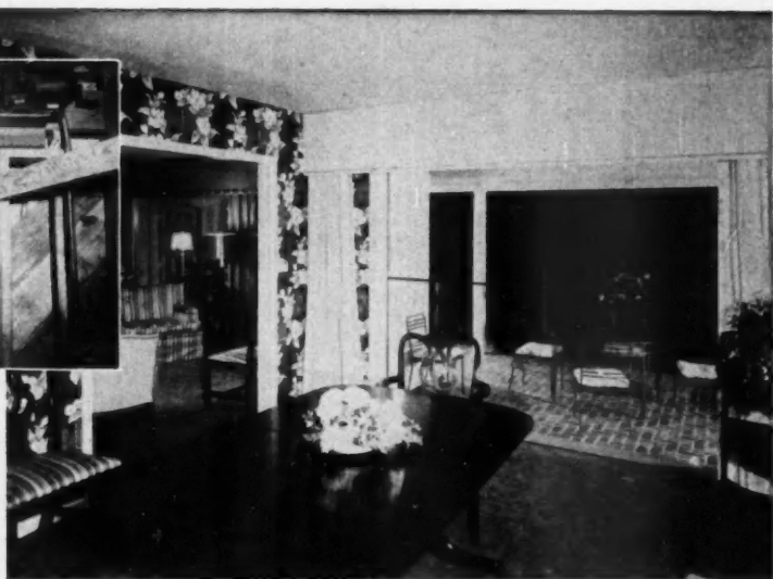
LOOKING toward the terrace from the dining room with the double-glazed plate glass wall section, which is raised or lowered by clicking an electric switch, shown lowered part of the way. This large glass unit is suspended on steel straps. Inset shows motor and mechanism as it appeared installed
