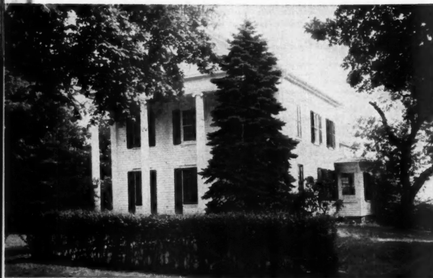
THE HOUSE AFTER modernisation retains much of its original form, with emphasis placed on removal of so-called ornamental "ginger-bread." Well proportioned columns and cornices with the addition of blinds for windows have removed every vestige of its former appearance and have turned a liability into an asset
