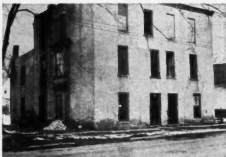
OLD STRUCTURE as it appeared when Sonnenberg started his remodeling operation. Stone walls are 20 inches in thickness
