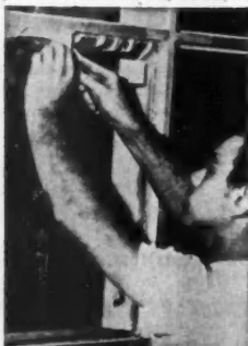
VOIDS filled when glass is set
