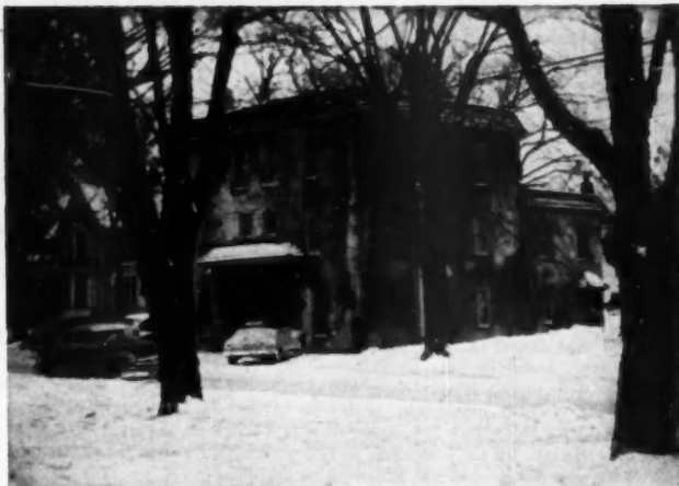
COMPLETED structure with covered entrance and tile coping to make it appear lower
