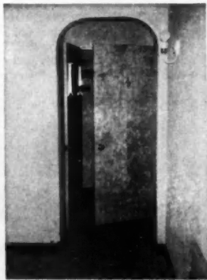
FLUSH panel doors were finished naturally and open doorways were arched
