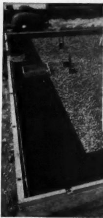
Cold transfer and heat loss are minimized when a border of PC Foamglas—as shown here—is used under a floor slab. In many modern homes, walls, roofs and floors have been successfully insulated with PC Foamglas. Photos Courtesy of National Homes Corporation, Lafayette, Ind.
