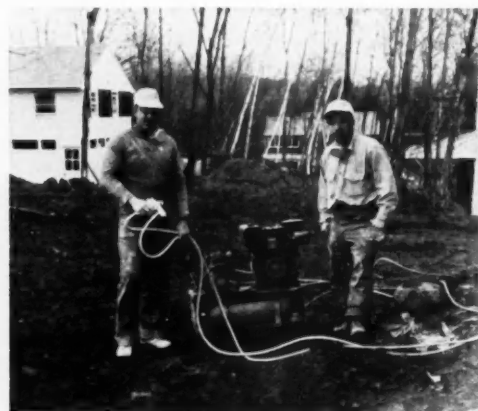
SPRAY GUN AND COMPRESSOR applies prime coat of paint
