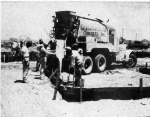
TRENCHER (left) digs a foundation in 15 minutes. Tractor spreads dirt. Concrete mix truck (right) pours foundation
