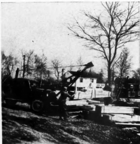
HOIST on Dodge power wagon picks up banded lumber
