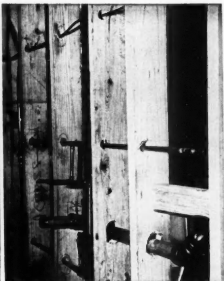
▲ PLUMBING fits perfectly in holes bored in studs by use of patterns and power equipment before erection
