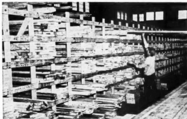
PIECES cut to length, marked and bored, are stored in these bins for delivery to job in complete sets. When construction crew is ready for base plates, a set of these is delivered to job. Raiser and top plates next in order of use are then delivered
