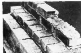
POORLY filled mortar joints make leaky walls
