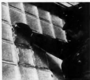
GOLD STRIPE on top mortar-bearing edge of Insulux block guides correct placement
