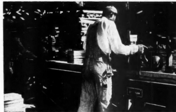
JOISTS and rafters, on Keesler job, are precut at a portable mill on the site, which is moved as construction progresses. Precutting of parts is also done in the mill
