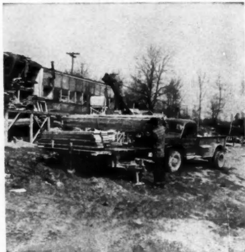
POWER WAGON HOIST loading trailer for delivery to site
