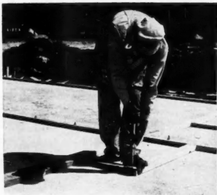
BASE plates are laid out on concrete slab and fastened with bolts and nails using a Drive-It. No sawing has to be done as all pieces have been cut to length. Installation time: 45 min.
