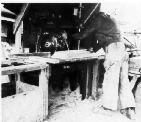
16-INCH DEWALT POWER SAW will cut eight studs at one time
