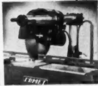
THE TIMBER CUTTER Up to 10 h.p., cuts 16" by 16" timbers.
