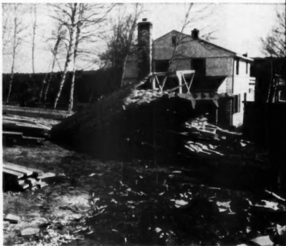
LUMBER IS DROPPED from till-top trailer pulled by power wagon
