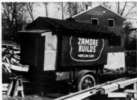
MOVABLE CARPENTER SHANTY. This unit carries a generator, electric hand saw, nails, and tools for a six man crew
