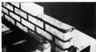
HOW MORTAR is properly spread, uniformly
