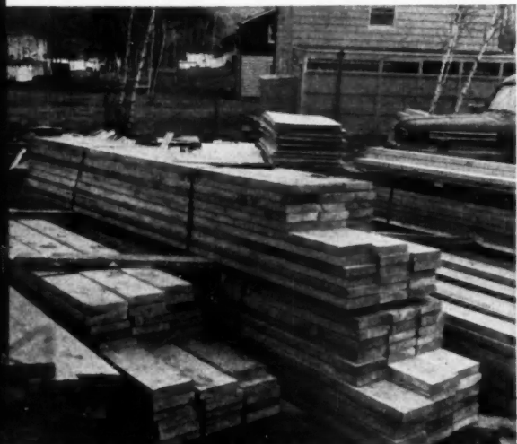
FRAMING LUMBER BANDED ready for delivery to house site
