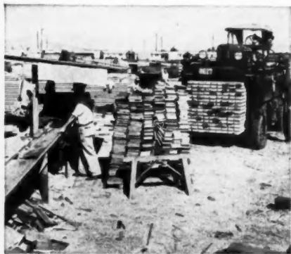
CARRIER moves lumber from cutting shed to individual building sites in project
