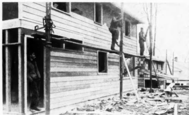
METAL PUMP BRACKETS for scaffolds, operated on vertical wood posts for wall surfaces
