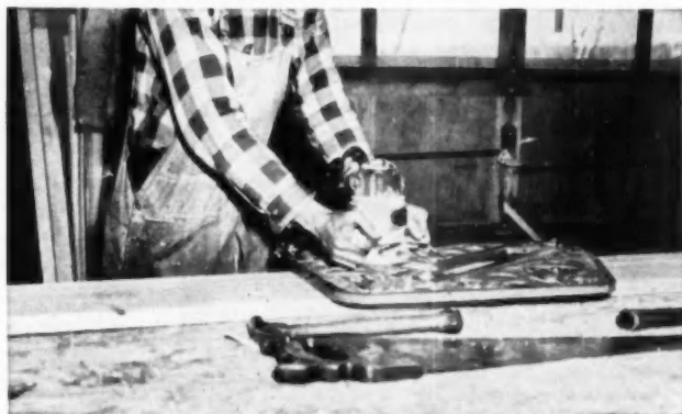
ELECTRIC ROUTER working on a template for stair stringer
