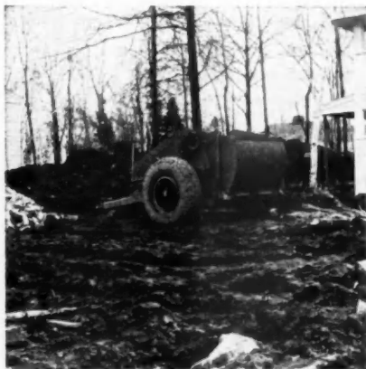
THREE YARD CARRYALL used for site leveling
