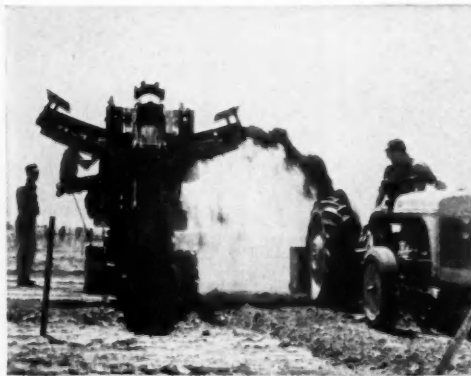
TRENCHER (left) digs a foundation in 15 minutes. Tractor spreads dirt. Concrete mix truck (right) pours foundation
