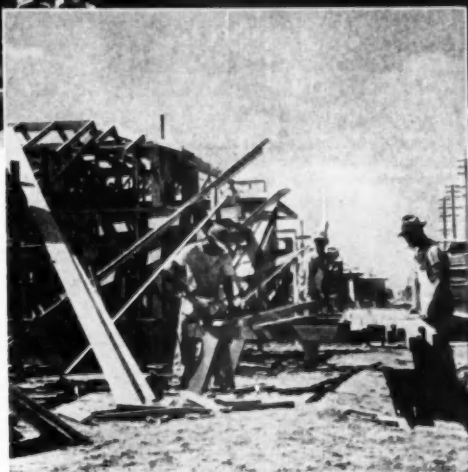
HAND SAW is used to notch and cut rafters at site
