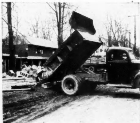
FORD DUMP TRUCK unloading concrete block at building site
