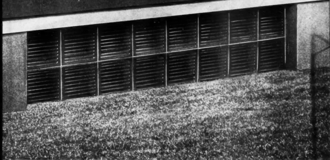
Installed in place of sash, Insulux Glass Block hides outside views and makes a sound, weather-tight, insulating wall.
