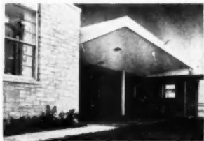
COVERED PLAY area has insulated canopy
