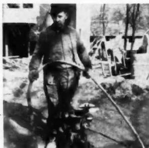
CONCRETE VIBRATOR used around the load-bearing edges of the floor slabs
