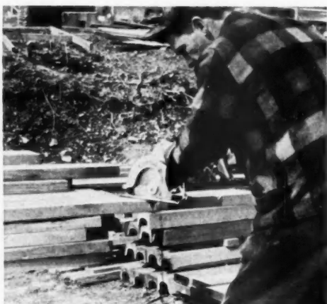
SKILSAW making bevel cut. Handy power equipment used on site
