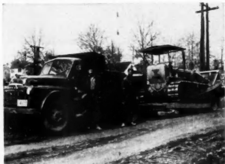
CATERPILLAR D-8 mounted on a two wheel trailer being towed by Dodge dump truck to site of a new 192-house Zamore project
