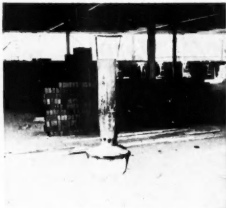
SALAMANDER used in partially opened building, will protect clay products when temperature is between 32 and 25 degrees F.
