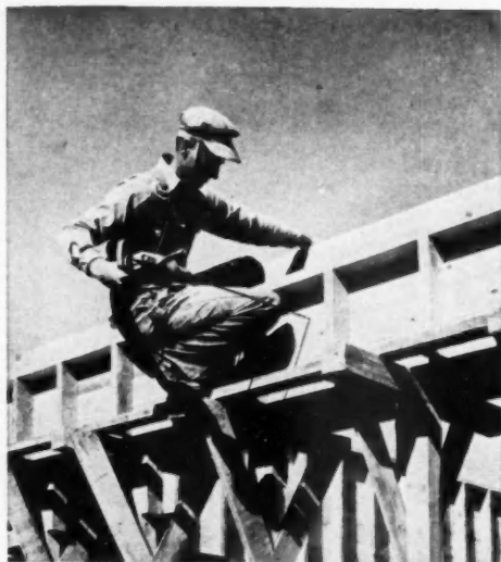
POWER DRILL with long bit speeds tying on of concrete forms
