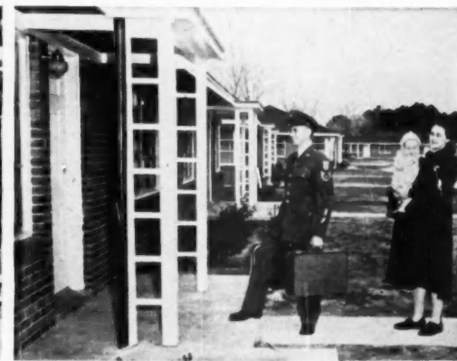
SERGEANT and Mrs. Edward K. Lynch and their son move into one of Keesler units of Wherry Housing Program. New pre-cutting system and use of power tools give them extra comforts
