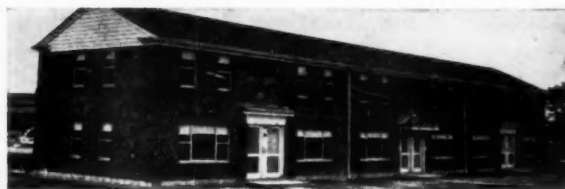
FT. CAMPBELL, KENTUCKY. Wherry Housing Project, Southern Apartments, utilized thousands of Rusco Prime Windows.
