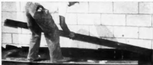
5 To complete the insulation of the floor perimeter place the same type of rigid, waterproofed insulation board 4-in. wide and 1-in. thick on edge against outside wall on wide insulation board (see diagram at top).
