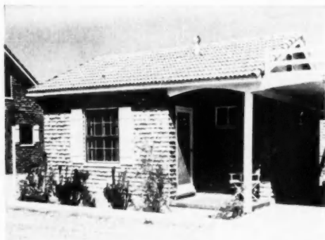
AS FURTHER PROTECTION against noise, the units are built of 4x12x8 inch concrete blocks, set with "weeping" joints
