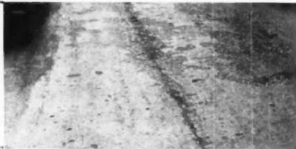
Correct air entrainment prevents the kind of deterioration shown on this pavement slab. Always be sure your mix will produce the air-entrained concrete the job requires.
