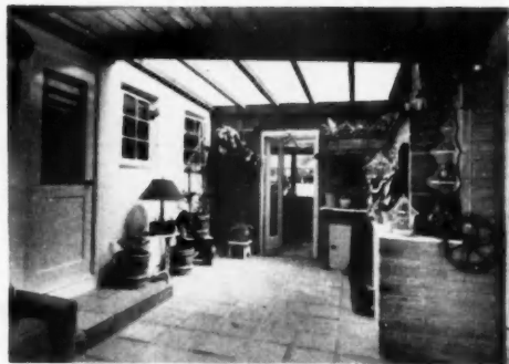
THE STRENGTH and light-transmitting qualities of translucent plastic laminate have been used to improve the patio
