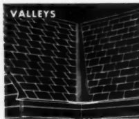
Terne Metal valley applied to asphalt shingle roof.
