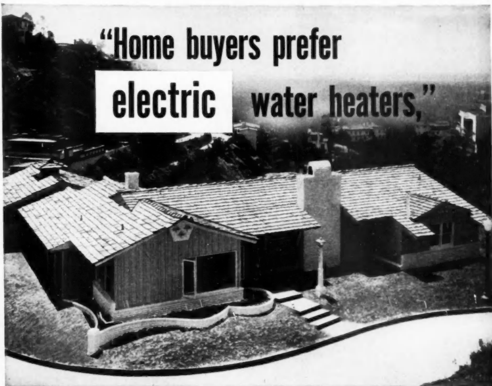
Mr. May's latest home in the Hollywood foothills is farmhouse style. The Electric Water Heater is located next to the automatic clothes washer in the utility room, which allows short hot water lines.
