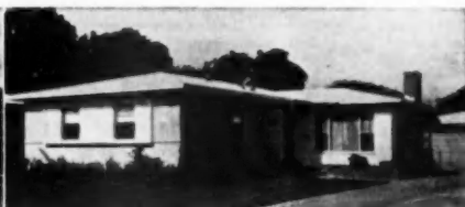
SANTA ANA, CALIFORNIA. Rusco used on all Barkley Square and Sunshine Homes by builder Burt Huff.
