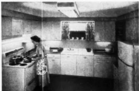
Kitchen Light Conditioning recipes call for under-cabinet and over-sink lighting, shown above, to reduce shadows, make work easier.
