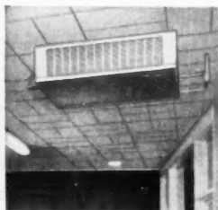
Type C with optional inlet grille for ceiling use—(heating only). Duct connectors also available.
