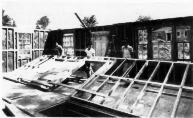
UP GOES A GROUP of wall panels assembled at plant to form a main partition
