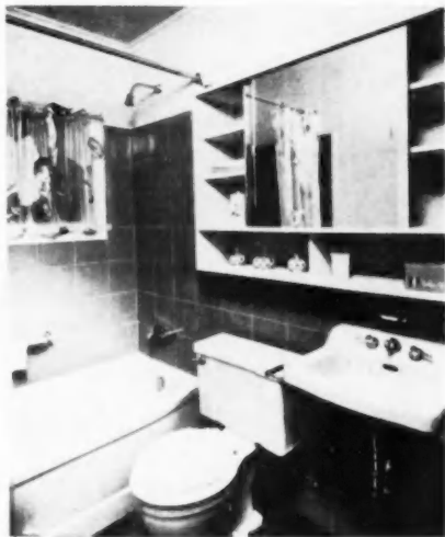
BATHROOM DETAIL includes a 2x4-foot shelf closet mostly enclosed by two 2x2-foot mirrored sliding panels. A 4-foot fluorescent fixture is overhead.
