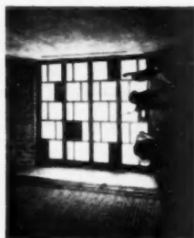
TRANSLUCENT plastic sheeting provides ample, well-diffused light admittance, but is not transparent. Here it is shown used in door panels
