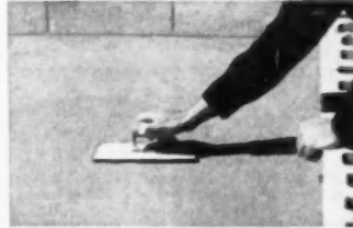
8 Finishing with steel trowel will produce smooth surface. Avoid excessive troweling. Moist cure floor at least two days. If finished floor is to be exposed moist cure at least five days.
