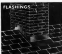
Terne stop flashing applied to chimney on slate roof.
