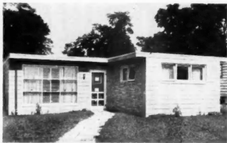
MODERN HOME is nearly all concrete: blocks for exterior were cast to resemble siding; floors and roof are concrete slabs; partitions are 4-inch concrete blocks
