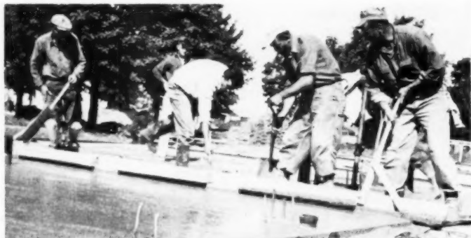
Screed levels off half of slab. Copper pipes seen in the slab are hot water heating pipes for baseboard heat. Pipes are one piece copper tubing. ends are closed to keep concrete out of them
