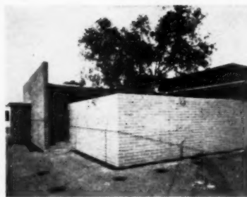
Texture and color tone of walls were improved by sandblast treatment
