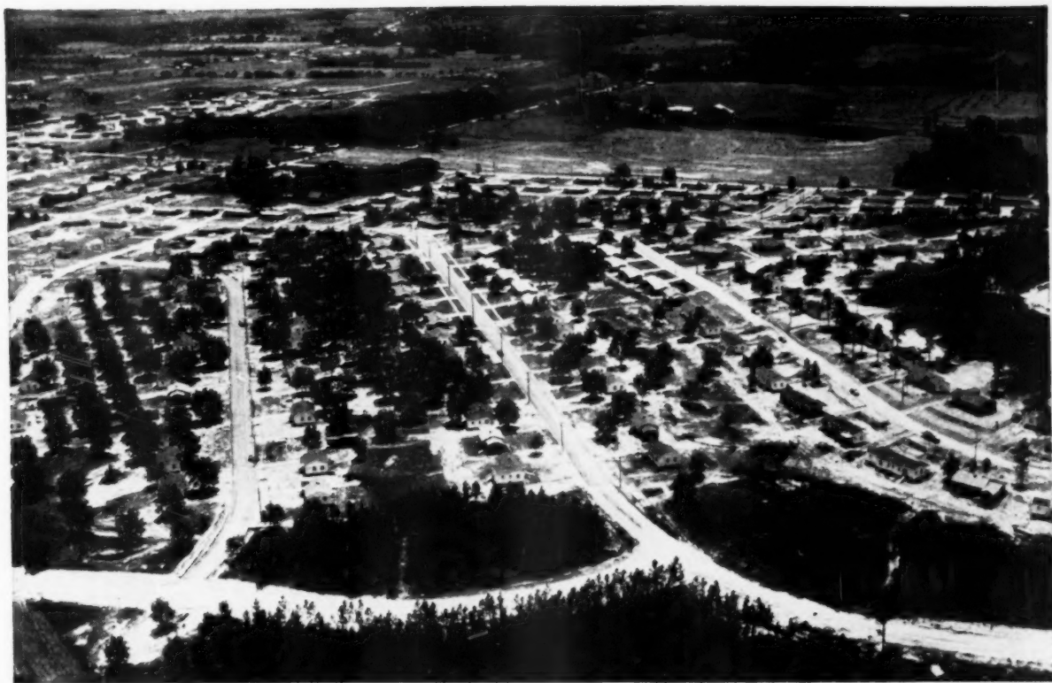
About 200 more Knox Homes have been added to this attractive Fleming Heights subdivision in Augusta, Ga., in the past year. All are roofed with Certain-teed Thick Butt Asphalt Shingles.
