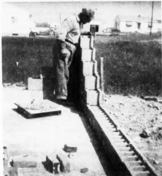
On the job demonstration of mortarless block
