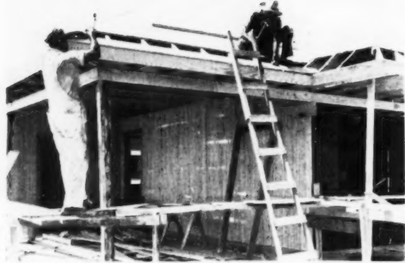
Roof sheathing is 1x8-inch pine boards. Barrett shingles are used, in three pastel shades, one black, one red blend, one slate and one white. Every house has a built-in ventilating fan installed in the attic, with exhaust vents in eave soffits
