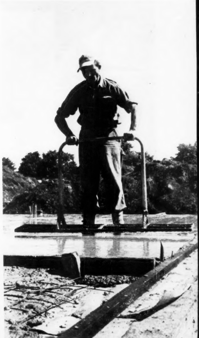
"Jitterbug" used to agitate concrete for float finish
