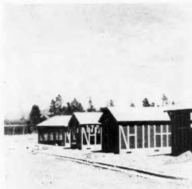
The Lake Hotel cabins in various stages of completion. Note how the exterior plan of exposed studding and cross-supports
