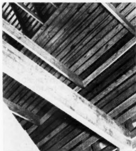
1x6 sheathing spaced 1 1/2 inches nailed to the rafter assures ventilation above the plate where corn would normally lay against the roof board. Air can circulate between the rafters
