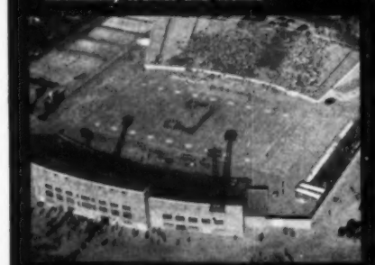
CHARLESTON, S. C.—Johnson Hagood Stadium Architects, Salsen and Cummings
