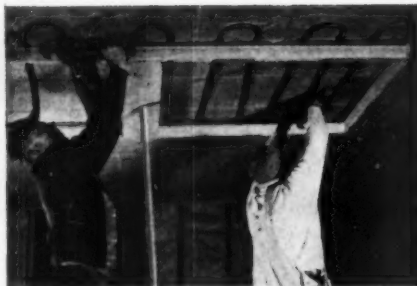
Lightweight PG's are easily installed. Trim, straight grids fasten tightly to ceiling — permitting a minimum, even thickness of plaster.
