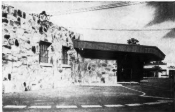
South elevation provides three drive-in windows (one not shown). Redwood fascia boards, 1x10-inch, with 1x2-inch redwood battens, are used as a design motif
