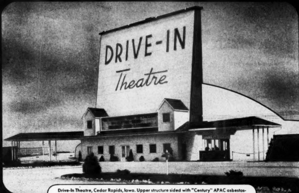
Drive-In Theatre, Cedar Rapids, Iowa. Upper structure sided with "Century" APAC asbestos-cement sheets, 1/4" thick. Theatre owned by Tri-States Theatre Corp., Des Moines, Iowa.
