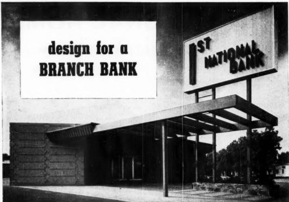
Native stone, lightweight concrete slabs, redwood and aluminum are combined to produce an inviting entrance. Sign is 16-gauge aluminum, over nine feet high
