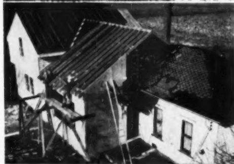
Major step in remodeling, extended living room wall so it runs flush with bedroom wing, raised roof to create better proportion with rest of building
