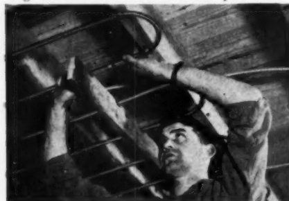
All PG's are furnished with one end of the tube expanded. After cleaning and fluxing, PG's are connected by soldering or brazing. Many fittings are eliminated.
