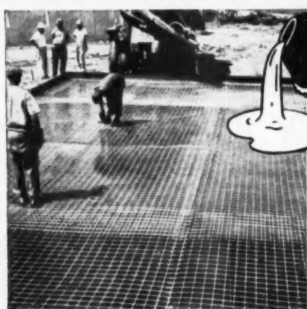
THIS PICTURE SHOWS how American Welded Wire Fabric knits the floor of an entire home into one solid concrete slab. It distributes the strength of steel evenly throughout the slab, controls cracking, prevents heaving and spalling. Floor slabs like this insure long-lasting living comfort and rock bottom economy for home owners.
