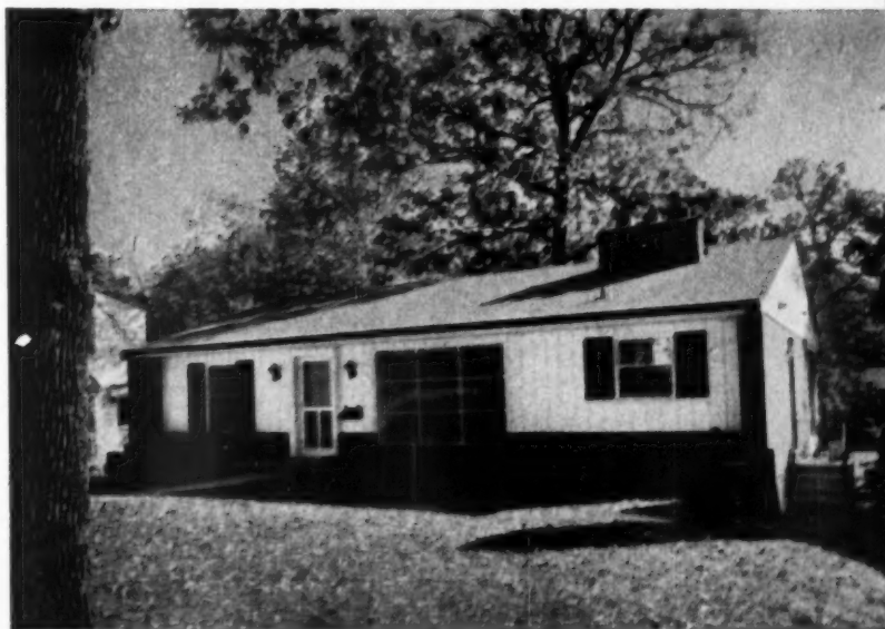
Front of the house presents a one-story view to the street. End walls of brick are extended to receive roof overhang
