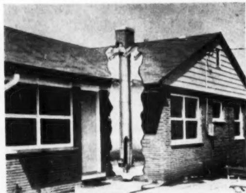
SECTIONAL CONSTRUCTION (shown above in cut-away) saves 30% to 50% on time and material over brick chimney cost. The Van-Packer may be placed directly over furnace in center of house as easily and inexpensively as against a wall.
