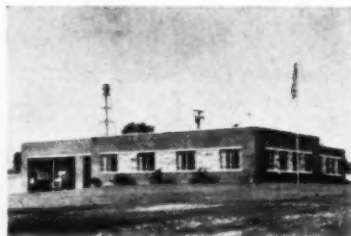
Superior Township Hall, Washtenaw County, Michigan
