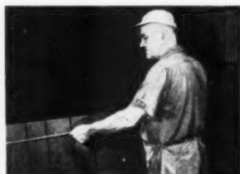
Chalk line establishes level for a course of shingles
