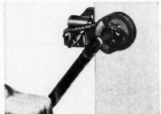
After inserting bit, attach handle and turn to bore hole.
