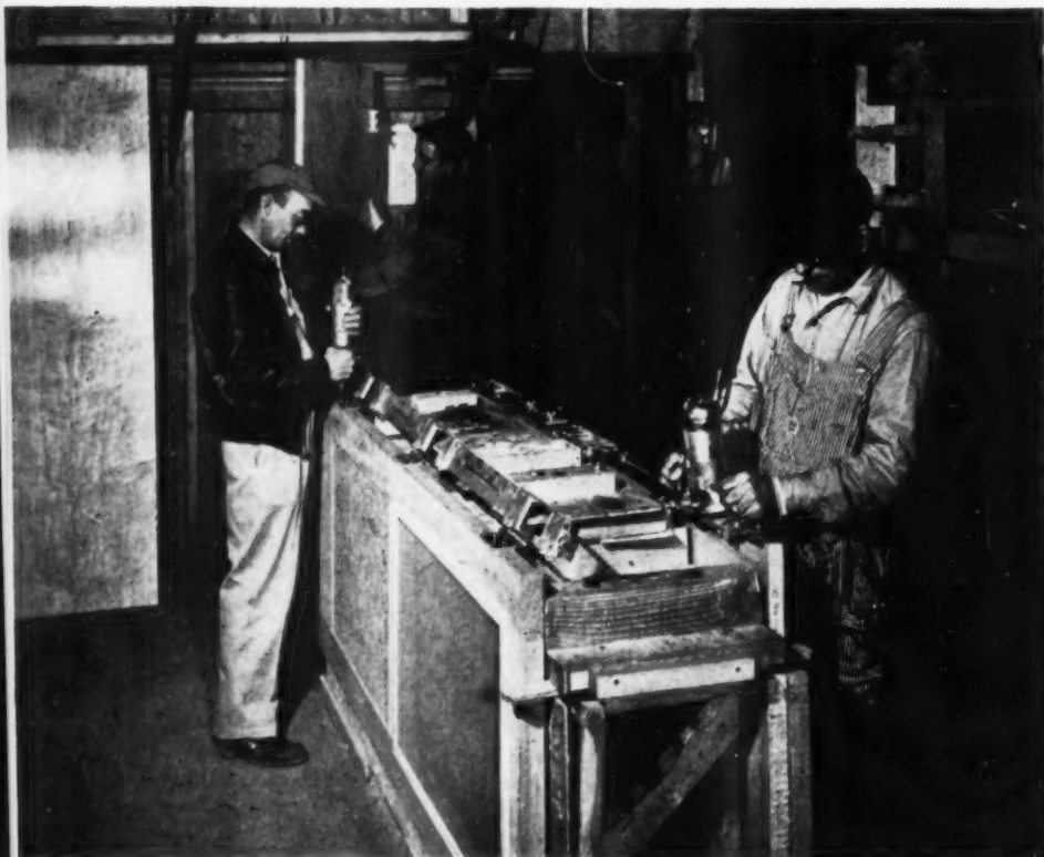
Butt template table: Carpenter on right is using electric butt router, cutting holes for hinges on doors. Carpenter on left is installing hinges with electric screw driver. Each process can be done alternately. Thus, each man works his way around table
