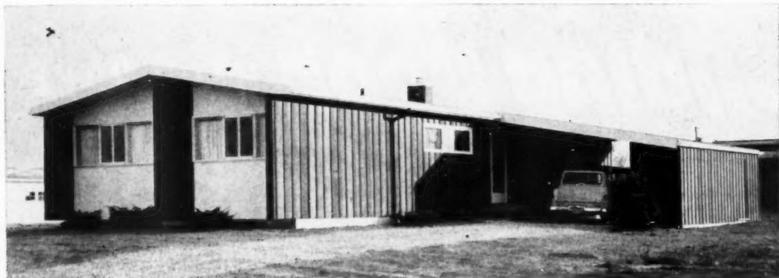
Redwood boards and battens, coated with natural redwood stain, combined with sections of exterior Weldtex paneling painted white
