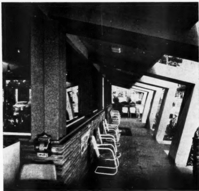
View inside of the terrace with protecting canopy formed by the roof overhang
