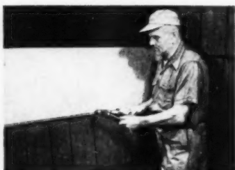
Clip and sheathing are nailed together at each stud
