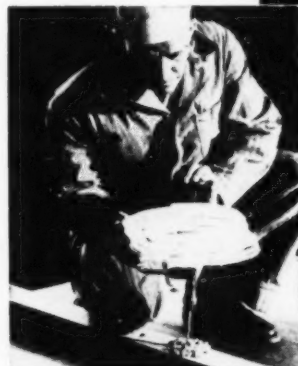
BRACE AND AUGER take 36 seconds to drill 7/8-inch diameter hole through 4 inches of wood. Coil of light shows laborious cranking action necessary. Hundreds of holes must be drilled in contemporary house for piping, wiring and fixtures
