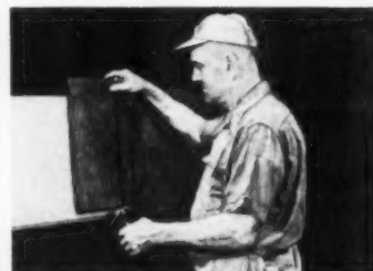
Kerf in butt of shingle is engaged in clip
