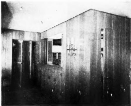
Guest closet in foreground is in end of room-separating wall between reception hall and living room. Accordian-type louvered doors at rear open to bedroom hall. 1x10 V-cut vertical pine paneling is used throughout
