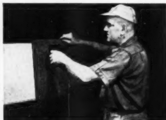
Only one staple secures each shingle at top
