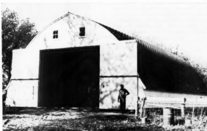
The laminated arch is a characteristic modern development that provides ample post-free interior space and permits a wide choice in building materials
