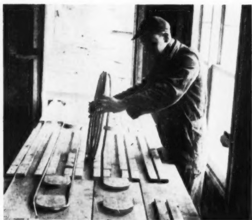
Simple bending templates are useful to produce uniform bends and even spacing of the row of tubes in a heating coil. Soft annealed copper tubes in 60-foot lengths require fewer joints, reduce installation time and expense
