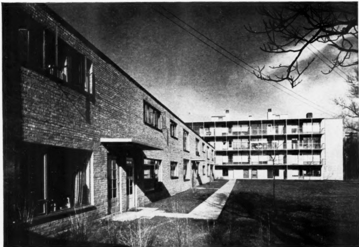
Pioneer Cooperative Apartments, Chicago, Illinois. Architects: George Fred Keck and William Keck, Chicago. Contractor: Perry Construction Company, Chicago. Windows: Lupton Steel Residence Casements, Fixed Windows and Architectural Projected Windows.
