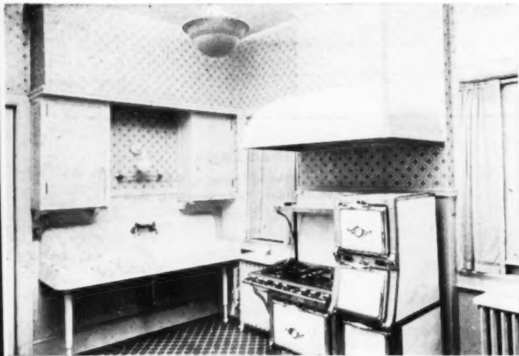
FIGURE 2. Designed in the 1915-25 period, this 200-watt totally indirect fixture gave a soft light that was almost completely shadowless. The low ceilings in today's homes do not allow the necessary suspension for achieving this even distribution of light. There are few if any kitchen fixtures on the market today that can equal its performance
