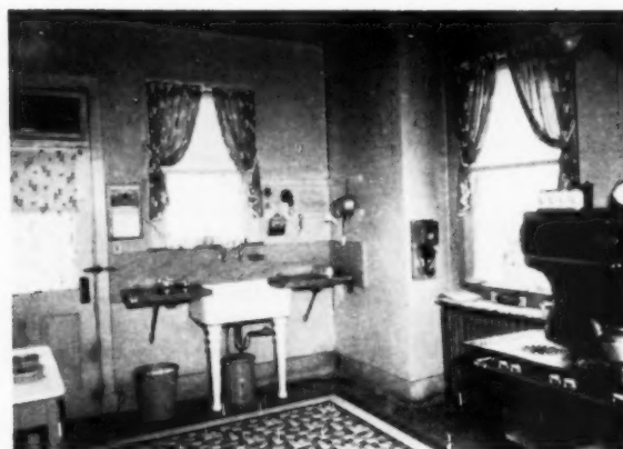
Kitchen of 1912 has sink mounted on legs, wood drainboard
