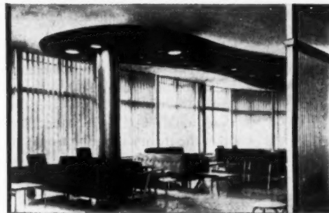
The pictures at right show how Milcor Metal Lath and plaster were used in the same building to create a modernistic column and protect it from fire and impact. Dead loads were reduced, because Milcor Metal Lath and plaster weigh less than masonry and concrete fireproofing.
