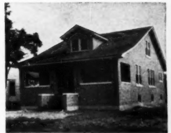
Perhaps the most significant house of pre-World War I was the bungalow. House at right shows the bungalow form at its most prosaic. Above is a California bungalow of 1910 designed by a follower of the Greene brothers
