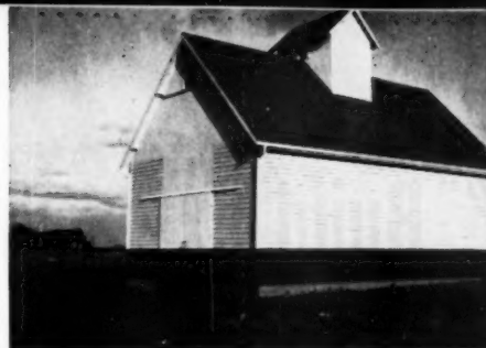
The double crib with center drive and overhead grain bins is still one of the most widely used types but will change drastically in the future (see Forecast below)
