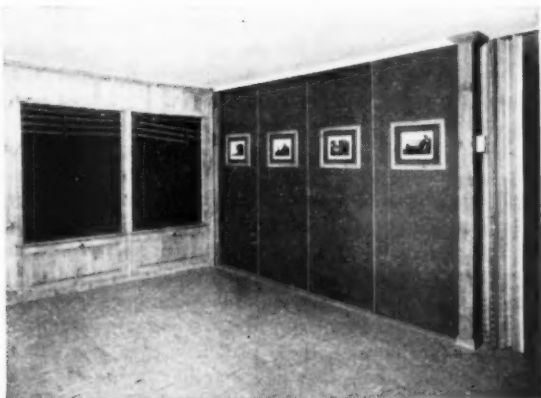
Fabricated window wall panels as well as sliding door partitions are also already being used in component construction operations by home builders
