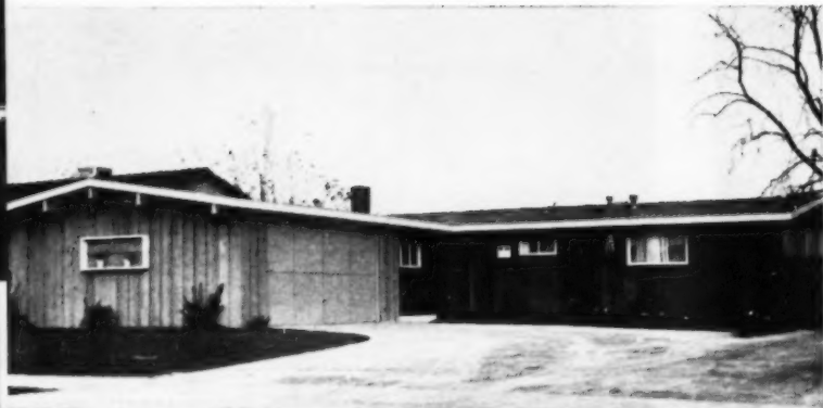
Today's house is compact but achieves a sense of spaciousness by open planning and emphasis on outdoor living. The outdoor
