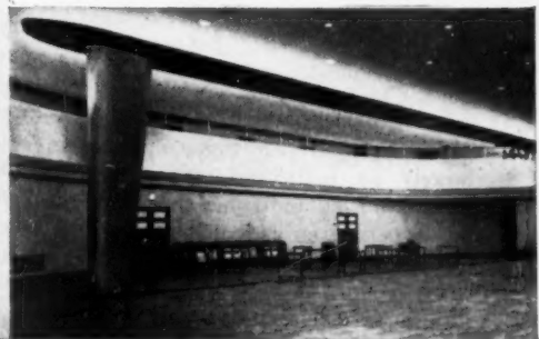
The pictures at right show how Milcor Metal Lath and plaster were used in the same building to create a modernistic column and protect it from fire and impact. Dead loads were reduced, because Milcor Metal Lath and plaster weigh less than masonry and concrete fireproofing.
