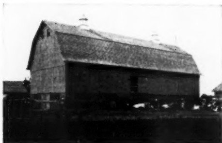
After 1900, the self-supporting gambrel roof with braced rafters became more common. Walls of more modern gambrel roof barns were often framed of lighter material such as 2 by 6's spaced 16 or 24 inch o.c.
