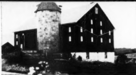
1880-1900. Typical bank barn. Two stories with large mow, gable roof, heavy timber framing mortised and pegged together. When a bank location wasn't possible, a ramp to mow floor was often built. Stable on lower level
