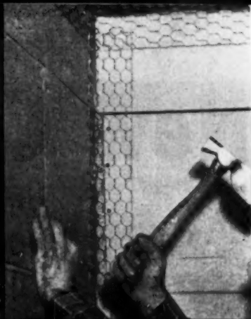
Preformed —Keycorner is preformed for corners, joints, ceiling junctures. Flex it and it fits right in.
