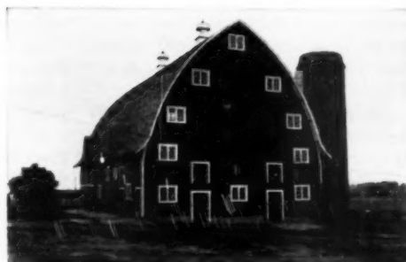
By 1920, the gothic roof had appeared. Early examples used sawed rafters or bent rafters made up of small boards bent to form segments of the arch and nailed together. Later, rafters were glued up and were often prefabricated
