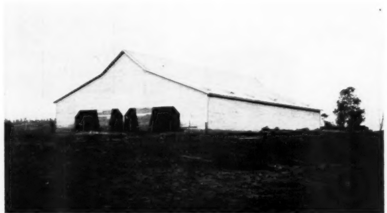
Self-feeding barn (above) and low-cost pole barns for the storage and self-feeding of hay for beef cattle began to be built as early as 1900. They became practical only fairly recently, however, when pressure-treated lumber and poles helped solve the problem of poles rotting out
