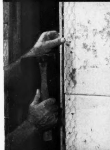
Solid Corners —Keybead's precision-formed bead on open mesh fits all outside corners, quickly, easily. Full, solid corners result.
