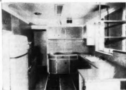
Kitchen has deep coved white ceiling with trim painted to match color of tiled walls. Built-in oven has hot dish shelf above
