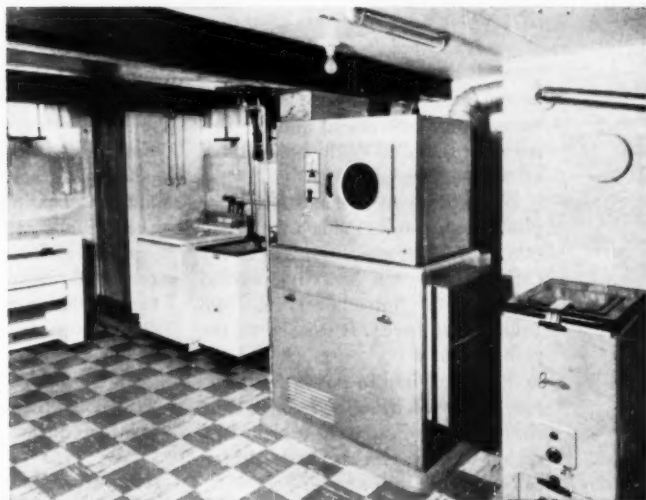
The development of the furnace fan revolutionized warm air heating. Yesterday's mammoth equipment no longer chokes the basement. Downflow furnaces can be installed in closets, attics, are as neat as a button
