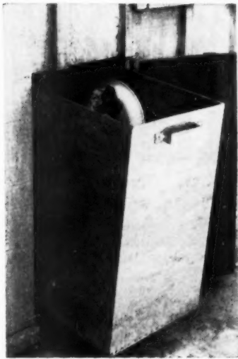
Metal pull-out container is large enough to hold at least one week's accumulation of refuse
