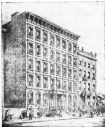
A Fifth Avenue apartment house, New York City, 1880
