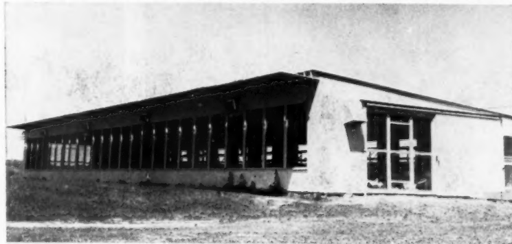
This poultry house design shows the trend toward specialized, large-scale production. It utilizes mechanical equipment for efficiency and such modern elements as the low-pitched roof, insulating windows, protective shade, and controlled ventilation
