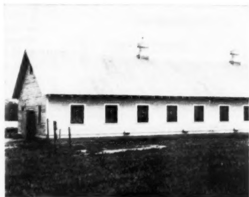
With the advent of the hay baler and chopper, the large storage mow became outmoded. This led to the modern 1 1/2-story braced rafter barns and the
