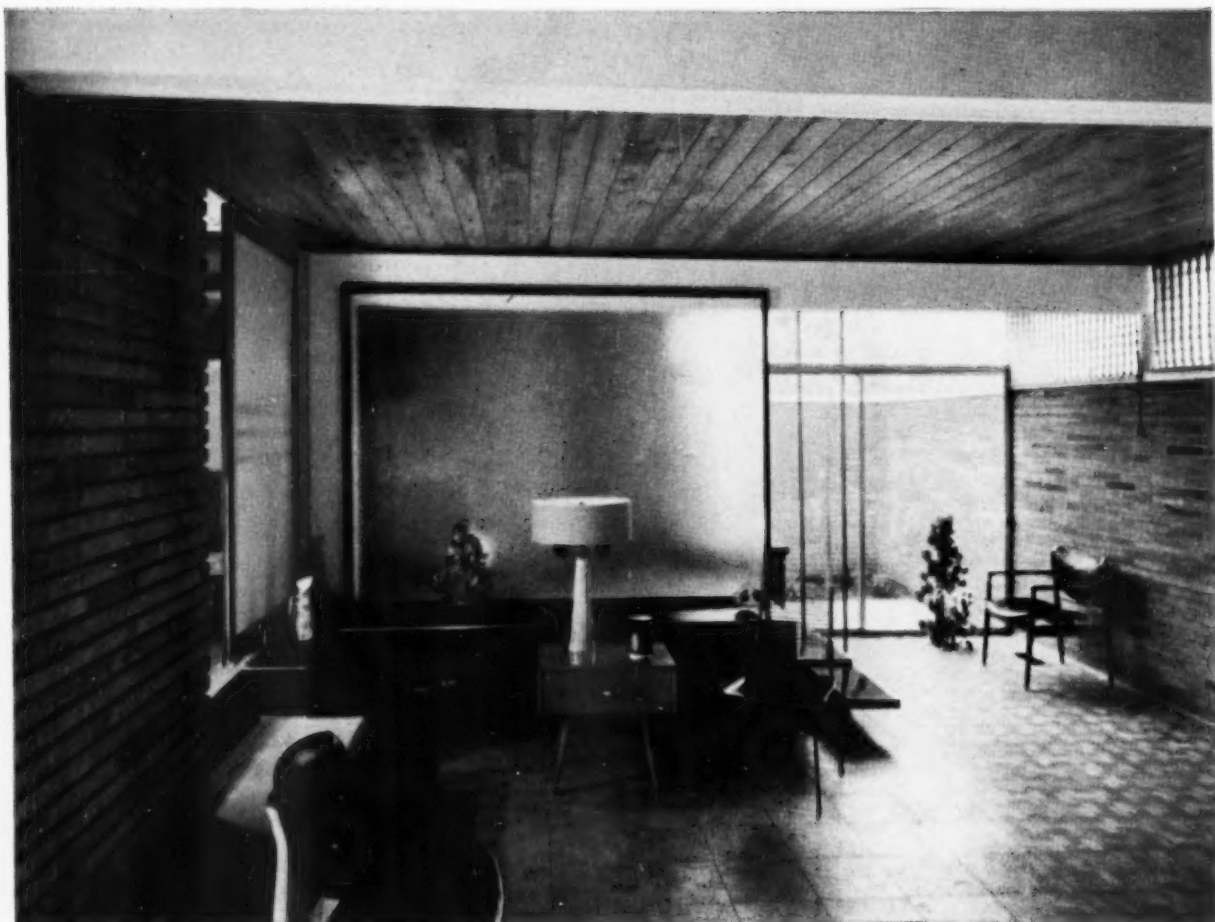
Ribbed, opaque glass panel separates entrance hall at normal level from living room, with counter and book shelves below. Sliding glass panels at right of living room give access to formal courtyard
