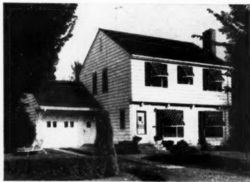
The deep shadow lines of bevel siding emphasize the length of this home and enhance the simplicity of the design.
