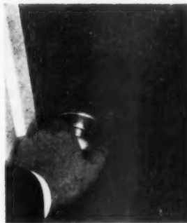
Standard lock installation—Note the lack of knuckle clearance.
