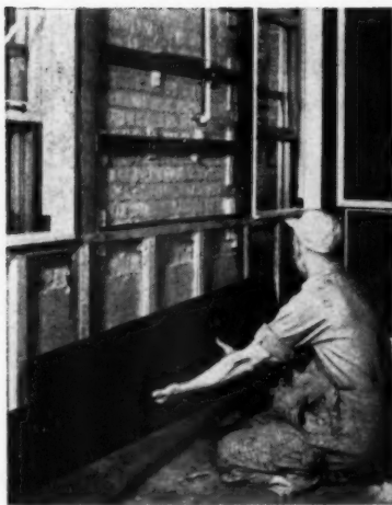
Wainscot is hardboard installed with adjacent edges flared out
