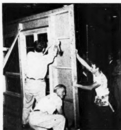
Workmen locating Lu-Re-Co wall panel
