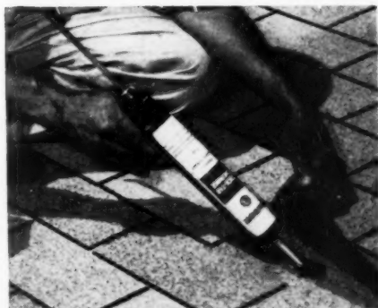
Shingle tabs are quickly, easily and surely cemented down with Flintkote's Stik-Tab Cement.
