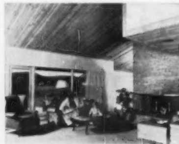
AB15090 — LAMINATED RANDOM WIDTH LUMBER — SHERMAN, BOOTHS 537-538 —West Coast Lumbermen's Assn., Dept. AB, 1410 S. Morrison St., Portland 5, Ore. Striking new texture for ceilings is achieved with laminated random thick dimension Douglas fir or West Coast hemlock laid solid as illustrated above. Economy results from use of lower grade lumber, elimination of ceiling insulation, rafters or joists and roof boards.
