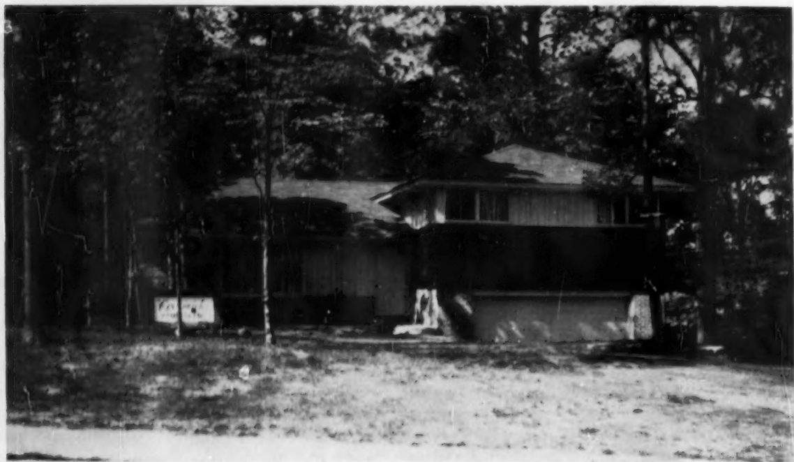
"Crosswicks Provincial" is set in wooded lot with at least 100-ft. frontage. Hip and gable roof blend well and Redwood clapboarding helps establish horizontal lines of house
