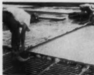
AB15298—PERLITE-METAL ROOF —Perlite Institute, Dept. AB, 10 E. 40th St., New York 16, N. Y. Lightweight perlite concrete is now approved as insulation over aluminum roof decks as well as over light-gauge steel decks and other types of permanent forms. The perlite concrete conforms to the shape of corrugated or cellular-type metal decking and increases strength, fire safety and rigidity.
