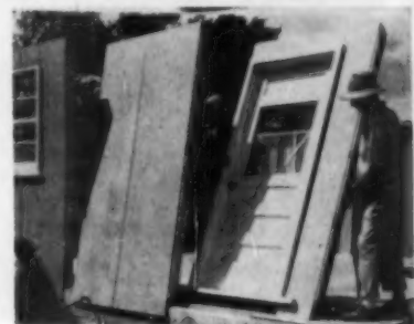
AB15364 — PRE-BUILT HOUSE — HILTON, BOOTH NO. 327 — Wadsworth, Inc., Dept. AB, 2949 Chrysler Rd., Kansas City, Kans. Shown are three of Wadsworth's basic wall sections: a 4-ft. modular window unit, 4-ft. blank or filler modular unit, and a 4-ft. door-rear assembly. Builders select the doors and windows desired for units. House also has pre-built truss units and modular units for interior.
