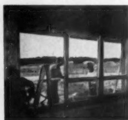
Workmen easily install Flexivent Units . . . either as assembled groups or built up in opening.
