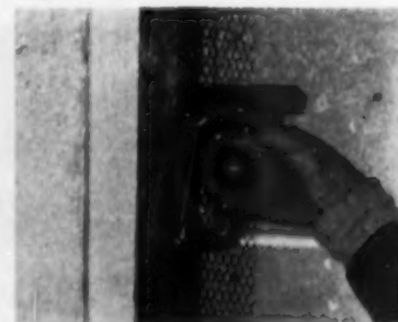
AB15372 — GUN TACKER — Fastener Corporation, Dept. AB, 860 Fletcher St., Chicago 14, Ill. Many builders are finding that the Duo-Fast Gun Tacker CT 859 which drives a heavy duty staple does a fast easy job of tacking up Cornerite. The one-hand operation enables workman to hold corner material snugly in position during the tacking operation, thus speeding the operation and saving labor costs.
