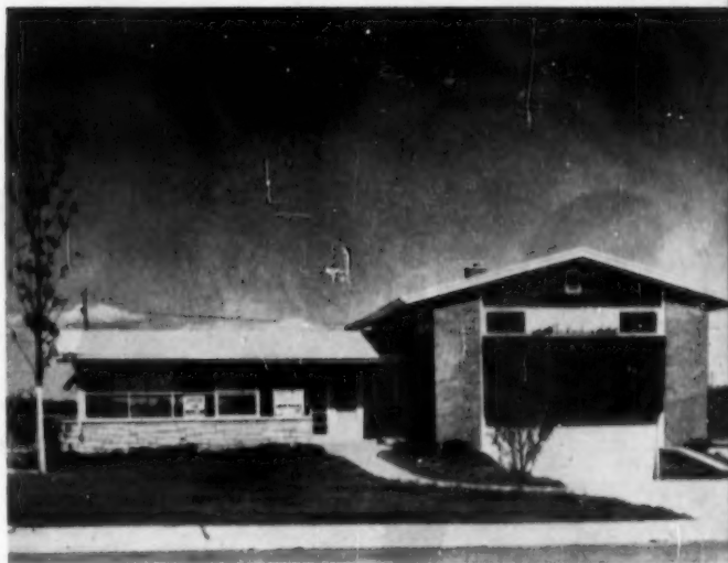
Low-pitched roof lines modern window treatment; straightforward use of materials give split level a contemporary look. Roof surfacing is of marble chips
