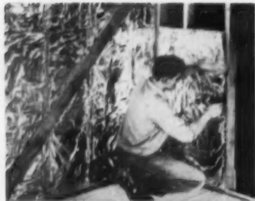
AB15165 — REFLECTIVE INSULATION — HILTON, BOOTH 15 — National Gypsum Co., Dept. AB, 325 Delaware Ave., Buffalo 2, N. Y. The new Gold Bond Twinsulation combines the insulating efficiencies of rock wool and reflective aluminum surfaces. The side of the blanket that faces the building interior is aluminum foil, while the exterior side is aluminum coated. Rock wool inside the casing also blocks passage of heat.
