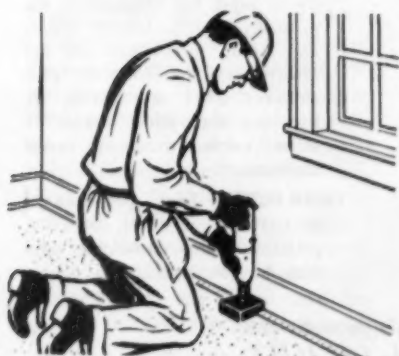
Carpet gripper anchored to concrete
