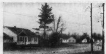
Part of the 147-house project at Cedarcrest, a charming, wooded section of Canton, Mass. Ranch houses, priced from $10,400, have heating comfort of custom-built homes. Builder: Frank Losordo Sons, Inc., Hyde Park, Mass. Heating Contractor: Frank Losordo.
