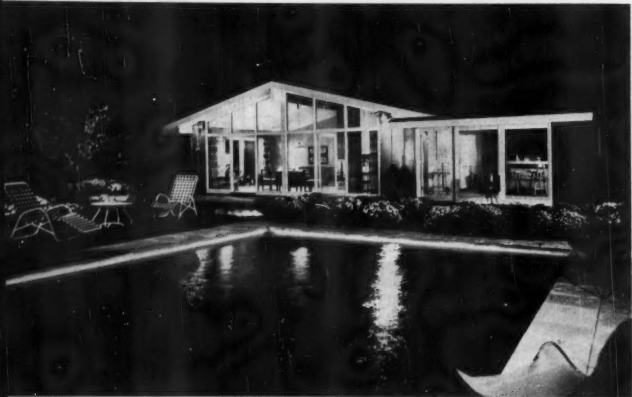
The structural profile of the house is clearly outlined by the window openings
