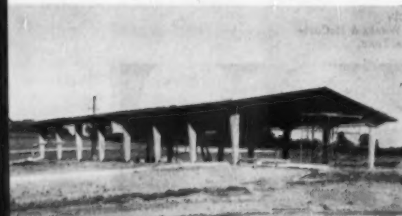
Only one more channel roof slab remains to be installed to complete first section
