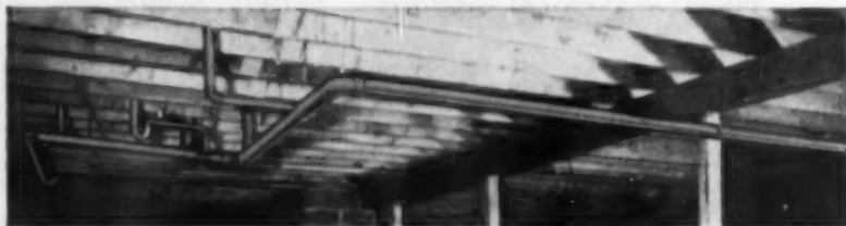
FAST, EASY-TO-MAKE JOINTS. Solder-type fittings save hours. No threading, no pouring and caulking.
