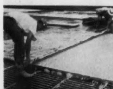
AB15298—PERLITE-METAL ROOF —Perlite Institute, Dept. AB, 10 E. 40th St., New York 16, N. Y. Lightweight perlite concrete is now approved as insulation over aluminum roof decks as well as over light-gauge steel decks and other types of permanent forms. The perlite concrete conforms to the shape of corrugated or cellular-type metal decking and increases strength, fire safety and rigidity.
