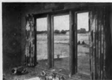
Casement position. Sash swing outward. When placed on end the versatile Flexivent provides an excellent low-cost casement window.
