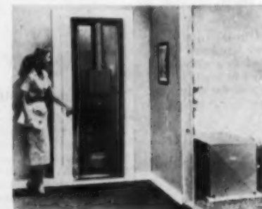
AB15385—AIR CONDITIONER FOR COUNTERFLOW SYSTEMS—SHERMAN, BOOTHS 401-402 —Carrier Corp., Dept. AB, Syracuse, N. Y. Latest Carrier Conversion Weathermaker is designed to convert down-flow forced warm air furnaces to year 'round air conditioning. Furnace is lifted few inches and small counterflow coil placed underneath. Furnace blower sends air downward. Illustration shows typical installation in basementless home.
