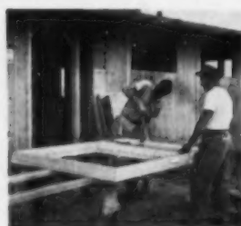
Completely packaged Flexivent Units are easily assembled on the job for immediate installation.
