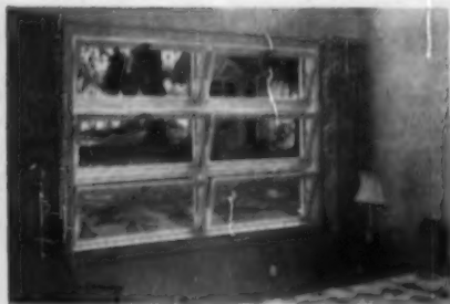
Hopper position. Sash swing inward. Easy to operate. Easy to clean outside glass surfaces from inside house. Better control of ventilation.
