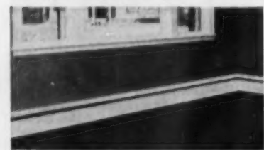
Webster Tru-Perimeter Forced Hot Water Baseboard Heating offsets heat loss beneath large window areas and along all exposed walls.
