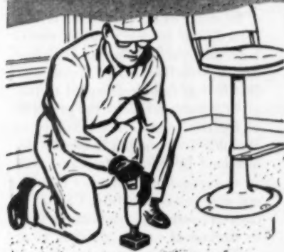
Anchoring seats, bar stools to concrete
