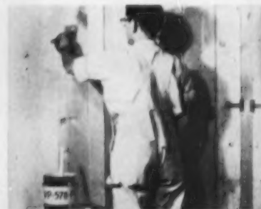
AB15198—PRIMER KNOT SEALER—SHERMAN, BOOTHS 539-540 —Western Pine Assn., Dept. AB, Yeon Bldg., Portland 4, Ore. A new primer knot sealer, WP-578-P, is a further development of the clear sealer formula, WP-578, and combines sealing and priming cost steps into one operation, thus adding new economy to the use of lower grade lumber where painted surfaces are desired. The sealer prevents possible paint discoloration.
