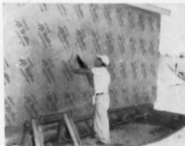
AB15076 — SHEATHING—HILTON, BOOTH 20 —The Upson Co., Dept. AB, Lockport, N. Y. "All Weather" sheathing is a laminated wood fibre panel waterproofed through its entire thickness of six plies. Made in all standard sizes, plus the "king sizes" of 8 ft. wide by 12, 14, 16, 18 and 20 ft. long, panels saw clean like wood, have efficient insulation value. Exceed requirements of FHA Technical Circular No. 12.
