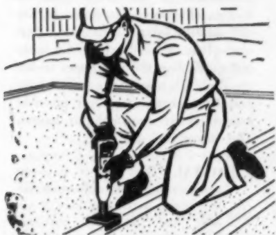
2" x 4" plates to concrete floor
