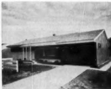
AB15052—PREFABRICATED HOME —HILTON, BOOTHS 166-167 —Modern Homes Corp., Dept. AB, 14507 W. Warren Ave., Dearborn, Mich. This model features open planning, sound "conditioning" of bathroom and ceiling, modular construction, "Klear-Span" (steel joists with wood panel decking) floor system, and a scissors truss which provides 10-foot vault-type ceiling. Modern's new "Power-Glide" sliding windows are included in all models.
