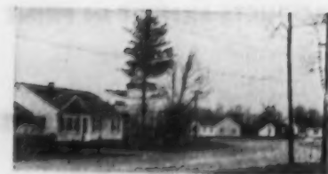
Part of the 147-house project at Cedarcrest, a charming, wooded section of Canton, Mass. Ranch homes, priced from $10,400, have heating comfort of custom-built homes. Builder: Frank Losordo Sons, Inc., Hyde Park, Mass. Heating Contractor: Frank Losordo.
