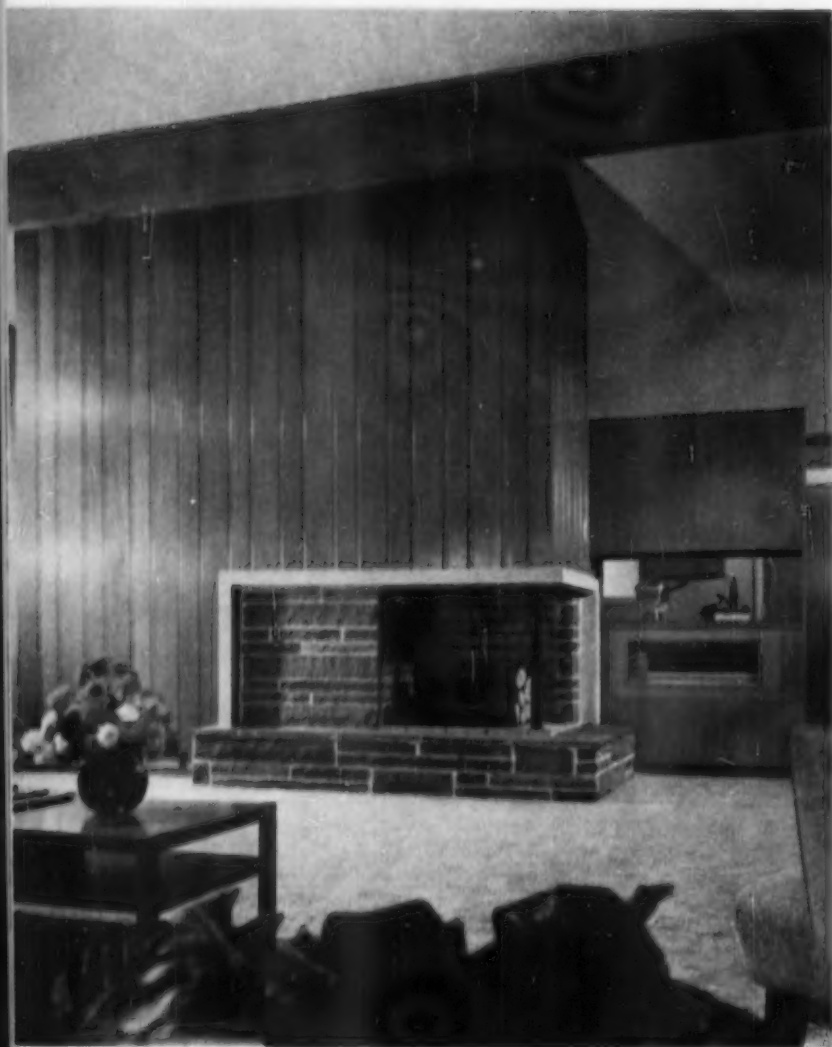
The fireplace and its position at the intersection of the living-dining room helps make this area sparkle with interest. The opening is framed with a band of Bedford stone on top and sides, with random field stone used for the panel and the raised hearth. The surrounding walls are faced with vertical redwood
