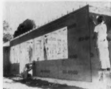
AB15173 — INSULATING SHEATHING—SHERMAN, BOOTHS 493-494 —Wood Conversion Co., Dept. AB, First National Bank Bldg., St. Paul 1, Minn. Improved Nu-Wood sheathing has greater surface protection and increased nail-holding strength. New nailing guide lines make application faster and easier. This sheathing is asphalt impregnated, can be used under wood siding, wood and asbestos shingles, stucco or masonry veneer.
