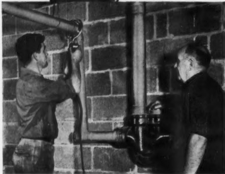
FAST, EASY-TO-MAKE JOINTS. Solder-type fittings save hours. No threading, no pouring and caulking.
