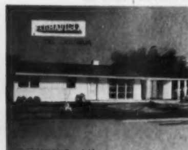
AB15294 — PACKAGED HOUSE —Permabilt Manufactured Homes, Inc., Dept. AB, 330 S. Kalamazoo Ave., Marshall, Mich. All exterior walls come built up in panels for 8-ft. ceiling height and in even lengths of 2 ft. to 12. ft. (mostly 4-ft. for easy handling). The package is complete and all materials are standard sizes and quality grades. This model is offered for the $12,000 to $14,000 market.
