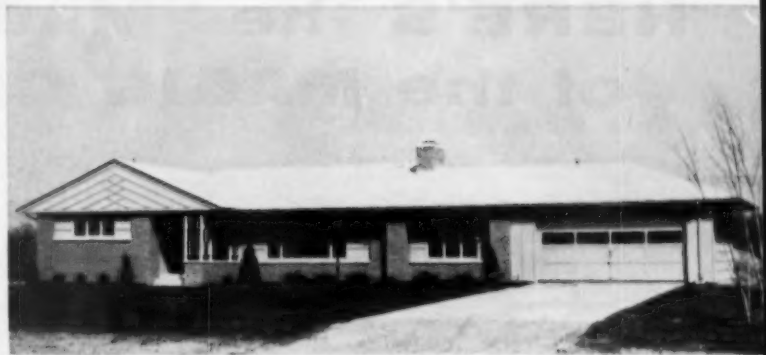
Typical of the houses that will be built in Forest Hills is this one by Harold Johnson
