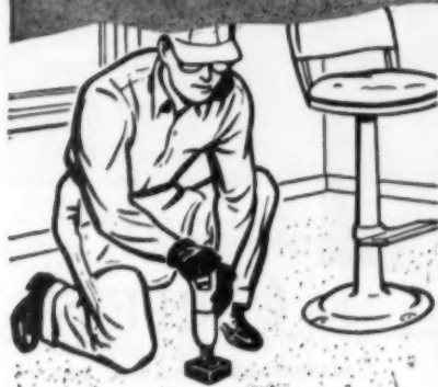
Anchoring seats, bar stools to concrete
