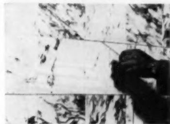
A string is used to space the tiles correctly, row after row. It can be removed after all the tiles are set, or row by row
