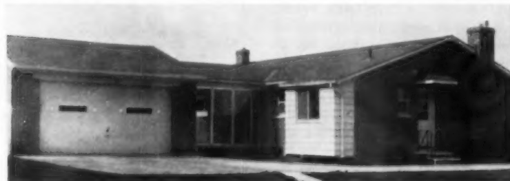
Turnaround drive is sloped to eliminate puddles of water or icy spots
