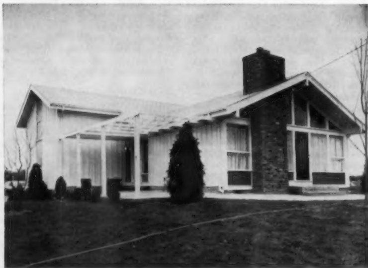
Front porch with overhead trellis is 25 feet long, abuts board and batten walls
