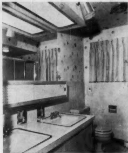
Soffit lighting over lavatory in bathroom of Brynhaven house has a 2-40 watt rapid start warm white fluorescent lamps controlled by wall switch in bathroom as well as by three other wall switches, one in each bedroom
