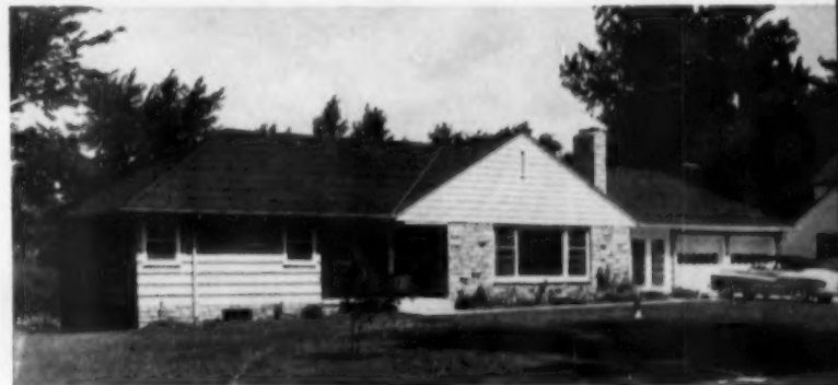
Emil Fronk plans houses of this size for Forest Hills, to be built on contract only
