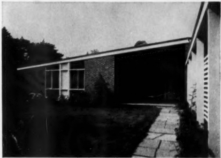
STREET SIDE , partial view at carport. Entrance porch is large enough to be used for auxiliary dining. Note that the roof line is flush with the wall on this side
