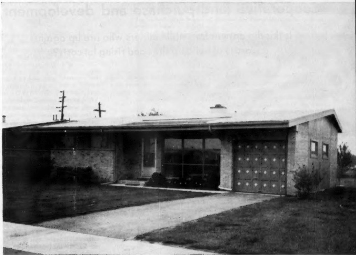
The owner of an identical house, plan reversed, has now enclosed the carport with frame on two sides and an upward-acting door on the front
