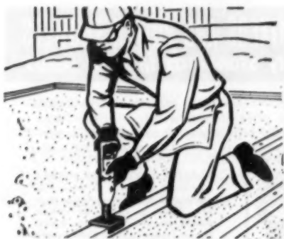
2" x 4" plates to concrete floor
