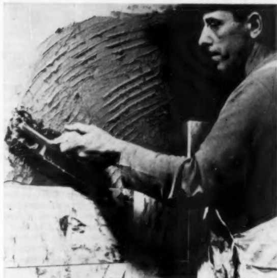
Markwa marble tile can be applied with adhesive or mortar. The adhesive is spread with notched trowel, covering only the wall space that can be tiled in an hour's time
