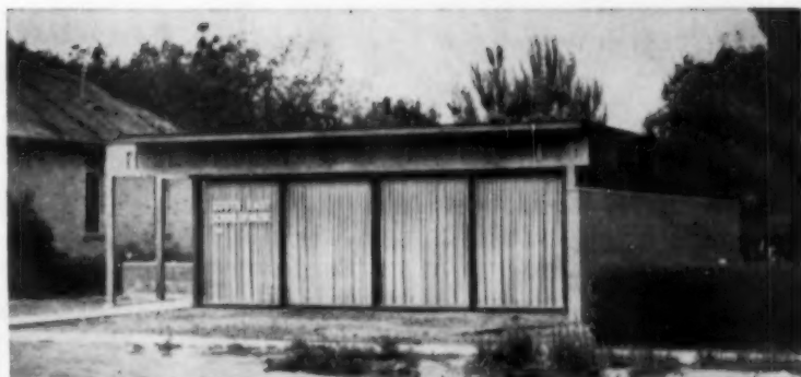
In simple, cost-reducing system, span of plywood girders eliminates interior load-bearing walls
