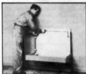
Frame is fastened directly to studs with lag screws.
