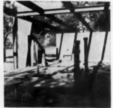
Construction photograph shows the steel in place and the plumbing core for interior bathroom-utility area
