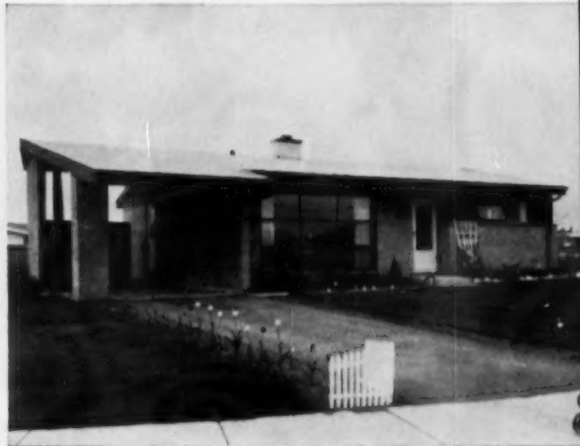
The extension of the roof line over to the corner masonry piers forms an inexpensive carport, open on three sides except for a group of storage units which extend part way up on the rear wall. BUT . . . see below
