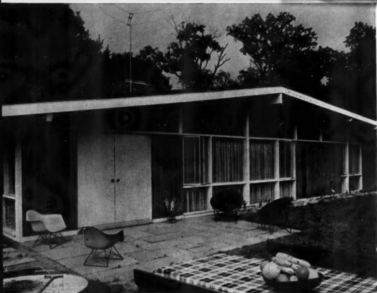
GARDEN SIDE has clerestory windows which form an interesting pattern under the wide gable roof sweep. Walls are faced with vertical cypress and brick
