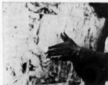
All joints are filled with white Portland non-staining cement mixed with water to consistency of thin cream, and spread on with the hand. Excess grouting cement is washed off later
