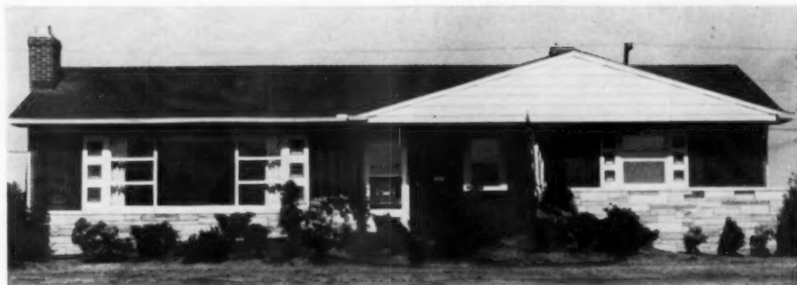
Slight ramp from driveway eliminates step at entrance, has rough finish
