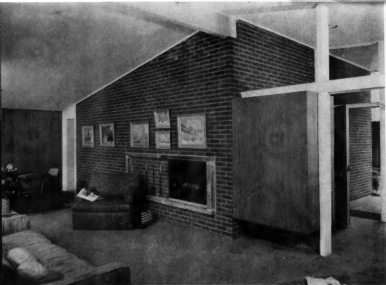
GUEST CLOSET is suspended from exposed horizontal and vertical supports
