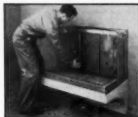
Hearth and firebox are formed of interlocking ceramic sections.
