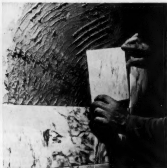
No adhesive is placed on tile, but tile is pressed into adhesive firmly and twisted in place. Tiles are applied just as they are lifted from the package
