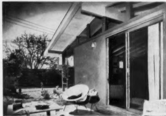
TYPICAL EAVE DETAIL Roof planks are carried out to eaves. Fascia board on end of rafters forms a natural gutter
