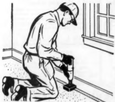
Carpet gripper anchored to concrete
