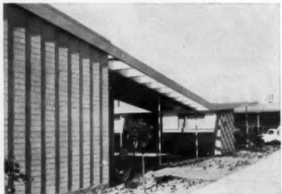
Shadow effect is given by concrete block wall. Rafters slant downward for butterfly design
