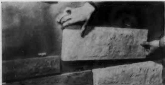
Emco-Rok is supported and held to the wall surface by galvanized clips
