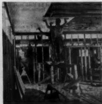
By noon, the drywall men were installing ceiling
