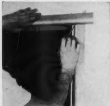
Trim must be measured for accurate fit. Head trim is cut to proper length with aviation Metal Master tin snips
