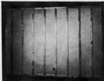
Paneling can be bonded directly to studding or to furring strips applied over existing walls (as shown.) Where planks or squares will be used, furring strips are applied horizontally.
