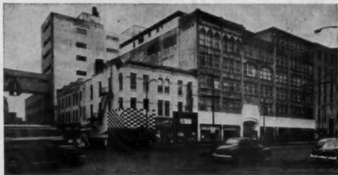
GIVES UNITY and outstanding design to a set of old and new buildings
