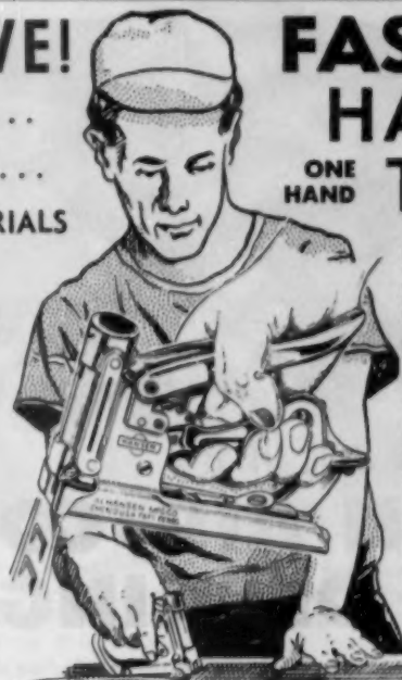
Tacking screen to lath to make reinforced corner.
