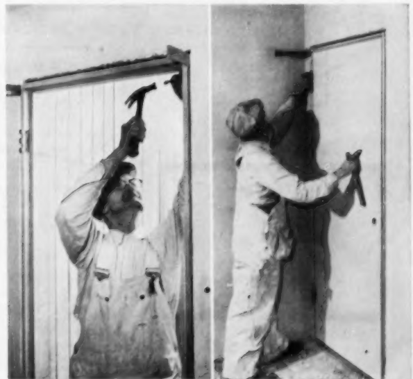
Doors and frames are delivered at the site ready for installation. Only work remaining is to true these members in the wall openings and install finish hardware
