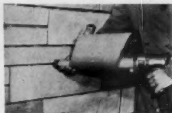
Clips and nails are completely imbedded in mortar. Each stone is held solidly to wall
