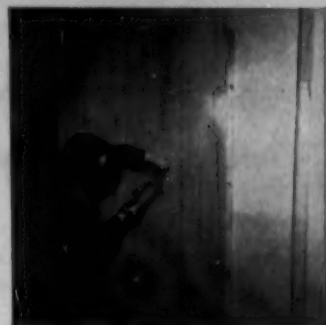
Bond is completed by tapping over the areas of contact with a hammer and a small block of wood. Bonding is immediate upon contact—no sustained pressure is required.
