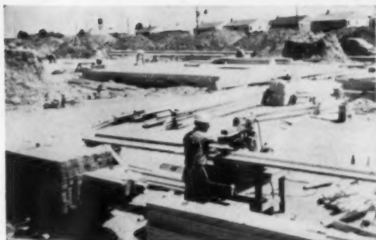
RADIAL SAW on skids is set at pile of 500 2x4's, enough for two houses. After cutting by specially detailed man, studs are moved by laborers a few feet to building site
