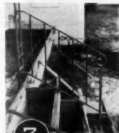
3 Standard step forms for 7" risers & 12" treads.
