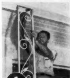
1 Hang post to soffit with lag screws.
