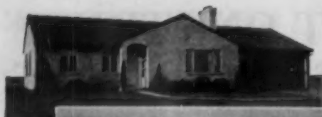
Residence of J. C. Davidson, Manager, Application Engineering Department, Airtemp Division, Chrysler Corporation, Dayton, Ohio. Completely air conditioned with Airtemp equipment and Kno-Draft Overhead Air Diffusers.
