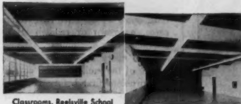
Classrooms, Reelsville School
