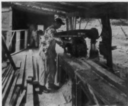
CUT-OFF SAW is workhorse of Gaddy pre-cutting operation. Long saw table extends clear through shed in background, where 2 x 6 window frames are routed out after initial cuts have been made on saw. Frames are then assembled in shed
