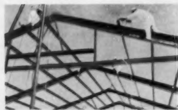
Cross members and reinforcing rods go in place to complete frame
