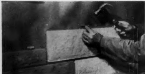
Both the top and bottom of Emco-Rok are secured to the sidewall
