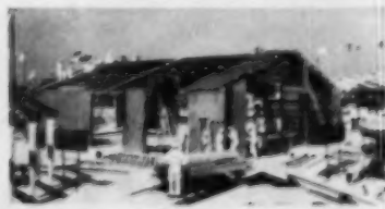
Near completion. Job was far advanced in less than four hours
