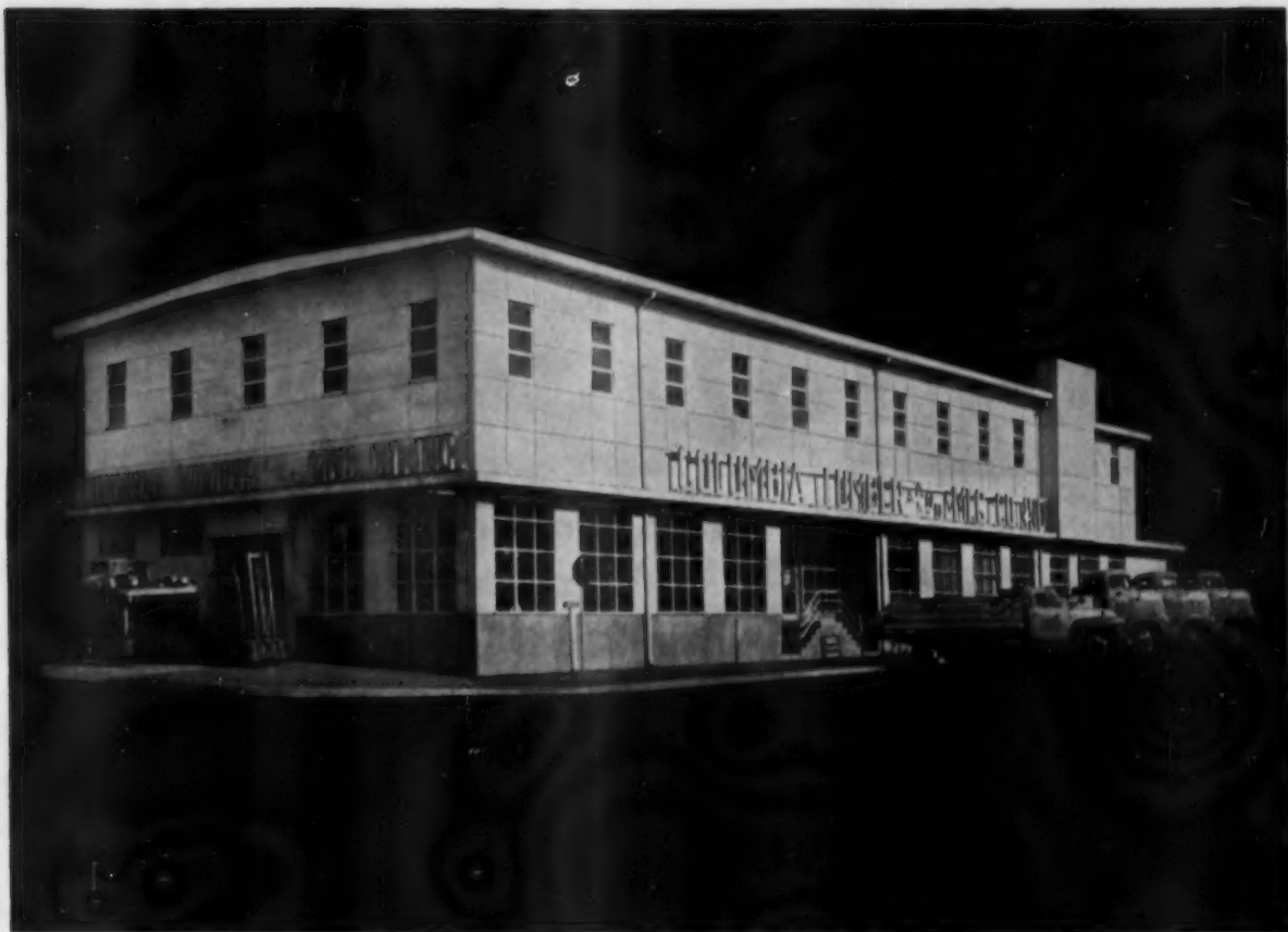
K&M APAC SHEETS GO UP EASILY, furnish a smart, modern appearance. In the picture above, they've been applied on the sidewalls of the Columbia Lumber & Manufacturing
