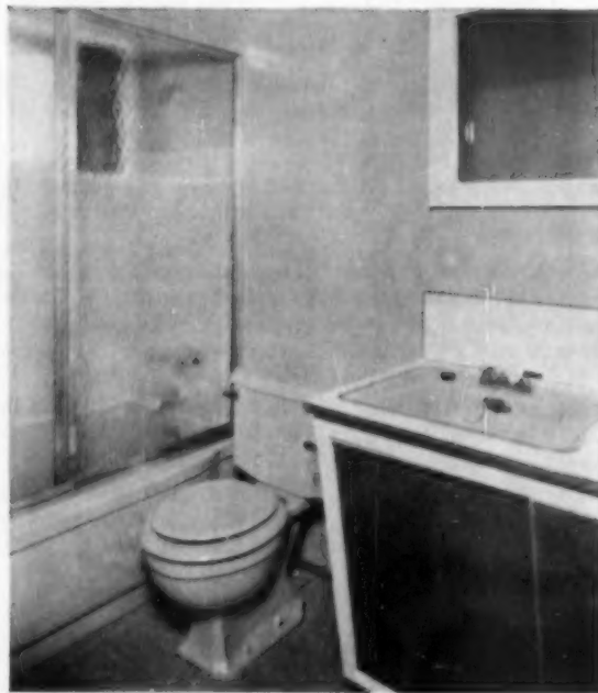
TWO BATHROOMS: Glass shower enclosure and built-in lavette are part of the package
