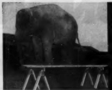
BRACKETS HOLD TREMENDOUS LOAD
