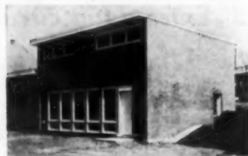
Series of windows at rear looks out on area to be landscaped for patio
