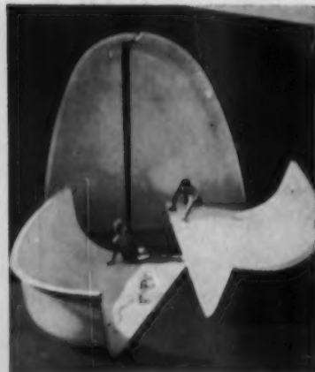
The four sections of reinforced Fiberglas are nested for shipment
