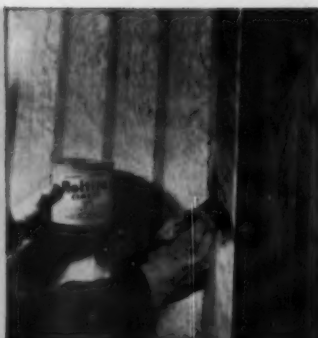
Apply Roltite to the furring strips and to the corresponding areas on the back of the panels. Do not coat the first 1/4" along the edge which will be used to swing the panel into place.
