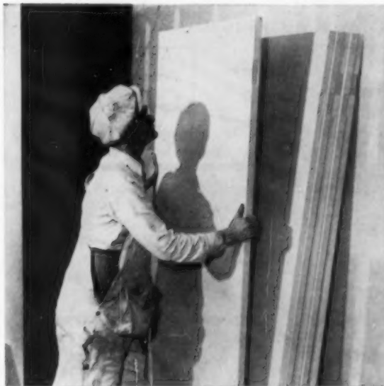
Doors and frames are delivered at the site ready for installation. Only work remaining is to true these members in the wall openings and install finish hardware
