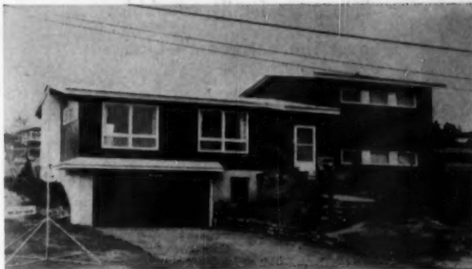
DARK RED VERTICAL PLANKING , stone approach, and marble chip roof make a striking exterior of this $35,000 four-level. An insul-metal flue serves the year-round conditioner. Plans show full bath room facilities on each of two bedroom levels.
