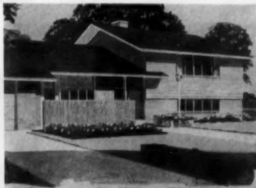
SAME SPLIT level with attached garage. Unlike version plan is only possible when all jogs and angles are fitted on far left, it has in-line plan. Extreme flexibility of into one simple rectangle of two-to-one proportion.
