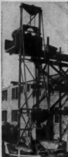
Cut placing costs —Jaeger Self-raising "Hoister" Tower makes quick work of material placing, saves labor. Assembles easily in 10' sections to 67'. 1-ton capacity. Available with material cage or 14' bucket. Easy to move. Positive automatic safety device.
