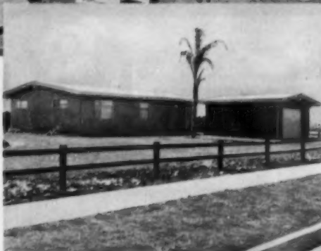
ONE OF THE HUNDRED completed homes shown in the large aerial view above. There will eventually be 350 homes in this tract. 34,000 feet of enduring Revere Copper Water Tube have already been installed in the first hundred homes in 1/2", 3/4" and 1" sizes. Bidr. and Gen. Cont.: M. J. BROCK & SONS, INC., Los Angeles, Calif. Revere Dist.: KEENAN PIPE & SUPPLY COMPANY, Los Angeles, Calif.
