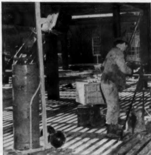
TAKING COUNTRY by storm, this portable infra-red heater burns LP-Gas. 100 lb. tank will supply spot-heater for 55 hours. Though not yet in full production, company should be by winter. Some dealers will rent unit.
