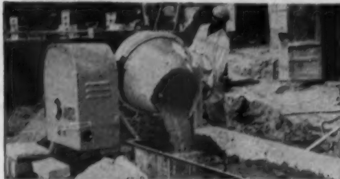
Mix better, pour faster —Jaeger 3 1/8 Tiltler drum has patented "dual mix" V-bottom that gives double the mixing action of ordinary tilters and also speeds discharge. Produces big daily yardage of high strength, high quality concrete or mortar. Tows fast, spots fast.
