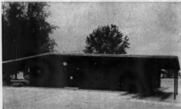
CLINIC has masonry bearing walls, interior bearing partitions. Roof is 4-in. decking above beams and walls. (Photo: Hutchings-Newman)
