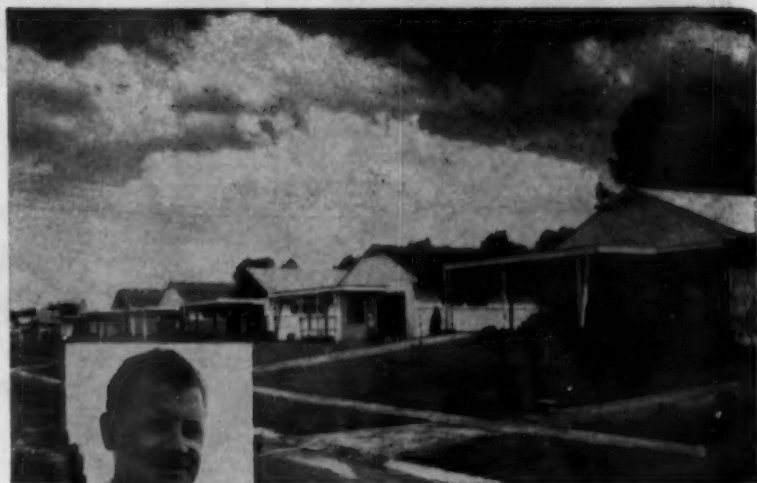
Another group of Fadco-built homes, Cincinnati, featuring Alfol in ceiling and sidewalls. Inset: E. B. Fadden, Pres.
