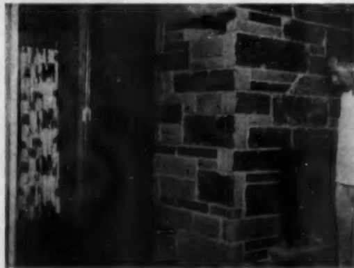
MASSIVE FIREPLACE of Lenroe stone from nearby Ithaca anchors the open-planned dining-living room section of Putvin's house. Hufcor doors at extreme left and at kitchen wall provide flexible command of space.
