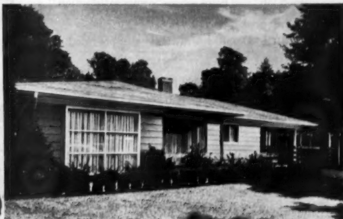
Planning, Design —Handsome contemporary design, efficient space-making floor plans mean lasting livability and appeal. A wide range of models and sizes enables you to meet any market.
