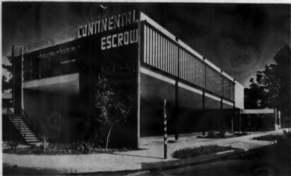
ANGLED wall gives big overhang with built-in lighting, which adds to striking effect of planter-wall.
