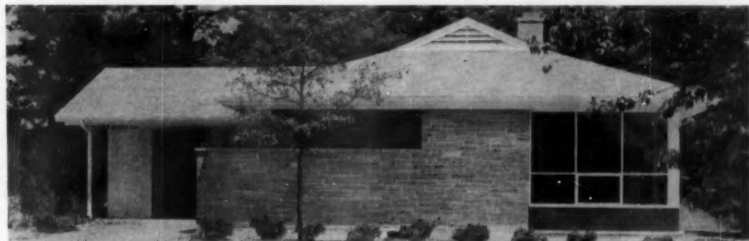
STILL ANOTHER version of Manilow house: ranch with carport storage, louvered roof—and stone front. Where masonry is used it definitely predominates; wood siding is used only for contrast. Roof is asphalt shingle. This
