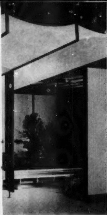
BARREL VAULT ROOF PANELS WITH CONCAVE SURFACES COMBINE STRUCTURE AND ORNAMENTATION
