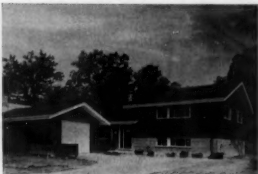
FAST-SELLING split level looks large on lot, is same size as ranch. Breezeway joins garage and house. Lower level is family room, with bedrooms above. Exterior of house is redwood and common brick; garage door, trim are white.
