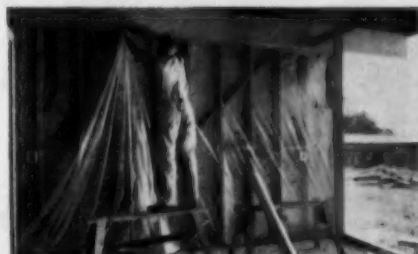
VISQUEEN film locks moisture out of studwall, prevents damage to insulation, paint peeling, rot.
