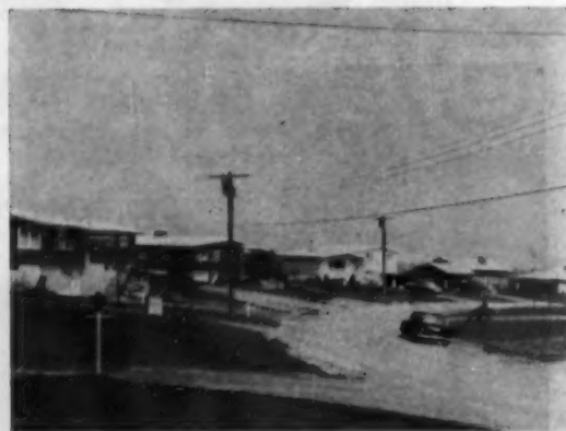
LIGHT COLORED ROOFS are a clear indication that Syracuse builders recognize effectiveness of marble chip and light shades of asphalt shingle in reflecting sun radiation and lowering heat load.
