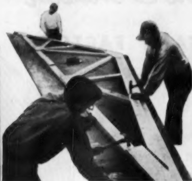
Craftsmanship —Main sections of Harnischfeger Homes are built in forms under rigidly controlled conditions.
