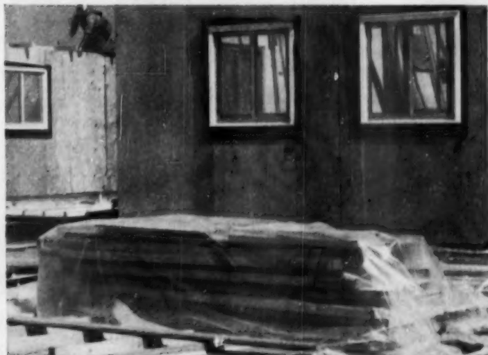
No water can reach materials or tools that are protected by VISQUEEN film
