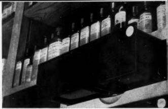
Drawers are shipped completely finished, no sanding, no cutting, While handles and pulls can be easily added, in this installation the frame of the cabinet was notched to provide a finger hold.
