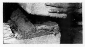
It is easy to build up reinforced corners with KEY-WALL. Short lengths may be cut and used without reducing effectiveness of reinforcement.
