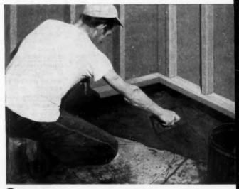
Spread mastic over waterproofed slab.
