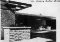
Concrete brick with extruded mortar joints and long law split units combined in this ranch type home.
