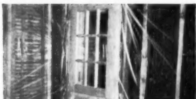
Olin Polyethylene as a moisture vapor barrier on warm side of walls retards paint blistering, peeling, staining. Helps keep out drafts—permanently.
