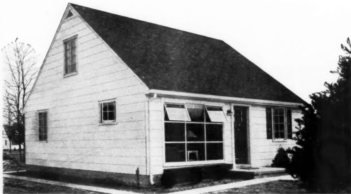
House in 200-unit project, Maryland. Contractor-BUILDER: Admiral Construction Corp.
