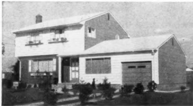
CLEAN LINES of two-story house (not a split) by Charles Rubelsky are softened by shutters, planter boxes ($31,000). Multi-levels are now found wherever land is high-priced or hilly. Bethpage, Long Island.
