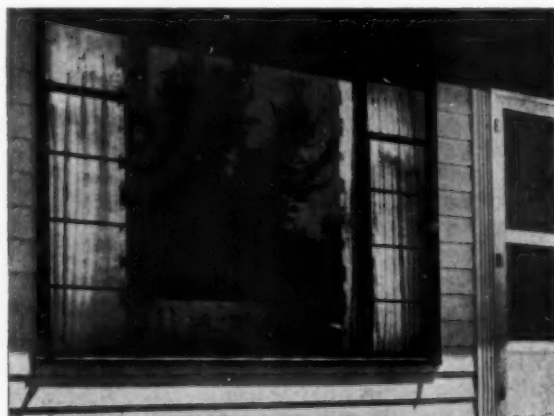
In this cottage, a fixed picture window is flanked by casement-type windows. Thanks to steel's rigidity and its freedom from warping, these casement windows will stay easy to open and close for many years of service. And occasional painting will keep them good-looking for the life of the house.
