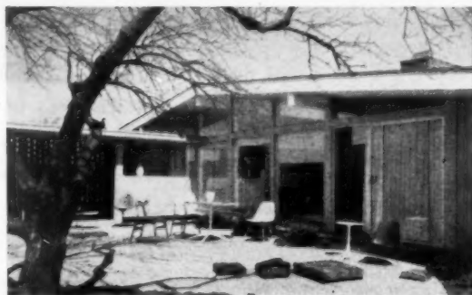
GLASS WALL of Rodney Lockwood's contemporary is protected from street by brick wall to entrance (center) and garage off left. Fixed glass under gable is protected by generous overhang. Detroit, Mich.
