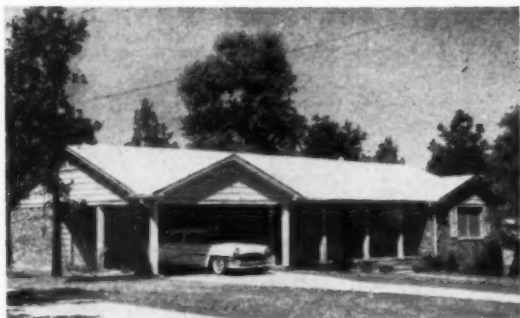
REPEATED GABLE , extended roof and covered walk to entrance (see p. 88) show carport is built into basic design of brick colonial. Symmetrical facade lends formal dignity to design. Vondal Gravlee, Birmingham, Ala.
