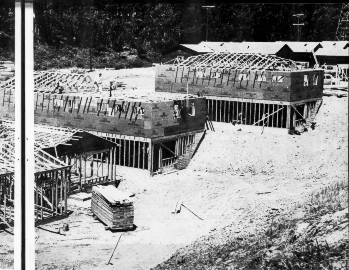
PROBLEM OF BUILDING ON SLOPING LAND is graphically shown here. Each house has own concrete retaining wall.
