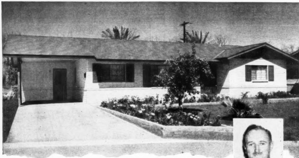
A typical concrete masonry house in Dennis Manor Ex
