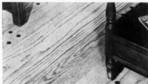
RANDOM WIDTH and walnut pegs are features of plank oak floors by various manufacturers.
