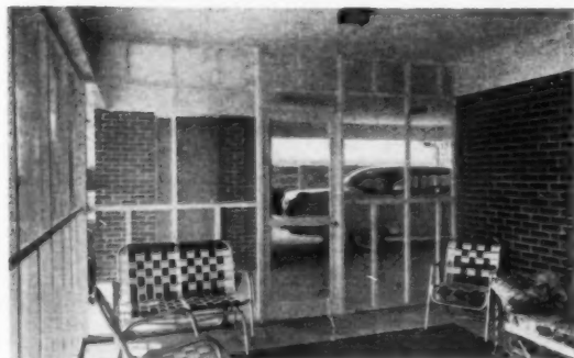
SCREENED PORCH is one of homey features of Better Homes and Gardens Idea house this year (see plan, p. 85). View shows accessibility of carport. Family-kitchen is entered off right. C. T. Donaldson, Montgomery.
