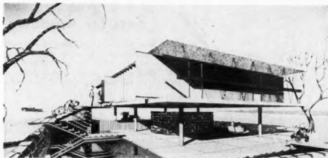
HOUSE ON STILTS is built between two concrete lift slabs. Architect was Robert A. Little.
