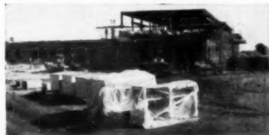
Olin Polyethylene protects materials and machines during wet, rainy periods. Its "see-through" quality makes supplies and equipment easy to locate.
