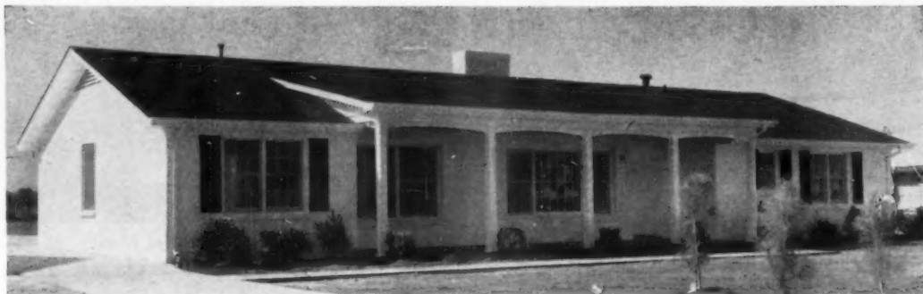
FRONT PORCH , 8' by 32', "recaptures charm of old South combined with modern design," says builder I. D.
