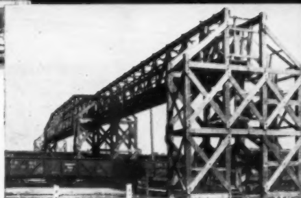
Fabricated timber overpass D & R G Railroad, Denver. Spans are 70' and 170'.
