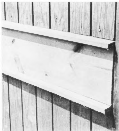
FINISH BOARD , with drip caps top and bottom, covers joints between levels. Without it, siding would have to lap, or else panels would have to run from top of house to bottom, would be too big and heavy to be handled easily.
