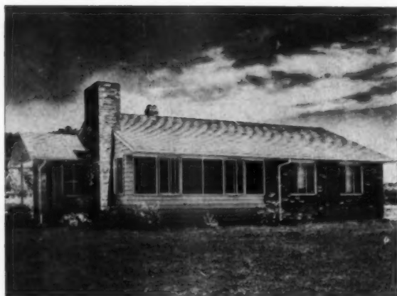
Outstanding feature of this modern home in Washington, D.C. is its window wall—set in frames of steel. Because steel is so strong, it is able to support large areas of glass with slender, inconspicuous frames. Aubinoe, Edwards & Beery, Architects; Aubinoe Construction Co., Builder.
