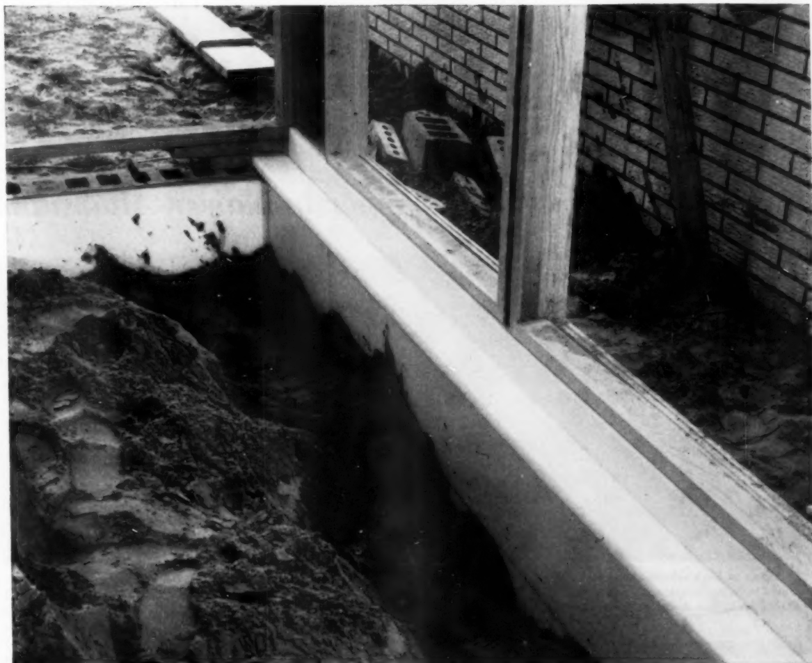
Styrofoam is used for perimeter insulation throughout to assure warm floors, and low heating cost for the life of the house.
