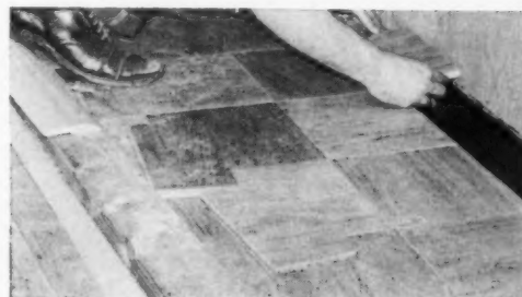
HARDWOOD PLYWOOD 9" squares by Plyfloor fit tongue and groove on mastic. Circle No. 11055.
