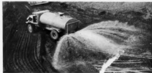
FINAL SETTLING OF FILL is done with water. Rain would do the same thing, but the job can't wait for nature.
