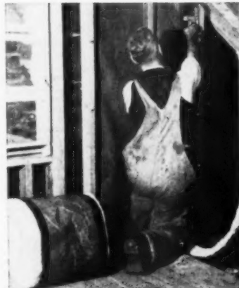
Hansen Tacker tacking insulation—one of many uses in doing a faster, better job, and cutting costs.
