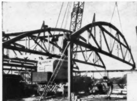
Erecting 100' Rilco Manocord trusses - Big Bear Store, Lincoln Park, Michigan
