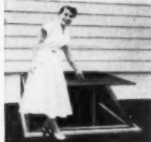
Finger-Tip Operation. Double-acting springs counter-balance the door in any position.
