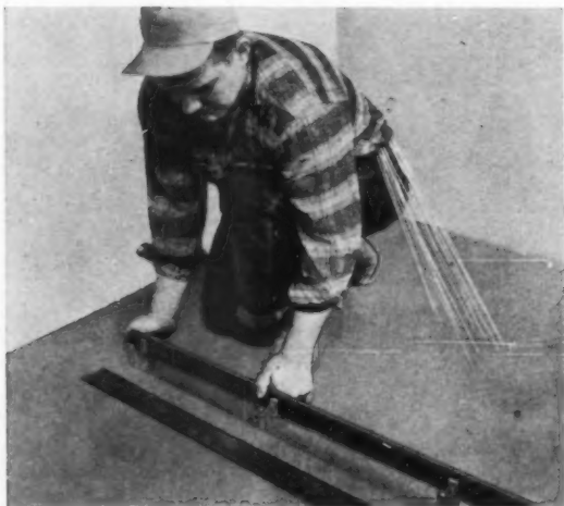
1 Floor runners, with integral base, have clips which are anchored to the floor. In this way, they line up the partition. The side pieces then snap into place and form a channel.
