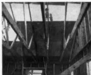
PRE-NOTCHED RAFTERS guarantee extra rigidity and accurate, foursquare interior partitions. Clear span trusses permit builders to vary the plans, since interior partitions carry no weight.
