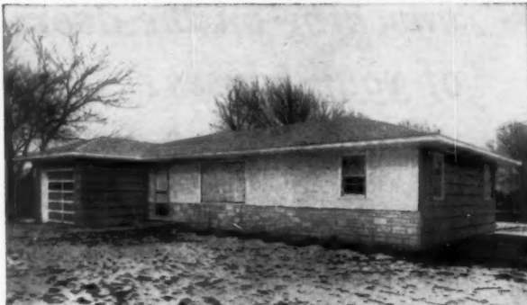
Extremes of climate (hundred-plus in summer, ten-minus in winter) helped the owner-builder decide to equip this Hickman Mills, Missouri home with the C-E Heatmaster System.
