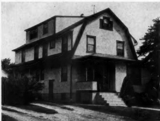
OLD HOUSE: Stucco cottage was purchased by Trade-In Homes, Inc., Baltimore, Md., for $16,000 in trade for new house (right).
