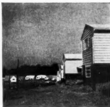
A small section of J. C. Conley's Riverdale Woods. This 134-house development in Riverdale, Md., just east of Washington, D. C., uses steel windows throughout, including big ranch windows.
