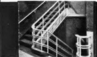
Railings made of aluminum stand up under the hardest kind of treatment.
