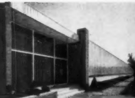
Curtain walls made of aluminum eliminate maintenance costs due to constant exposure.
