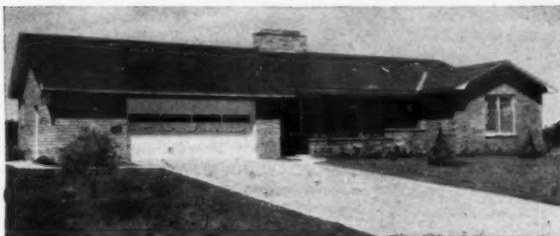
Ranch-house architecture is at its best when Vibrapac Block are used.
