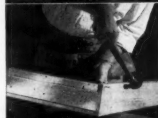
Adjustable Kenna-pak is nailed flush with side jambs.
