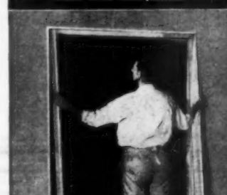
One man raises Kenna-pak and jambs into place.
