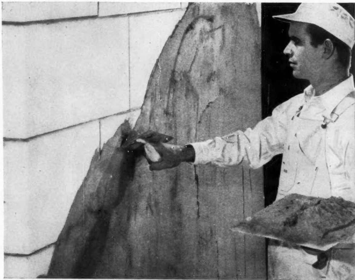
Plaster keys directly to Styrofoam without need for lurring or lathing. Acts in same capacity as plasterboard but gives added advantages of great strength and high insulation value.
