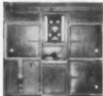
Refrigerators above, loading counter between. Freezer and storage below.
