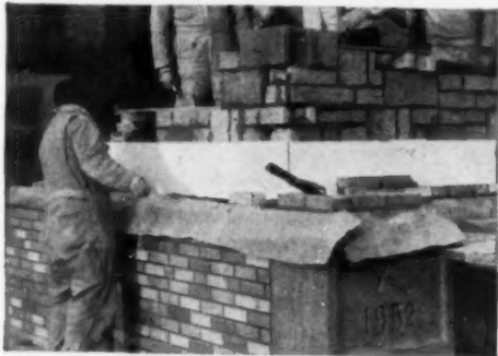
Cavity Walls —Styrofoam proves completely satisfactory as cavity wall insulation for light or heavy construction.
