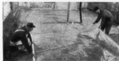
Ideal for slab, full cellar, or crawl space construction, light, tough Olin Polyethylene makes a permanent moisture barrier. Comes in extra wide roll widths for additional time-saving.
