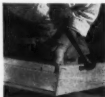
Adjustable Kenna-pak is nailed flush with side jambs
