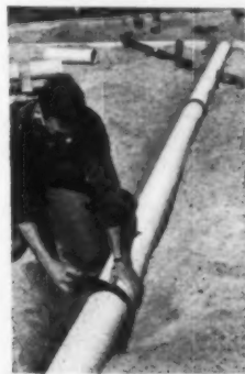
Taped joints easy to make.
