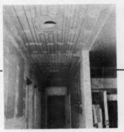
HEAT CABLES in the ceiling provide electric radiant heat for the hallway. They are only one segment of the house's system. Wall thermostat, connected to outside thermostat, and the master control are also located here. Besides the hall, the family room, kitchen and living room are warmed by ceiling units. Other heat applications are found in the three bedrooms which have baseboard units. For quick concentrated warmth, the baths have wall heaters.
