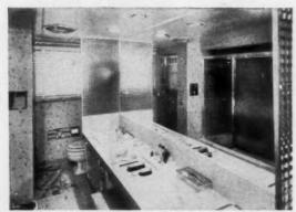
HEATING PLUS LIGHT for this bathroom comes from Nutone's Heat-a-Lite installed in ceiling over the vanitory area. Builder Ray Nelson of Cincinnati, Ohio, also includes a Nutone ceiling ventilating fan as part of his bathroom package. Nutone Inc., Dept. AB, Madison and Red Bank Rds., Cincinnati 27, Ohio. (No. 5013, p. 132.)
