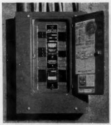
MAIN PANEL, 125-amp-rated split-bus type, shows 1¼" rigid conduit bringing three #3 RH service conductors from weatherhead. Promotion emphasized 2,400-watt kitchen split-circuits.
