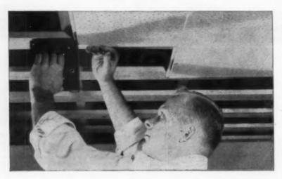
In one fast installation, Cushiontone provides modern Sound-Conditioning and a beautiful ceiling. Sturdy T & G joint speeds nailing, stapling, or cementing and insures a level ceiling.
