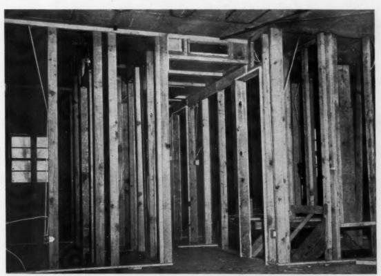
WIRING IS ROUGHED IN and dropped to proper location before outside walls receive insulation and rock lath, and ceiling receives lath and radiant-heating tubes. Room partitions and hall plenum for optional cooling, and
