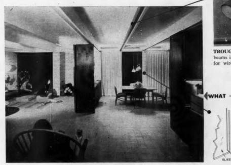
TROUGH in underside of beams is utilized as raceway for wires, switched outlets.
