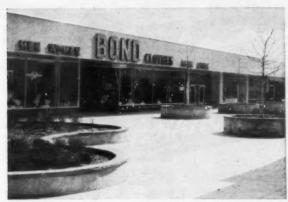
Forty thousand sq. ft. of Weldwood Porc-Lin-Ply were used for fascia of soffits in this shopping center in Valley Stream, N. Y. 1/16" thick panels weigh only 1.75 lbs./sq. ft. Hard, semi-matte finish panels in 9 colors are easily wiped clean.
