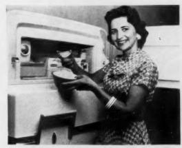
GAS REFRIGERATOR (Servel) produces half-moon shaped pieces of ice which are stored loose in a plastic basket. This eliminates cracking cubes out of trays.
