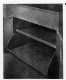
UNDER BUILT-IN RANGE, two large pullout shelves provide convenient storage for pots and pans. Narrower versions are designed for canned goods, every can is easily seen.
