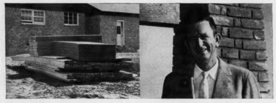
**Stockplies at Job site** need little protection, as Insulite Sheathing comes through any weather safe and sound. Latch takes deliveries in large quantities, drops enough for each house near the foundations.
