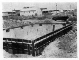
ENGINEERED CONCRETE FORMING equipment can be used and reused for foundations. Average labor on large project for setting, bracing, pouring and stripping was 27-32 man hrs. per basement. Waco (No. S26, p. 150).
