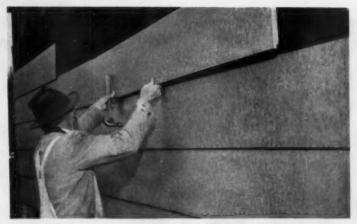
**SELF-ALIGNING**, the siding is easily applied by one man. Rabbeted joints eliminate the necessity of carefully lining up each piece.
