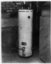
40-GAL. CAPACITY gas hot-water heater amply fills needs of this modern home for personal, clothes and dish washing. Unit is by John Wood.
