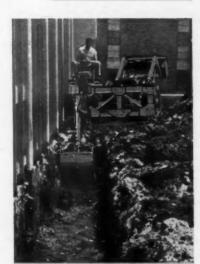
and look what it does! Only the Davis 210 Backhoe can dig flush alongside of a building like this. It has three interchangeable digging positions – from either end or from the center of the frame. It utilizes an exclusive rotory hydroulic boom swing cylinder that provides 200° continuous operating arc.
