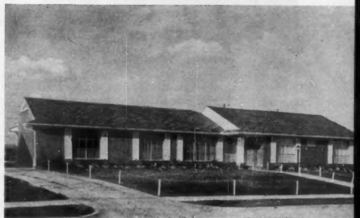
BIG WINDOWS and big shutters create the effect of a house much larger, more costly. Maxwell Construction built it. Cost: $26,000 with land.
