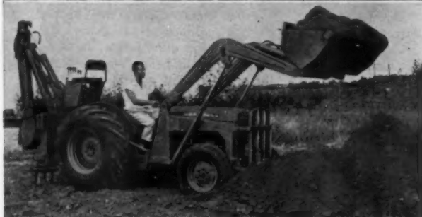
Davis 210 digging flush alongside a building.
