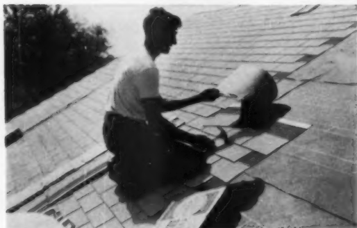
HURRICANE PROTECTION is offered as a "Hidden-Value" prize by Flintkote. Enough Seal-Tab Shingles for a complete roof will go to the winning builder. The shingles have a self-sealing strip on the underside which permits them to bond into a weather-proof roof.
