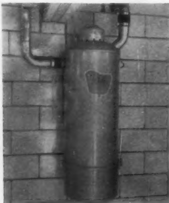
BUILT-IN VACUUM system with 3 or 4 inlet valves is prize donation from H-P Products. Vacu-Flo power unit (above), tubing, fittings are installed in walls. Value: $300.
