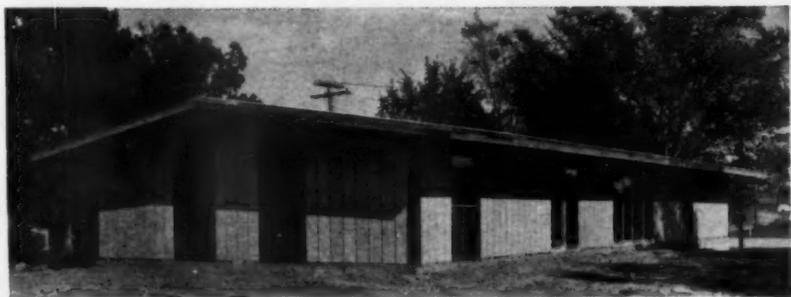
**EXTRA THIN** load-bearing walls of the test house make extra space available inside. Wallboard is nailed to 2x2 furring strips. Finished wall is only 5" thick, less than veneered wall.
