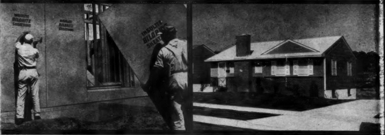
**4' x 9' size avoids “piecing out.”** in vital sill area between foundation and sidewall. One man can easily lift, carry and nail a big, light 4' x 9' Bildrite panel. Applied, it makes a solid, tight, strong insulating shell from eave line to top of foundation.
