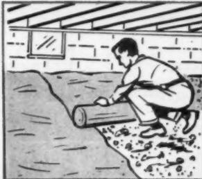
Warp's Polyethylene COVERALL permanently solves moisture vapor problems under houses. Prevents rotting of joists and sills. Also recommended for use between Studdings and Siding, and between Sheeting and Roofing material. COVERALL lasts a lifetime—is inexpensive, comes in various thicknesses and widths to 40 feet, for simple, easy installation.
