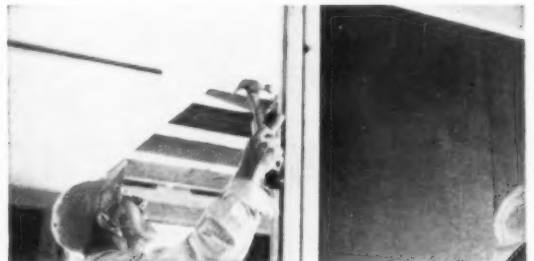
WHAT'S the point of 4" stud walls when they aren't load-bearing? Here's a 2" prefab hollow-core section.
