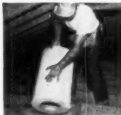
One man can install a Van-Packer in 3 hours—saves on labor costs.
