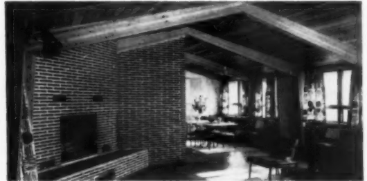
HERE'S a new entry in the home building field—glue-laminated beams. Few codes even consider them.
