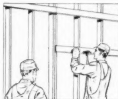
Hummer System reduces cost of laminated construction by using strips in place of full sheets for back layer.
