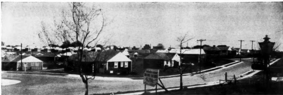
PARTIAL VIEW of Rockledge Homes, Abington Township, Penna. All 106 homes have Anaconda copper tube sanitary drainage lines.
