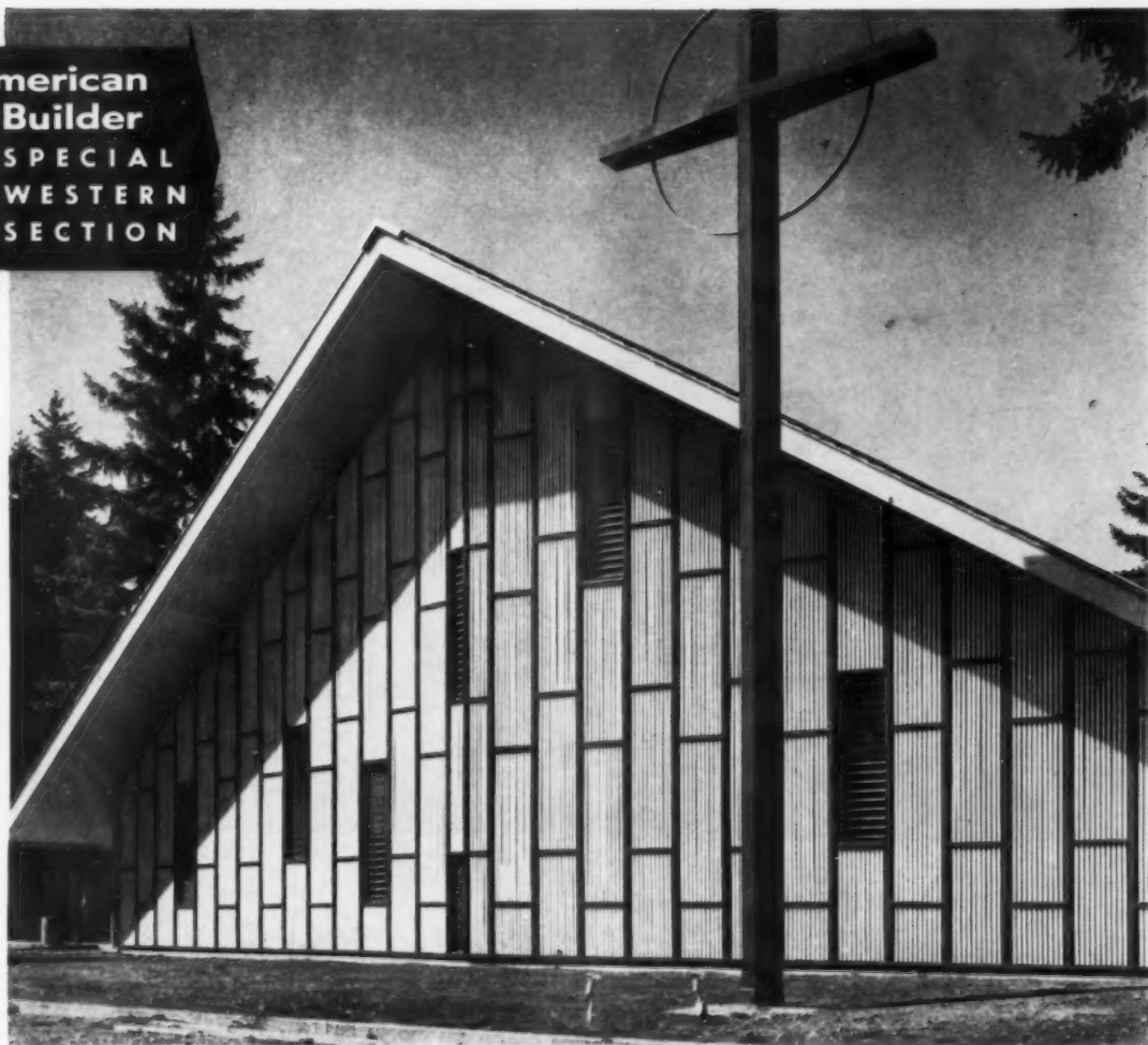
GABLE WALL is of glass. Vertical slats diffuse light. Cross is made of glued laminated beams and copper ring.
