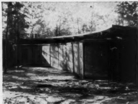
LANAI is formed between continuous curve of screening and house's facade, made of sliding glass doors.
