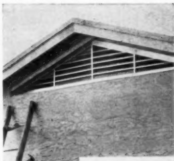
NEED for proper venting when an attic fan is installed is a must. Here's a new unit from Louver Mfg. & Supply; 4-12' lengths. (No. M37, p. 114).
