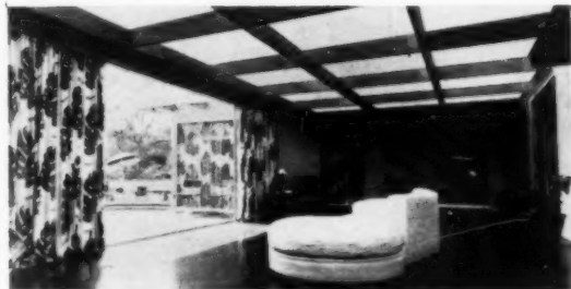
FIBER GLASS reinforced plastic panels are finding many new uses in the home—where good codes permit it.
