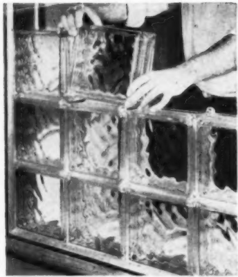
SPACE-DIVIDING interior glass panels are now easier to construct. Owens-Illinois' glass blocks can be bolted together without use of mortar. (No. M19, p. 114).
