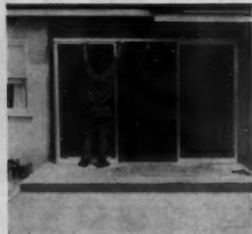
FRAMING IS SIMPLE , one man job. Placement of glass panels completes transformation.
