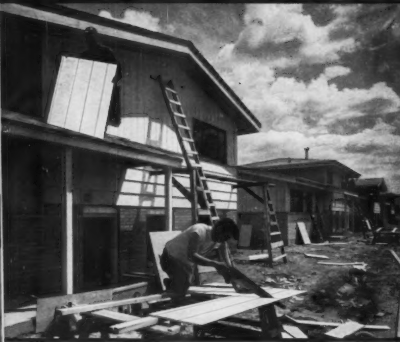
Speedy application of Insulite Primed Siding—both horizontal boards and vertical grooved panels—is seen in recent photo above, made at new Lincolnwood area of Park Forest.
