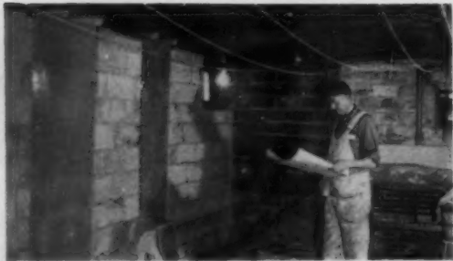
ON block walls toggle-bolt fasteners were used . . .
