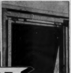
ATTACH HARDWARE AND HANG DOOR
