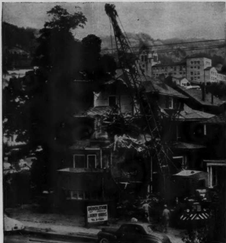
Harris' patented demolition bucket makes short work of this wrecking job.
