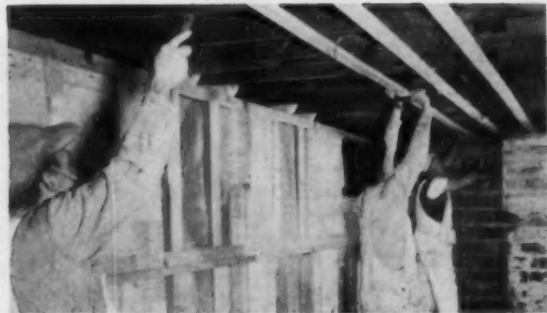
. . . to hold furring. Ceiling strips were nailed to joists.
