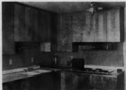
ONLY FINISHED TRIM showing on final job is the doors. Cutting block, center, covers hole in the corner.
