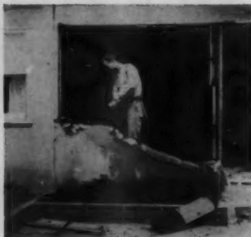
REMOVAL OF WALL is accomplished to accept Hi-Lo "floating" glass door.
