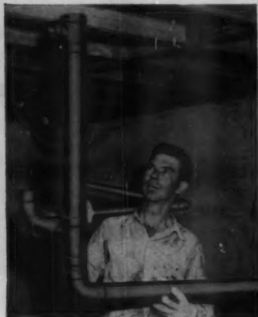
Lightweight tube and fittings make possible time-saving preassembly sections which are easily handled and can be readily put in place.
