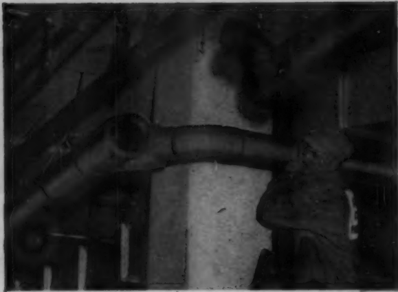
Typical of the larger Anaconda cast-brass drainage fittings is this 8" to 6" Y-branch, being installed in the soil line of a large hospital.
