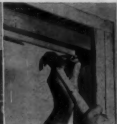
NAIL HEADER TO JAMB
