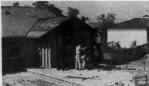
FOUNDATION, subfloor are in. Gable ridge . . .
