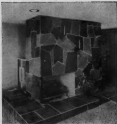
UPPER LEVEL of two-level poured-concrete fireplace. Hearth rests on floor. Fireplace separates stairwell from living area.
