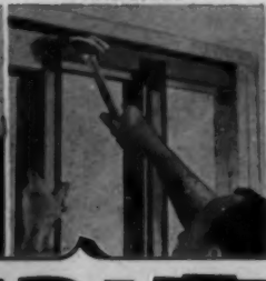
ERECT SPLIT JAMBS AND STUDS
