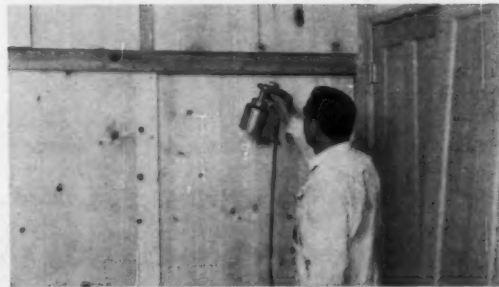
. . . which is sealed, then glazed in a gray tone.
