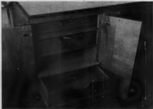
SAME PIECE is used for shelf or drawer bottom. Thus builder can offer any combination of shelves and drawers.
