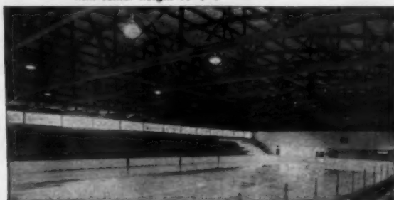
Ice-skating rink, Bowdoin college, Brunswick, Maine Rilco Monocord trusses span 138' 4", spaced 14' o.c. with center height 19' 7".
