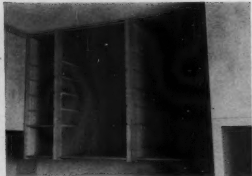
INDIVIDUAL CABINETS are mounted next to each other in any desired order. Doors are only remaining step.
