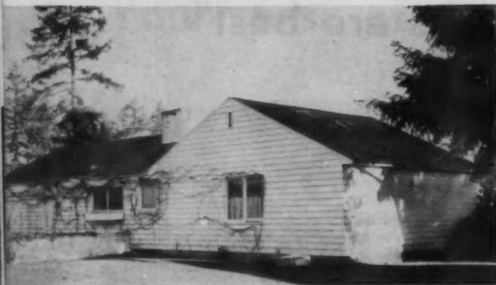
BEFORE: From the rear, the bedroom where addition went on. ▲
