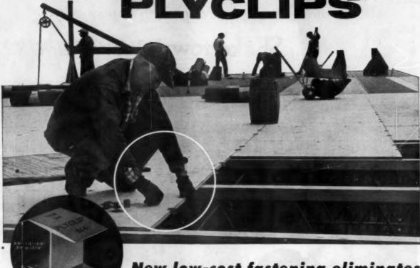
New low-cost fastening eliminates blocking on fir plywood roof decks
