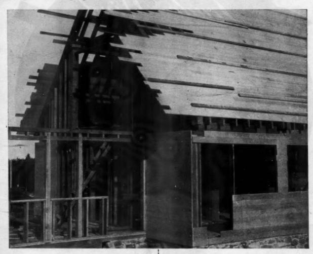
ENGELMANN SPRUCE not only gives you a lightweight wood for easy handling on the job site, but also combines strength plus the ability to be easily nailed without splitting. For sheathing, subflooring and roof decking, its insulation value is high—an important consideration for residential properties. Its strength is frequently well suited for studding, joists and other construction uses.
