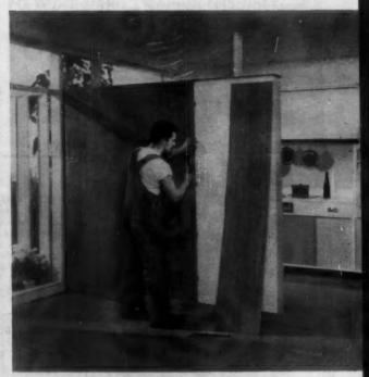
WOOD TEXTURED, plastic finished wall panels are hard, yet flexible. Soil-proof, moisture-proof finish makes them time and money savers. Panels are easy to cut and install. Marsh Wall Products. (No. S77, p. 150.)
