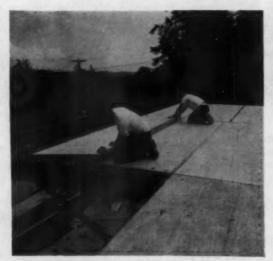
DUAL-PURPOSE 4x12' panels roof the house. They provide roof decking and ceiling in one component. Each panel consists of fir plywood top and bottom skins glued to lumber framing members. Insulation is sandwiched in between.
