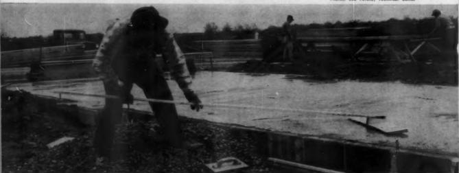
POURING center bearing footing and slab monolithically saves four courses of block.
