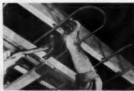
PG's save time. Anaconda Panel Grids are easily lifted and propped in place, leaving worker's hands free to fasten tube straps. Metal lath will be installed below the grids.
