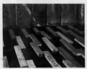
2 Lay screeds at right angles to proposed direction of flooring, 12" on centers with ends lapped 4". Staggered pattern helps to provide good nailing surface.
