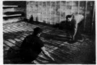
Heat for this basement game room will be provided by ½" PG's embedded in a concrete slab. For floor or ceiling radiant panel heating systems, Anaconda PG's offer many installation economies. 5815
