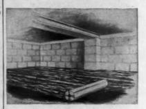
In basementless homes, the simple, lowcost way to protect crawl space is to spread DURETHENE polyethylene film on the ground and then cover it with a heavy layer of dirt. This provides a permanent moisture barrier and prevents serious dry-rot damage to plates, sills, joists and sub-flooring.
