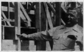
"YOU CAN SAVE \$60 per house balloon framing your splits," says Harry Lubell. "We've tried it both ways. Balloon framing is better all-around construction. Once partitions with ledger boards are in place: unskilled labor does the rest."
