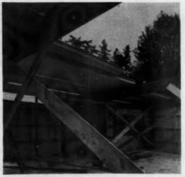
CANTILEVERED beams finished in redwood support the roof. Panels similar to the roof made the floor of the second story and ceiling of the first. Cost: 75¢ a sq. ft. for roof—90¢ for floor (including fabrication and installation).
