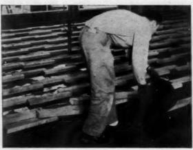
Apply surface moisture barrier to slab and lay flat, dry, preservative-treated 2 x 4 wood screeds in hot mastic. Use random length screeds, 18" to 30".
