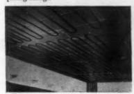
Ceiling installation on gypsum lath. Note changes in spacings-4½" centers near the outside walls where heat loss is greatest but with the c-c spacing in-creased at the center and inside areas.
