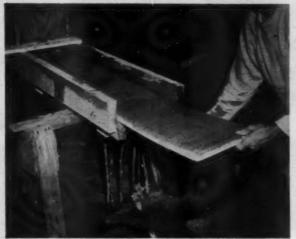
"STYROFOAM bonds readily to the interior masonry surface. A uniform layer of cement mortar is applied by running the  $1^{\prime}$  x  $9^{\prime}$  boards through a coating trough."
