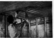
Hook-type fasteners of nonrusting Everdur, also offering easy, fast instal lation, are partially set in joists-PG's slip over hooks. Fasteners are driven to draw tube to ceiling.
