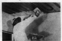
No sags or dips in the tube lines. PG's are uniform and fasten snugly to ceiling construction permitting a uniform thickness of plaster with resulting savings in materials and time.
