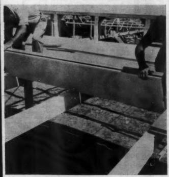
ROOF DECKING is installed quickly and economically. Panels eliminate need for ceiling joist. Fewer roof beams are required as decking spans 32" and 48" instead of 16". Simpson Logging Co. (No. S76, p. 150.)
