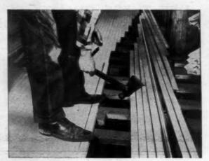
Blind nail tongued-and-grooved, end-matched strip oak flooring at each screed intersection. Double-nail at lapped screeds. Finished floor is beautiful and durable.
