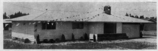
L-SHAPED house has composition roof, horizontal siding. Chimney is prefabricated by Metalbestos.
