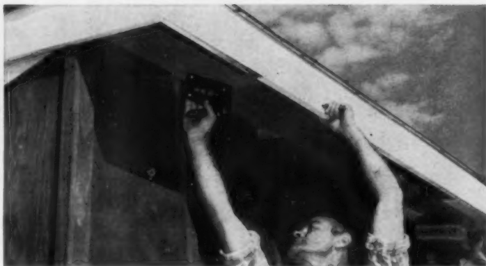
ONE BLOW of hand stapler places and drives staple home, freeing other hand to position work. Tool above is in wide use installing tile, insulation.
