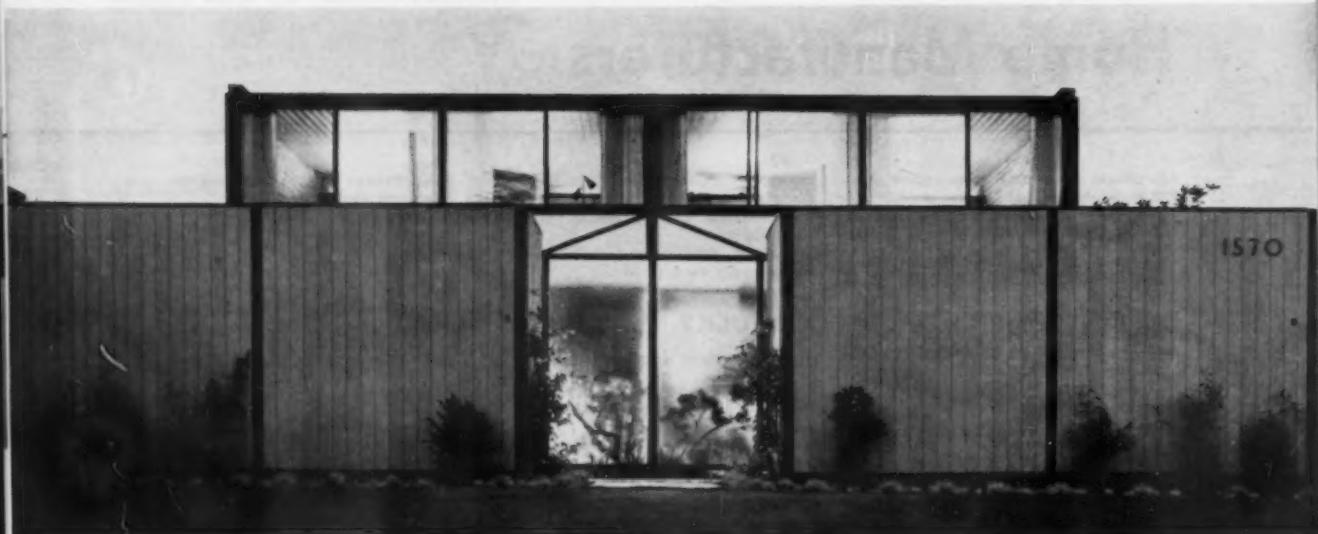
High fence of fir siding and obscure glass panels provide privacy to courtyard entry.
