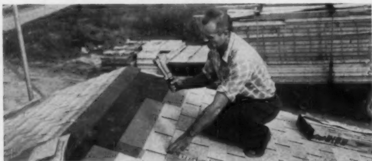
ONE BLOW of hand stapler places and drives staple home, freeing other hand to position work. Tool above is in wide use installing tile, insulation.
