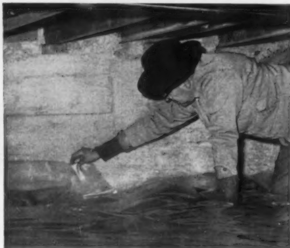
IN CRAWL SPACES—VISQUEEN film banishes musty odors, keeps earth-born moisture away from floor joists.
