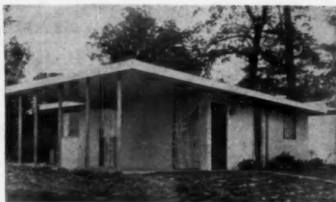
ALCOA "ALUMALORE," a baked alkyd, is outside wall finish. Roof finish is simply untreated aluminum.
