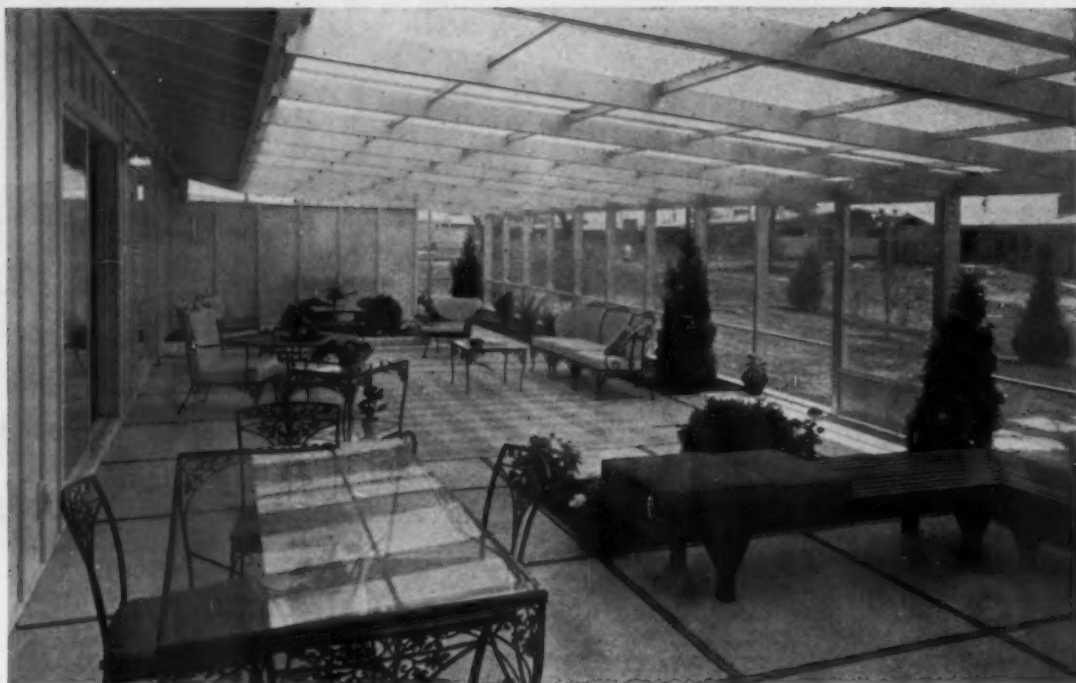
NEW CONCEPT in outdoor living is this terrace room across the rear of the house. Corrugated roofing is made of Fiberglas. Sides of the terrace are completely screened.
