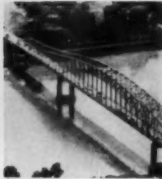
MISSOURI RIVER BRIDGE St. Charles, Mo.
