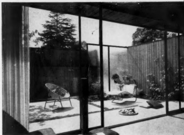
INDOOR-OUTDOOR living is achieved with Miller steel-framed sliding-glass door units and glass wall units of ceiling height. View, here, is from inside. Wall units fasten directly to undersides of joists.
