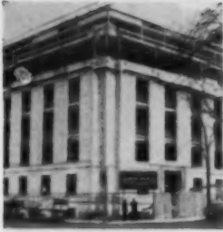
NEW SENATE OFFICE BUILDING Washington, D. C.
