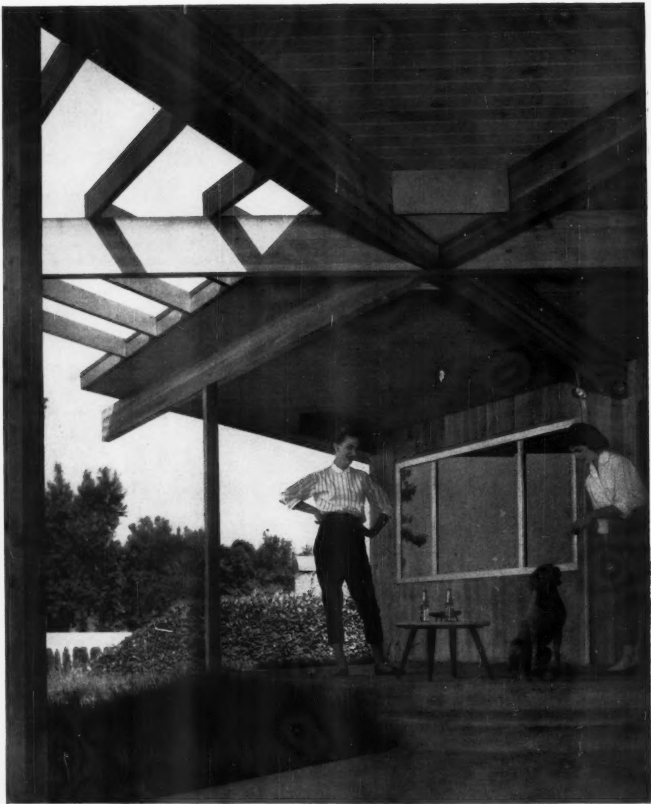
Strong selling point of this home is a roofed-over patio featuring laminated wood beams continued from inside the house. Beams support extended roof and, with roof decking, are stained to match siding. Open section adds light and interest.
