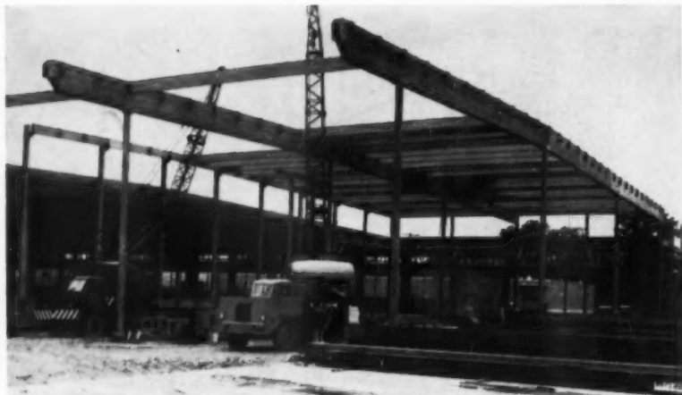
Above, carton plant, Kieckhefer-Eddy Division, Closter, N. J. Constructed with Rilco glued laminated wood beams and purlins in sizes up to 11" x 45½" x 68'¾". Below is completed building. Contractor: S. S. Jacobs Co., Jacksonville, Fla.
