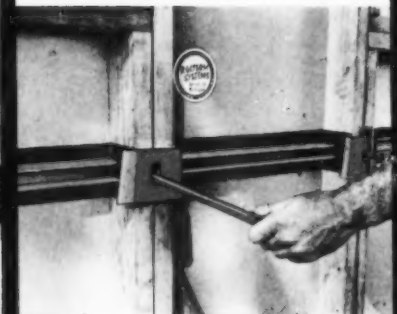
Rocform tapered tie-rod is inserted through clamp and into clamp on opposite wall form.
