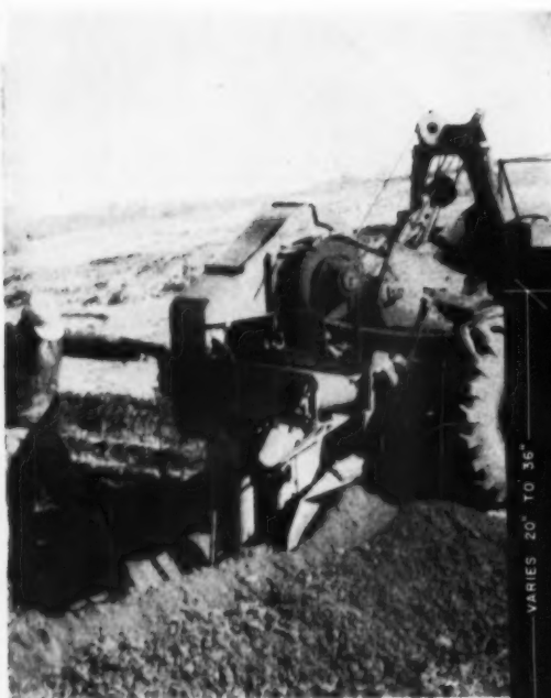
DITCHER RIG DIGS —Combination rig simultaneously digs trench 3 ft. deep and carves bell-shaped footing into fill.
