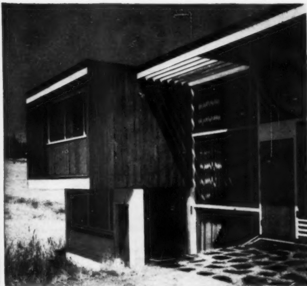
This Massachusetts home uses butt vertical siding in keeping with dramatically simple lines of its design. Flush doors pick up lines and shading of siding. Notice how overhangs protect all windows. Architects: D. H. and M. K. Hunter.
