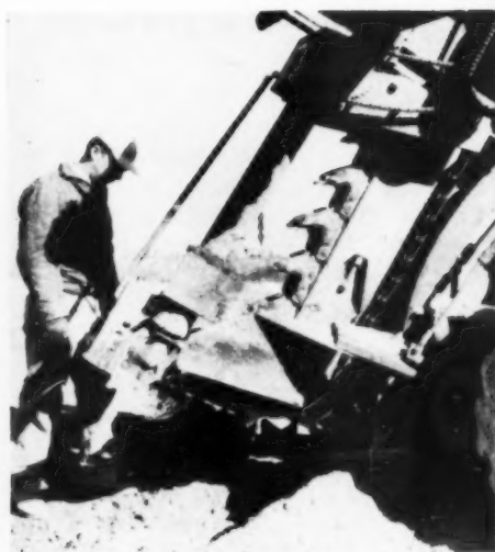
THEN MOVES CLEAR —Once rig reaches corner stake its cutters are raised and the machine is turned to dig along a new length of trench.
