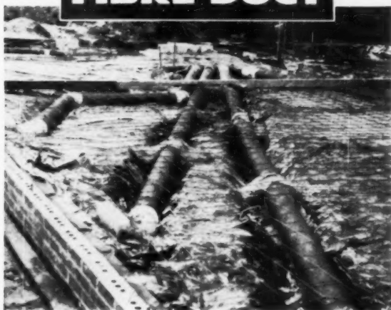
Residence, Hartsville, S.C. Heating Contractor, Kent Hungerpillar
