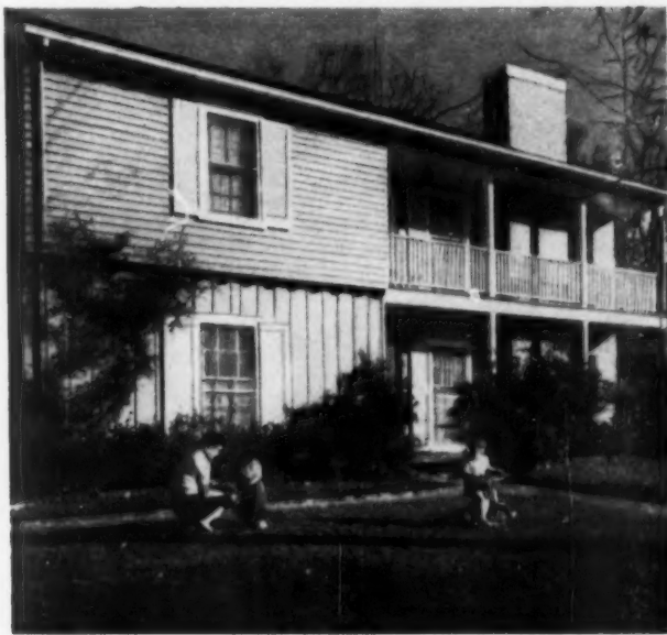
On this handsome traditional home, horizontal bevel siding is combined with vertical board-and-batten siding for a novel effect. Here elements are painted in the same color for visual unity. Architect: Favrot, Reed, Mathes and Bergman.
