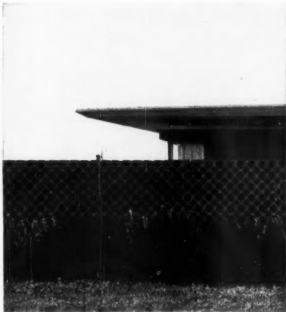
FORMING umbrella-shaped roof takes 4 men only one day. Removing forms takes half a day. Lumber can run wild over edges to eliminate cutting.
