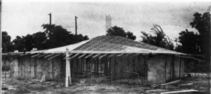
FORMING umbrella-shaped roof takes 4 men only one day. Removing forms takes half a day. Lumber can run wild over edges to eliminate cutting.
