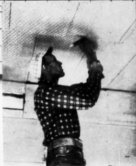
▲ THIRD LATHS —Man staples lath to Dow Styrofoam insulation board on ceiling to ready it for plaster crews.
