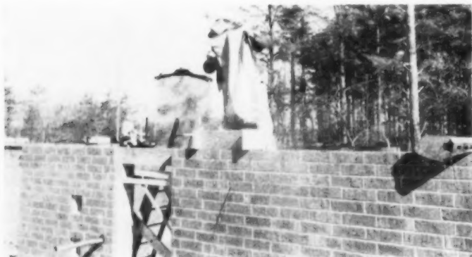
NEW 8x8" TILE-LITES (base of wall, above) promise to be the least expensive way to install lights or windows in a masonry wall. They don't increase cooling load. Cavity walls were insulated with a pour-in vermiculite called Zonolite Water-Repellent Fill (below).
