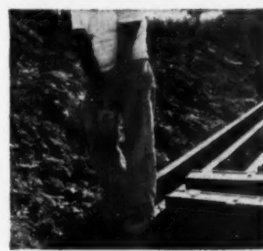
4. Concrete consolidated in side forms with Stow DU midget vibrator.
