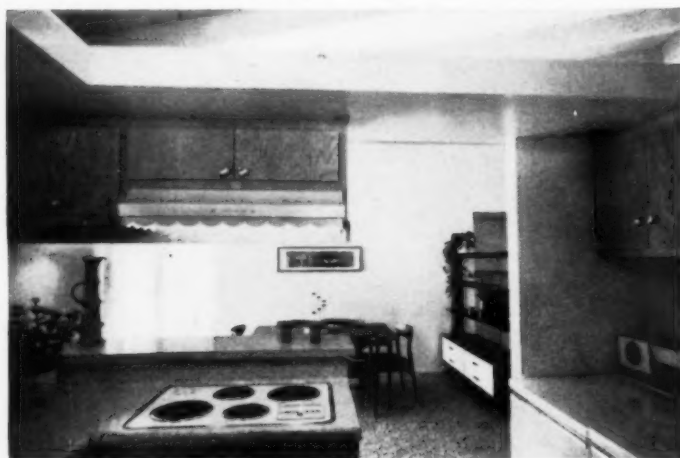
VIEW FROM THE KITCHEN back into the family room shows that instead of being dropped across the whole room, ceiling is simply a soffit running around the perimeter. This combines a high, open effect in the kitchen with good family room/kitchen separation, also supports cabinets.
