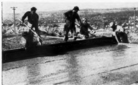
2. 4-inch slump concrete is screeded. Note the termite shield at edge of slab.
