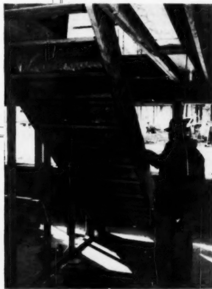
COMPONENT STAIRS come to site covered with protective paper. Positioning them requires little site work. To get lowest prices, Bennett buys components in quantity (5 or more).
