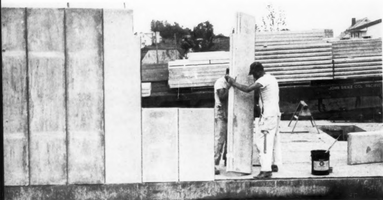
CALSI-CRETE PANELS are set up to form one wall of a house. Drawings show how they are joined and trimmed.
