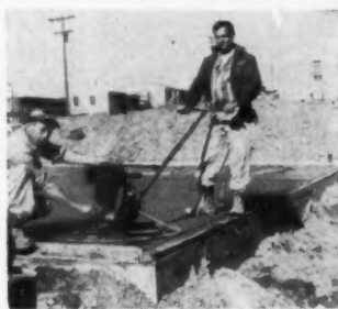
3. 1 1/2 to 2 hours after screeding, Stow G-42 Roto-Trowel used to float and finish floors.
