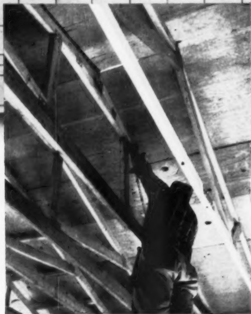
◀ FOURTH CHECKS TRUSSES —Trusses at end of house are redesigned to save space by permitting suspension of utility equipment.
