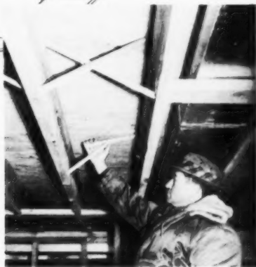
COMPONENT METAL BRIDGING , demonstrated by Bennett's superintendent, is adjustable, requires no cutting. It's merely snapped into place as shown here.
