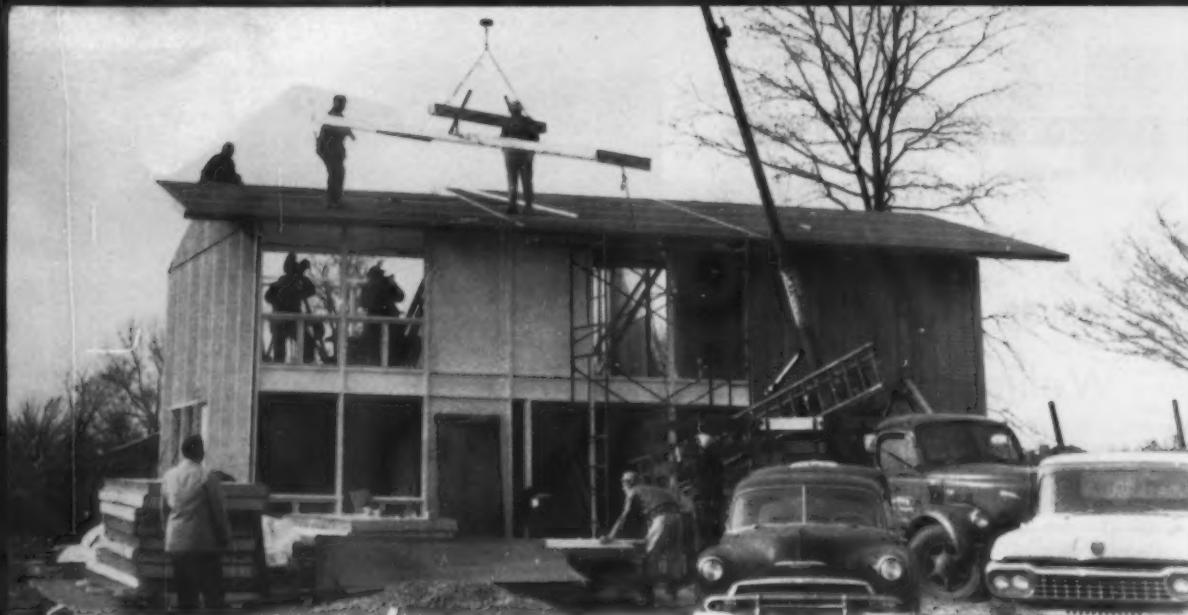
SHELL OF THE RESEARCH HOUSE is shown here being closed in. Roof panel is lifted into position by a light sign-hanger's crane. Wall panels were built as two-
