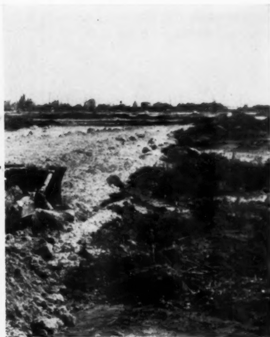
GRID ROLLERS COMPACT EACH EMBANKMENT LIFT —Tractor-drawn Hyster No. 3 grid roller with ballast added passes over each lift to bring it to 95% modified compaction. Each lift gets identical treatment.
