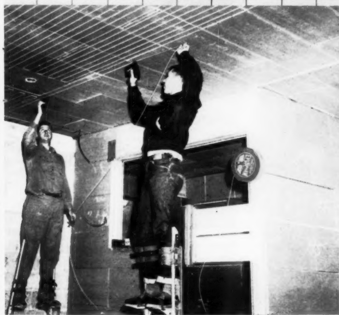
◀ SIXTH CLOSES CEILING —Workmen atop stilts apply Ceil-Heat wiring to ceiling. Heating method helps sell houses in area with limited cold seasons.
