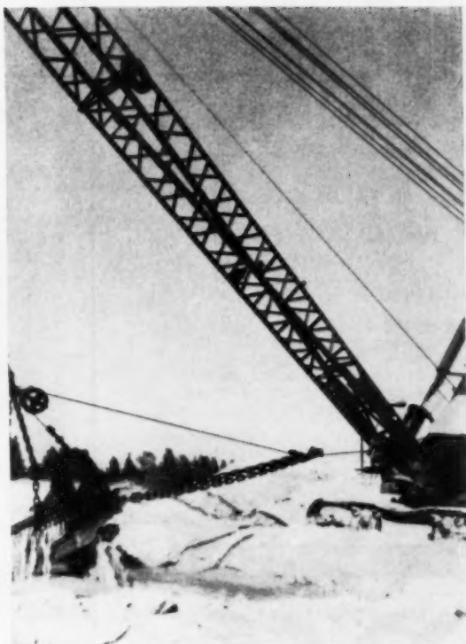
DRAGLINE BORROWS LIMESTONE FILL —Blasting crews first fracture rock in 30-ft. lifts in limestone borrow pit. Dragline with 2½-yd. bucket scoops rock from pit and loads it into scrapers.
