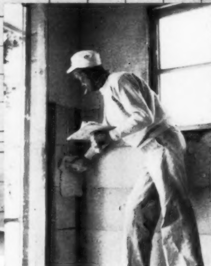
▲ FIFTH PLASTERS —Brown and finish plaster coats are applied directly over Styrofoam that is tacked to studs. Painting finishes job.
