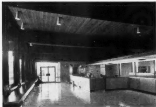
SECTION of main banking room illustrates use of glue-lam Douglas Fir beams and Western red cedar deck. A combination of fluorescent and incandescent lighting is used.
