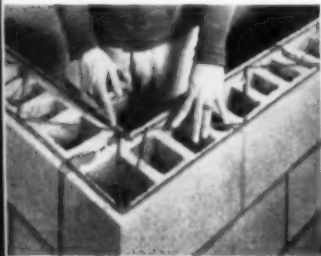
Two engineered products that meet a need. Dur-o-wal reinforcement, shown at left, and Rapid Control Joint, right. Weatherproof neoprene flanges on the latter flex with the joint, simplify the caulking problem.
