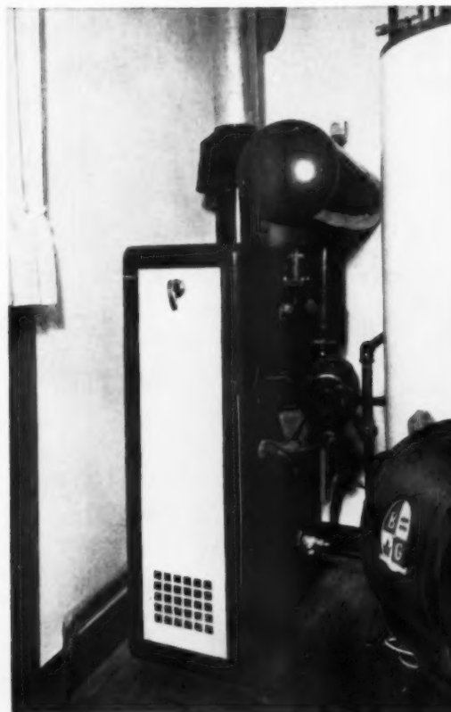
Photo shows small space required by a B&G Hydro-Flo System. The boiler can be installed at any level within a building.
