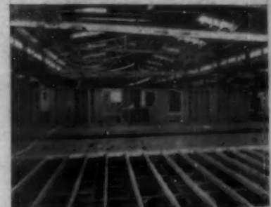
House moves sidewise on assembly line
