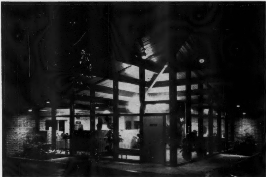
SMALL BANK, designed by architect Clive Kienle, was planned to attract passing motorists—day or night.
