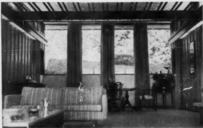
VOLK RESIDENCE, Smoke Rise, N. J. All exterior window walls were constructed of shop-built, prefabricated modular frames, all dimensioned around standard Thermopane sizes. These same panel types, which were fitted into the modular wood framing system, together forming the structural wall and exterior and interior finish, accommodate standard steel sash, blank opaque walls, French doors and regularly hinged doors.
