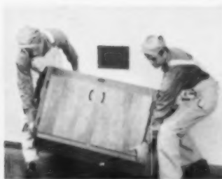
11:05—base cabinet in place
