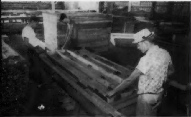
TO CUT COSTS , shops generally use "unskilled" labor with carpenter supervisor. Fett says builder should erect minimum of 3 homes weekly to make own components.
