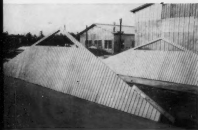
BESIDES TRUSSES and panels, Fett produces gable ends—ready to set in place. Until recently, he was absorbing all component production; now he sells to other builders.
