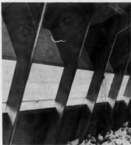
LIGHT AND AIR , as needed in this poultry house, may be admitted by a strip of chicken wire. If necessary, building can be insulated with standard materials.
