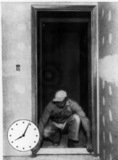
8:04 a.m. Spacer is positioned for parallel alignment of jambs. Overlapping design simplifies installation over drywall. All steel frame eliminates splitting and warping. No call backs.
