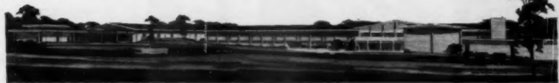
General contractor on the project was Kloster Company. Neal J. Campbell was consulting engineer.
