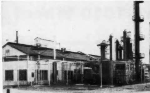
Standby for critical processes in chemical, ceramic, and other manufacturing plants.
