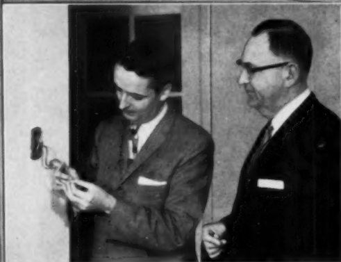
Telephone man Robert Dahill checks position of telephone-wired kitchen outlet with builder Arthur P. Aaron.
