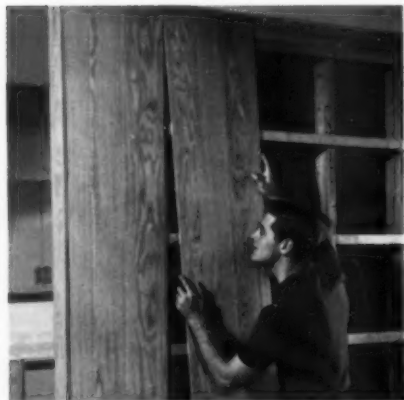
Fast installation. 1/4" thick tongued and grooved Random Planks are 16" by 8" . . . go up with simple clips over furring strips or existing walls.
