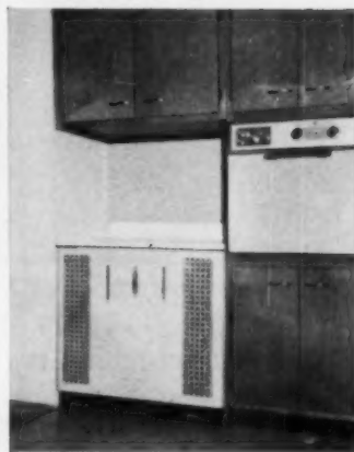
The amazingly compact house heating boiler is concealed behind the grille work of this countertop cabinet, providing added working space in the kitchen. View at left shows a section of development.
