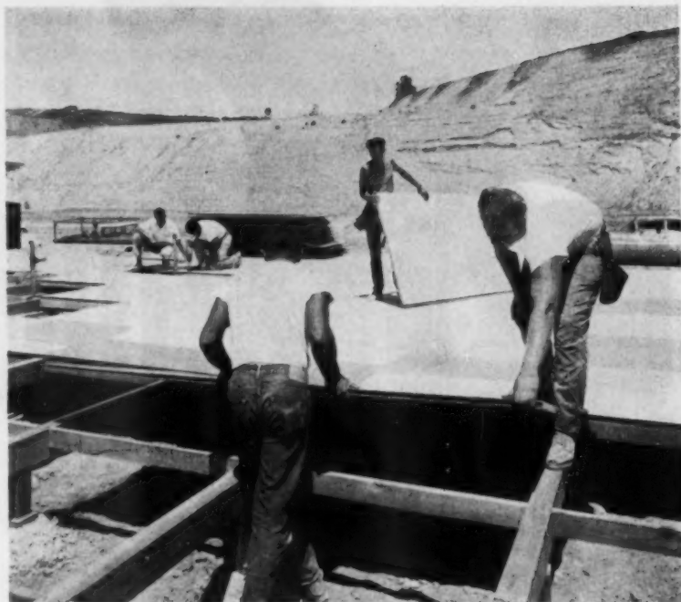
METHOD —Panels are placed as subflooring over girders on 4' centers. Standard panels require at least 2x4" blocking under panels edges—a practice method eliminates.
