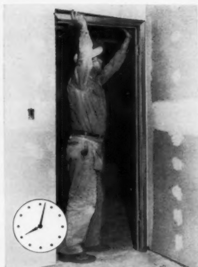
8:02 a.m. Place header in starting position and rotate to horizontal position. Note trim hairline-mitered corner. Provides neat, professionally-finished appearance without on-the-job fitting.
