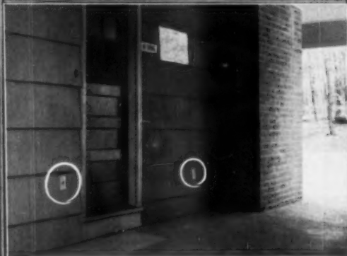
Breezeways of A & A homes come with outlets for permanent or portable telephones.
