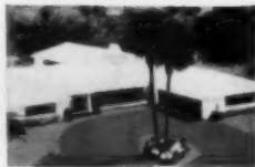
Architect's drawing — Arvida home of Dr. and Mrs. John F. Pearl. Architect: Arthur H. Rude, of Ft. Lauderdale.
