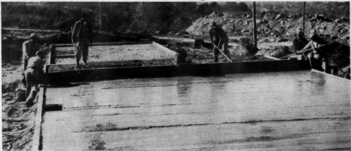
1. Making first pass with 24 ft. 8 in. Stow vibrating screed. 16 man hours per slab saved by Major Building Co.
