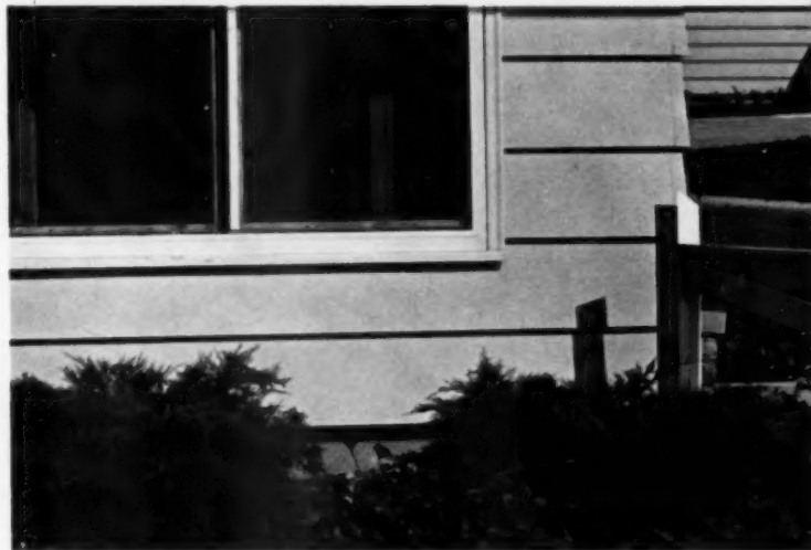
Masonite "X" siding—provides a deep \frac{1}{8} " shadowline—factory-primed.
