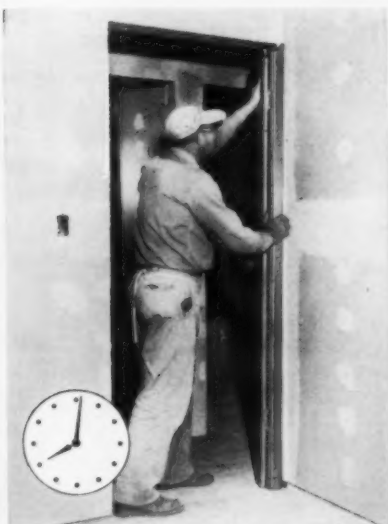
8:01 a.m. Hinge jamb is placed in starting position and rotated to vertical. Lightweight sturdy 22 gauge, rust-resistant steel sections are easy for one man to handle.
