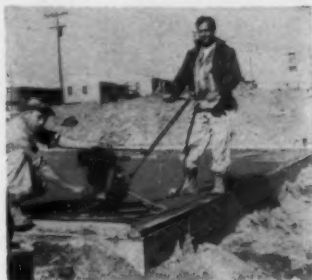
3. 1½ to 2 hours after screeding, Stow G-42 Roto-Trowel used to float and finish floors.
