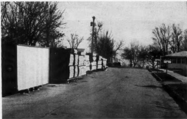
TO SPEED BUILDING production, McFarling puts all materials possible on straddle buggy blocks so it can be quickly moved to building site. Stockpiled here is dimension lumber, casing (in large box), trusses. Van-type trailers are used for tools, materials.
