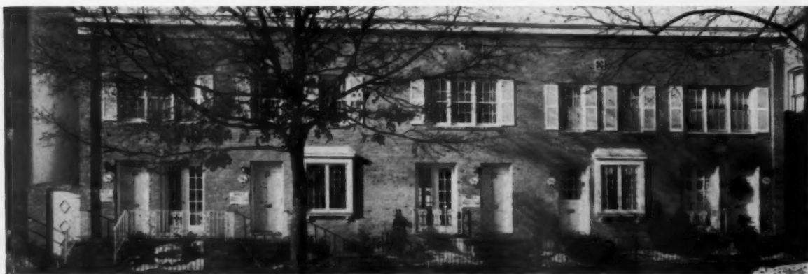
Completely restored rowhouses show builder a 7-8% net profit
