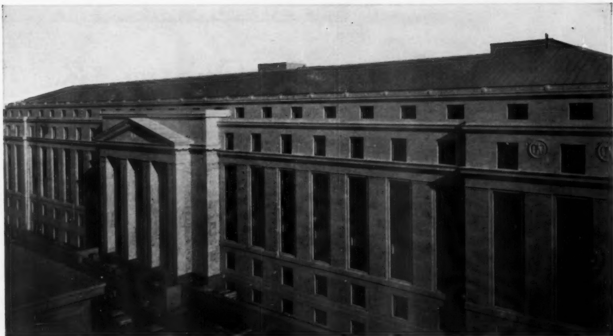
Copper batten seam roofing on the new Senate Office Building, Washington, D. C.
