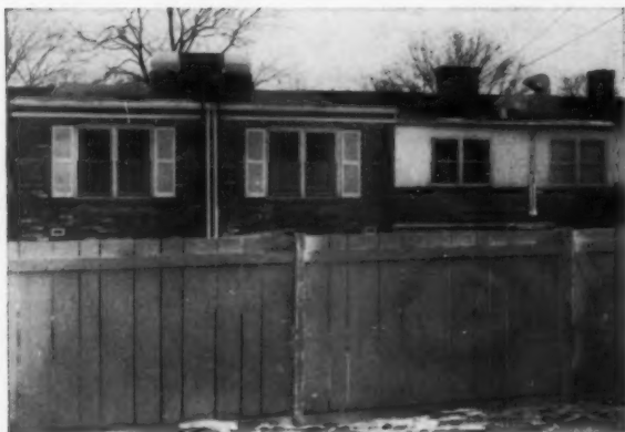
Different elevations leveled off
