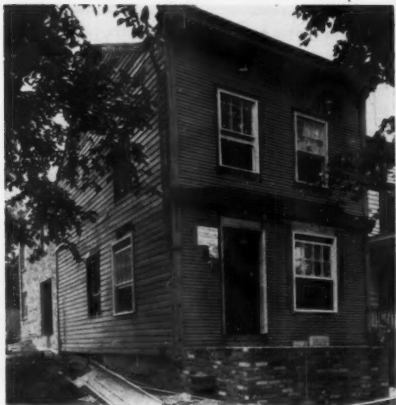
Before—restoring begins on old house
