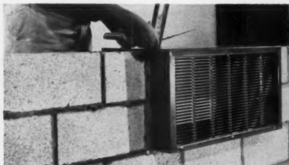
SLEEVE for a/c unit simplifies masonry lay-up. It displaces exactly four concrete block or equivalent even number of brick.
