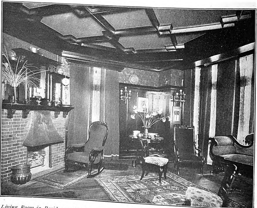
Living Room in Residence of Albert Sutton
