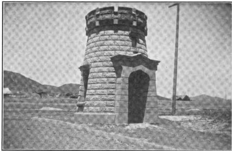
One of Eighteen Towers erected in Hollywood by T. A. McMurtrie from stone made by his latest model machines, capable of adjustment for any size or style of stone.
