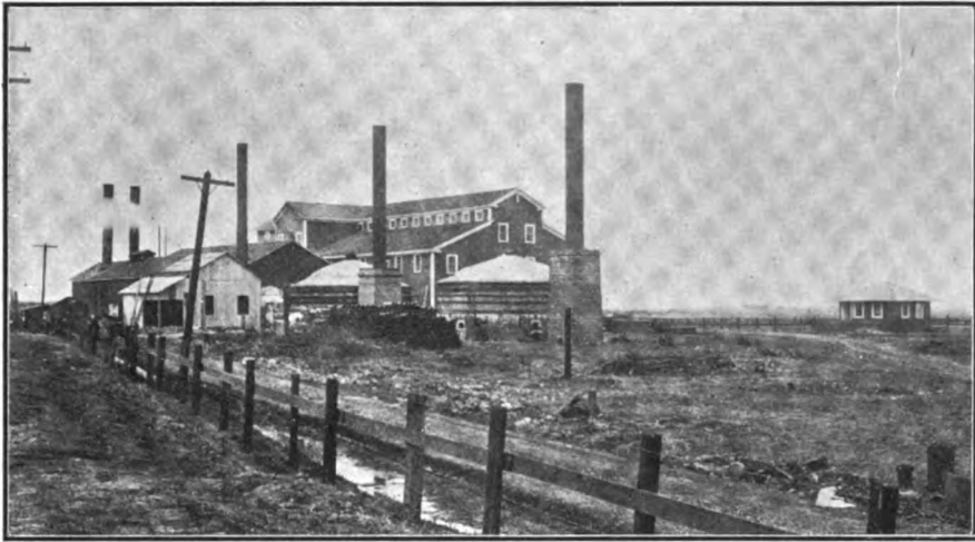
California Brick and Clay Company's New Plant at Antioch, Cal.
