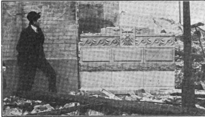
Sample Wall of Concrete Stone which resisted perfectly the heat of San Francisco's big fire
