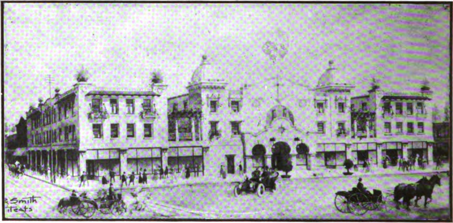
Mission Hotel, Santa Rosa Stone and Smith, Architects
