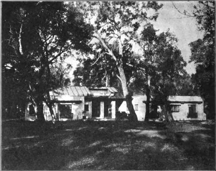
Showing the Possibilities of Reinforced Concrete in Residence Work. Bungalow at Fair Oaks, Cal. Albert Farr, Architect. Richards-Neustadt Co., Contractors
