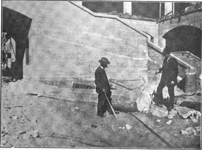
Figure 3. (Note Smooth End of Column)
