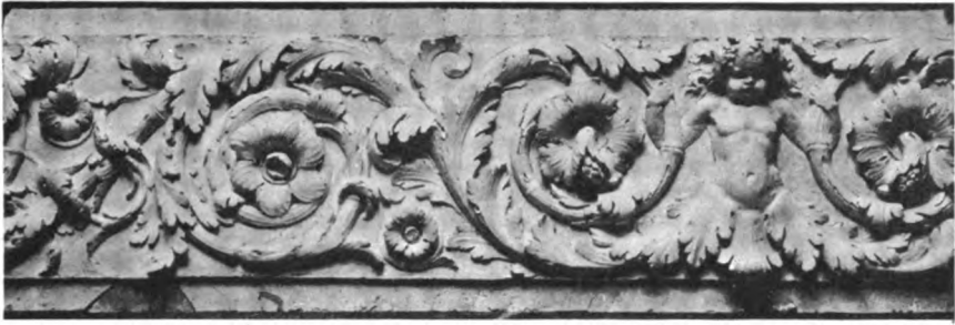
Detail of Ornamental Concrete Stone for Reinforced Concrete Buildings. by O. S. Sarsi.
