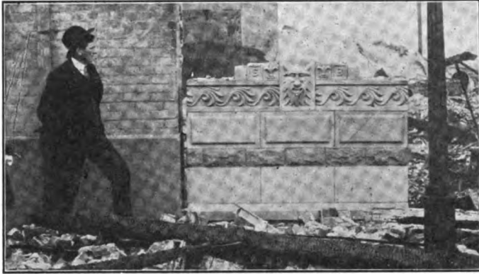
Sample Wall of Concrete Stone which resisted perfectly the heat of San Francisco's big fire
