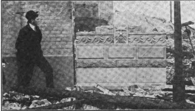
Sample Wall of Concrete Stone which resisted perfectly the heat of San Francisco's big fire
