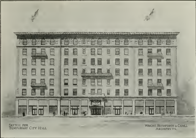
TEMPORARY CITY HALL, SAN FRANCISCO Wright, Rushforth & Cahill, Architects
