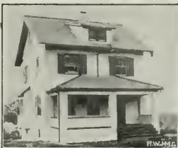
Residence of Mr. Oswald Hessler, Bogota, N. Y., Covered with J-M Asbestos Shingles
