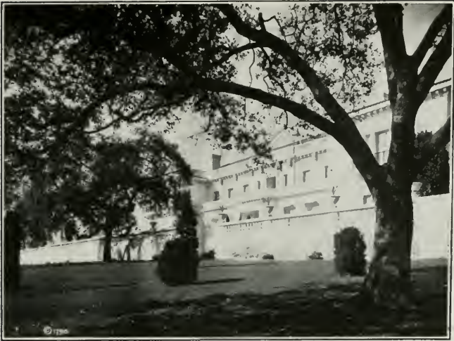
Residence of Henry E. Huntington, Los Angeles Myron Hunt and Elmer Gray, Architects
