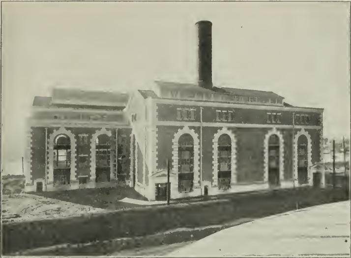
Southern Pacific Company's Power House, Fruitvale, California D. J. Patterson, Architect
