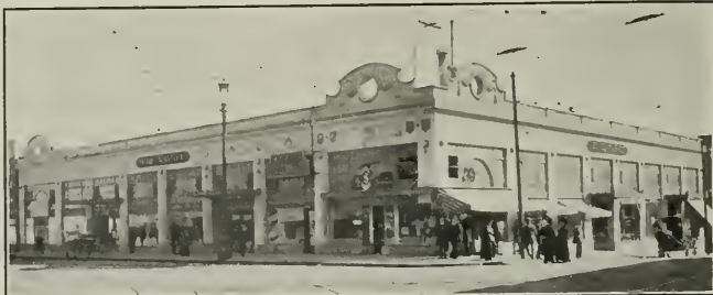
HOME MARKET SAN FRANCISCO. CHAS. S. KAISER, ARCHITECT
