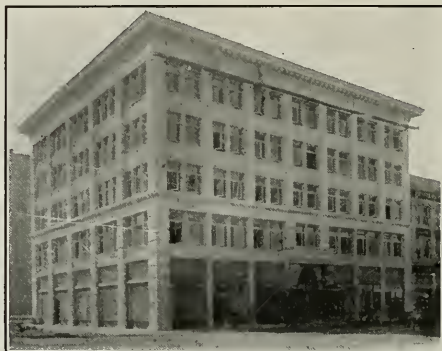
SAUNDERS BUILDING, SAN FRANCISCO
