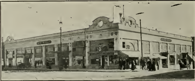
HOME MARKET, SAN FRANCISCO. CHAS. S. KAISER, ARCHITECT
