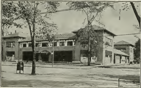
Ferroinclave was used for Roof of this Garage
