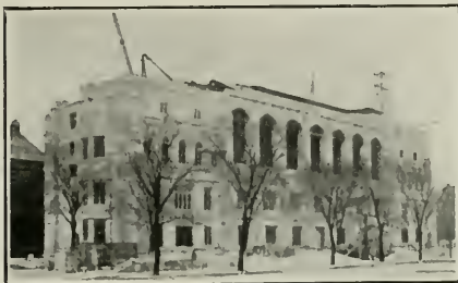
HARPER MEMORIAL LIBRARY, UNIVERSITY OF CHICAGO Waterproofed with CERESIT. A $5000 bond in the National Surety Company was given the contractor, guaranteeing against any dampness for three years.
