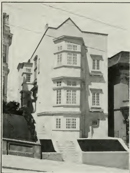
The Same House Showing Pleasing Alterations W. Garden Mitchell, Architect
