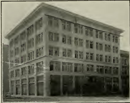
SAUNDERS BUILDING SAN FRANCISCO
