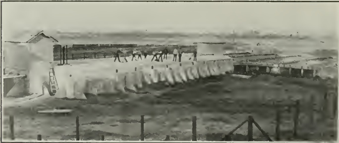
Septic Tank, Santa Clara, California
