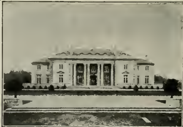
Residence of Alfred I. Dupont Wilmington, Del. 20,000 square feet of NEPONSET Red Rope used here. Architects, Carrere & Hastings.
