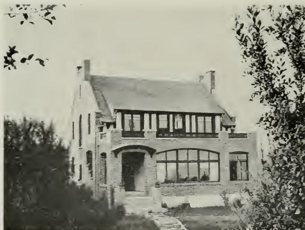
Residence of Clayton L. Wilson, Seattle, Washington Wilson & Lowless, Architects
