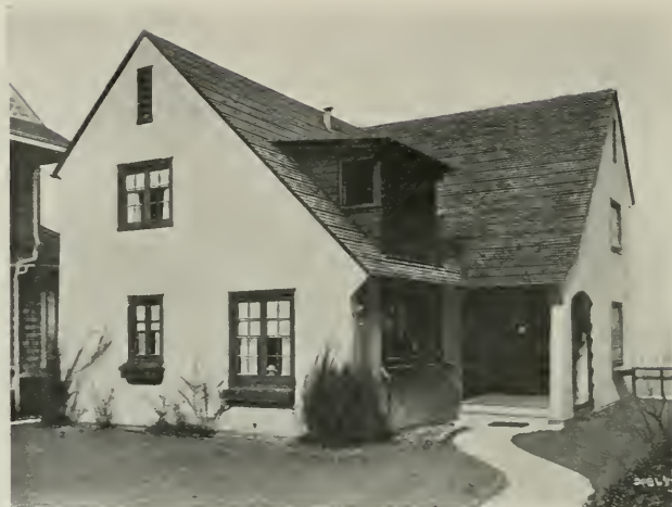
House for H. H. Wolfe, Seattle, Washington Willcox & Sayward, Architects
