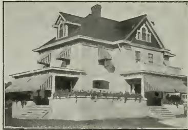
Residence of Geo. D. McIlvaine, Pittsburgh, Roofed with NEPONSET PROSLATE.
