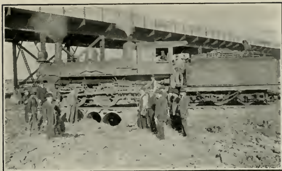
Fig. 2. Chicago Great Western Railroad Uses Ingot Iron Culverts Along its Roadbed
