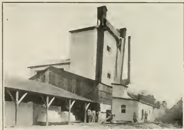
The Sacramento Sandstone Brick Company's Plant on the American River, near Sacramento, California.
