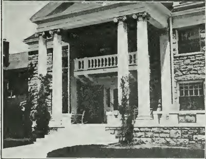
Lower Cut Shows Residence of Wallace Good, Root & Siemens, Architects.
