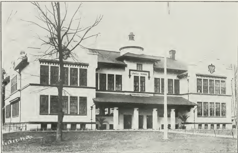
Lowell Grammar School Building, San Jose
