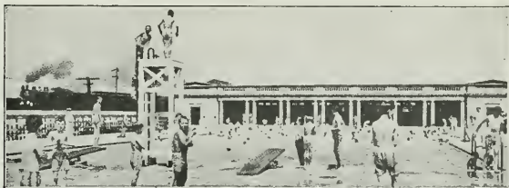
SWIMMING POOL SOUTH PARK COMMISSION, CHICAGO. Waterproofed with CERESIT Waterproofing.
