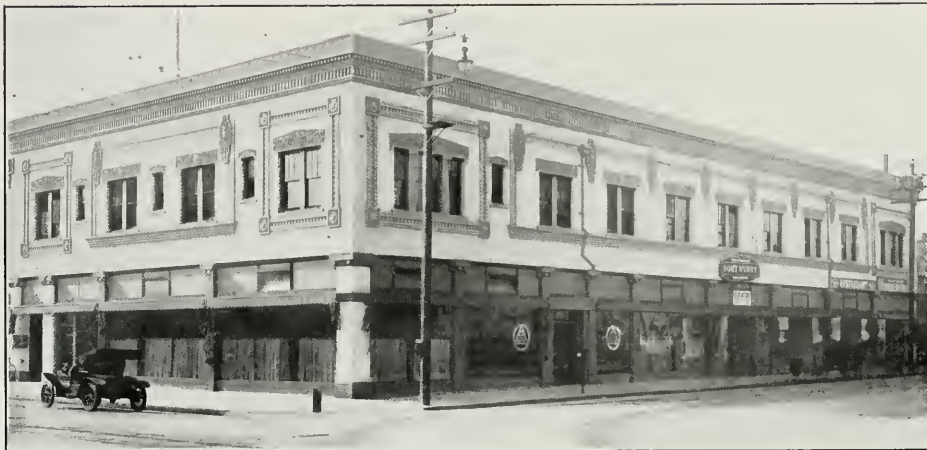
Stores and Apartments, San Jose
