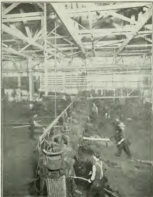
Interior Rudgear-Merle Rolling Mill, showing Splendid Equipment for Manufacturing Steel Bars
