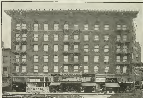
Terminal Hotel, San Francisco William Curlett & Son, Architects Pressed Brick Front, Laid in English Bond with MEDUSA WHITE PORTLAND CEMENT
