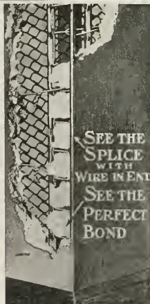
A Corner in Plaster.
