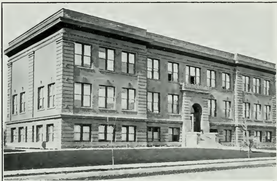
Santa Clara High School Building
