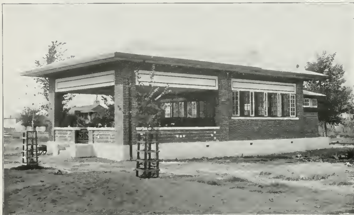
Open-Air Kindergarten Sacramento, California
