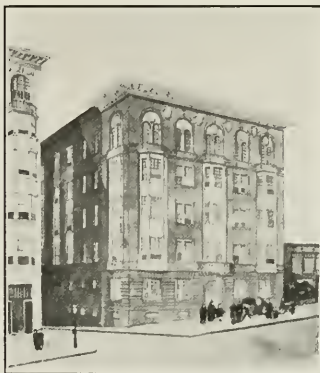
The Angelus Apartments, A. Boldocchi, Owner, Bush Street and Chelsea Place, San Francisco, Righetti & Headman, Architects R. W. Moller, Contractor
