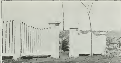
Upper Cut Shows Concrete Fence
