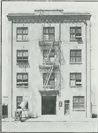
Mill Building of the Pacific Cereal Association. The First Reinforced Concrete Building Erected After the San Francisco Fire. C. A. Meussdorffer, Architect
