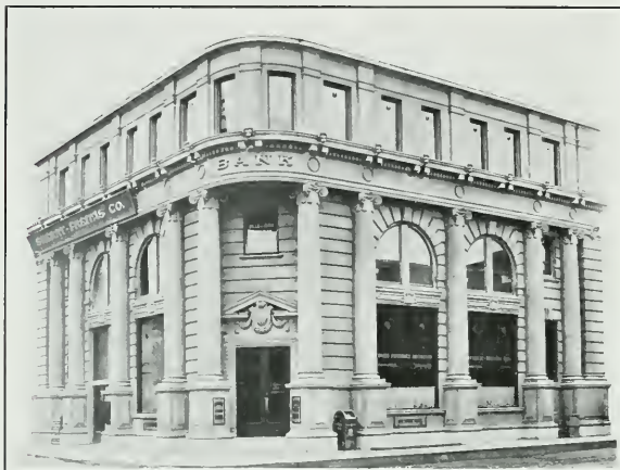
Portuguese American Bank, Designed to Carry Additional Stories, San Francisco C. A. Meussdorffer, Architect
