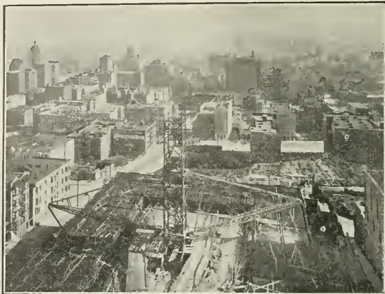
Progress Picture Showing the G-Y System of Pouring Concrete by Gravity in Operation on the L. H. Sly Apartment Hotel, Nob Hill, San Francisco
