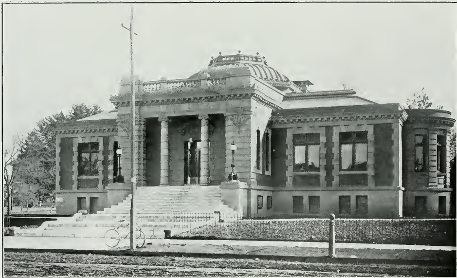
Carnegie Library Building, San Jose
