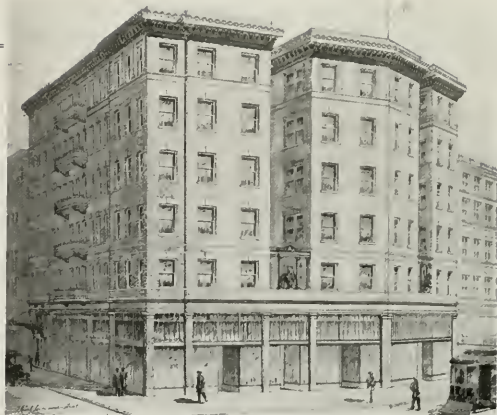
Apartment House for Marion Leventritt, San Francisco. G. A. Lansburgh, Architect
