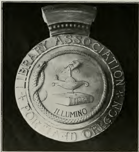
TERRA COTTA DETAIL, PUBLIC LIBRARY BUILDING PORTLAND, OREGON
