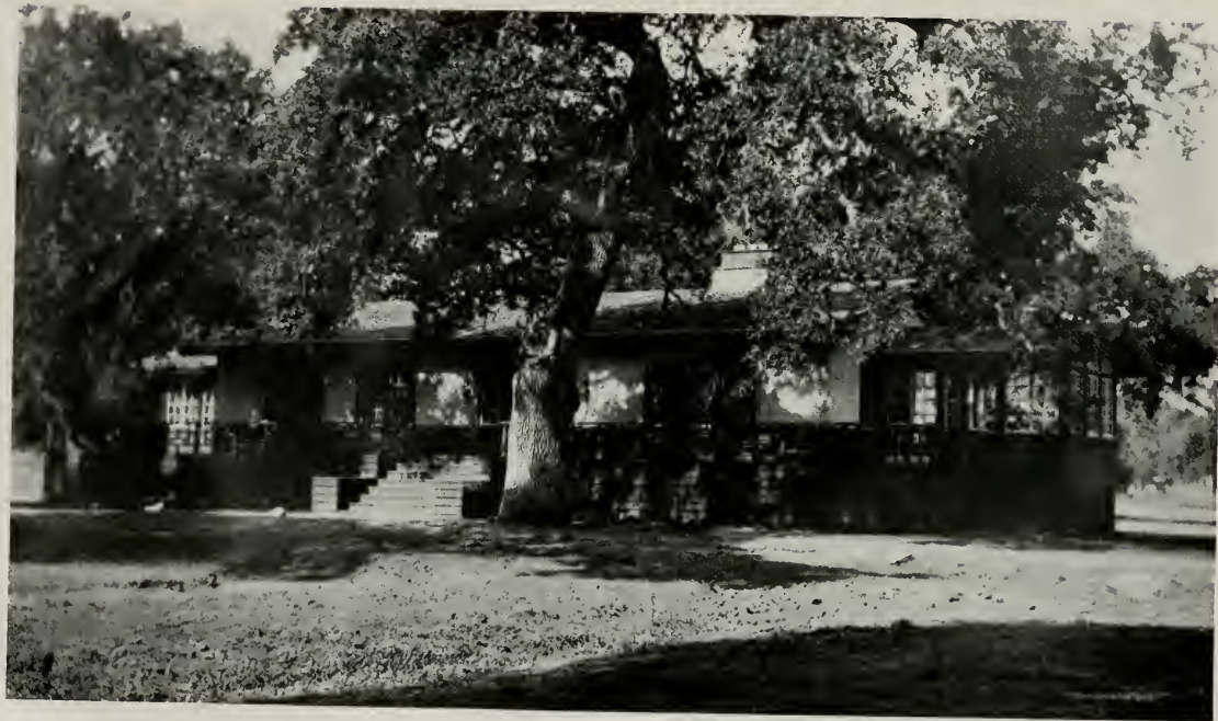
COUNTRY HOME OF DOUGLAS WATSON, ESQ., WHITE OAKS LOUIS C. MULLGARDT, ARCHITECT
