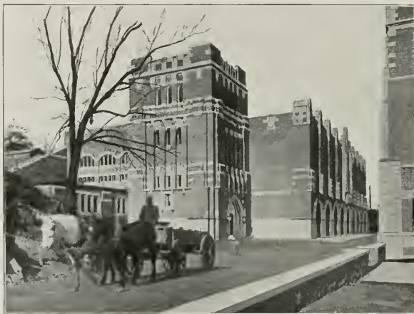
Fig. 27.—GYMNASIUM, U. S. MILITARY ACADEMY, WEST POINT. ALL TRIM ABOVE THE FIRST STORY OF CONCRETE STONE Cram, Goodhue & Ferguson, Architects
