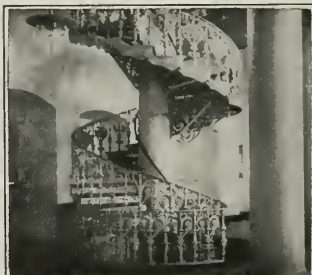
Circular Iron Stairs in Hall of Records, Sao Francisco Erected 1876
