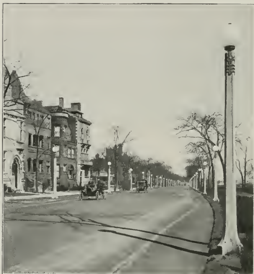
Fig. 14.—LAKE SHORE DRIVE, CHICAGO, WITH CONCRETE LAMP STANDARDS
