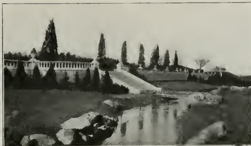
Fig. 12.—CONCRETE RETAINING WALL AND BALUSTRADE ON DUKE ESTATE, SOMERVILLE, N. J.
