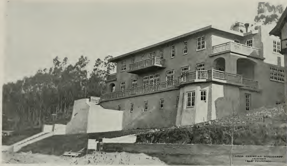
HOME OF MR. ALEXANDER SCLATER, CLAREMONT HILLS, CALIFORNIA LOUIS C. MULLGARDT, ARCHITECT
