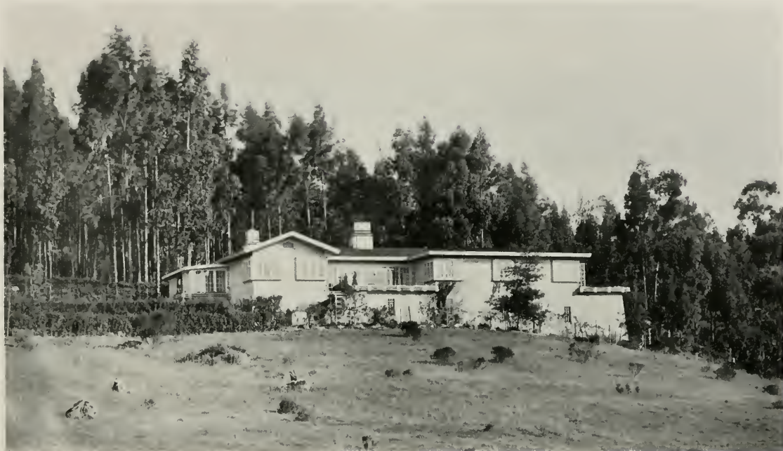
HOME FOR MR. CHARLES W. FORE, PIEDMONT HILLS LOUIS C. MULLGARDT, ARCHITECT
