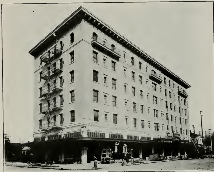
MODESTO HOTEL, MODESTO, CAL. Bernard Joseph, Architect Exterior Faced with Sacramento Sandstone Brick
