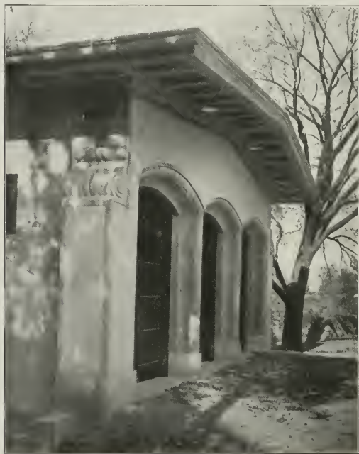
Fig. 6.—WESTERN FIRE STATION, WESTON, MASS.
