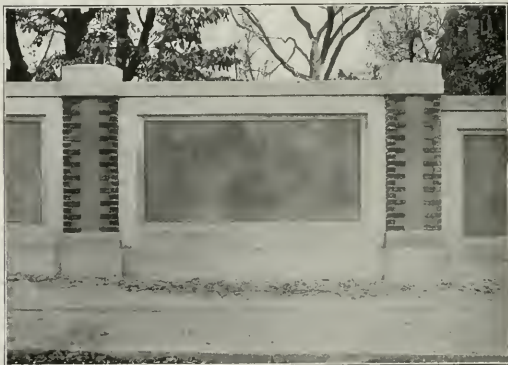
Fig. 11.—CEMENT GUN CONSTRUCTION ON WALL OF THE BOSTON ELEVATED RAILWAY
