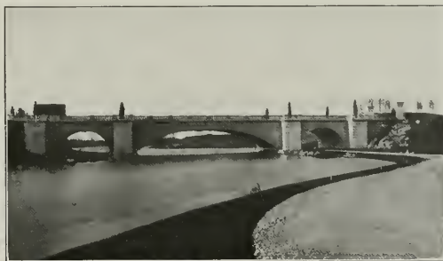
Fig. 13.—CONCRETE ARCH BRIDGE ON THE DUKE ESTATE, SOMERVILLE, N. J.
