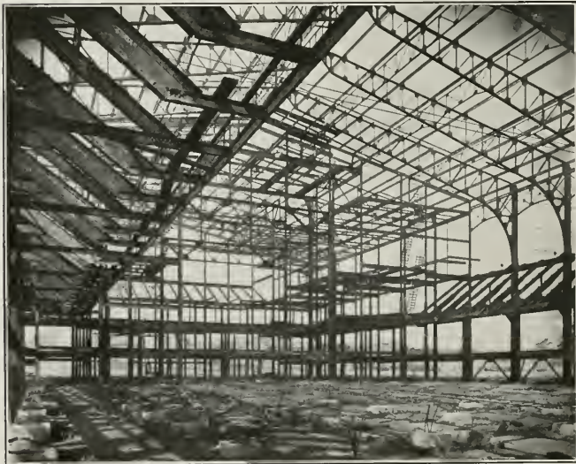
Fig. 8.—A CLOSE VIEW OF STRUCTURAL STEEL WORK
