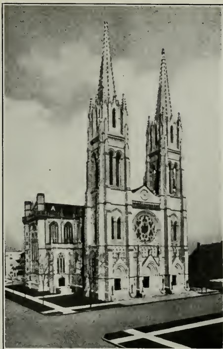
Immaculate Conception Cathedral, Denver, Colorado, in the Tower of Which Is Installed a Chime of Fifteen Bells made by the McShane Bell Foundry Co., Baltimore, Md., (Standard Electric Time Co., Sheldon Building, San Fran- cisco, Pacific Coast Agents).
