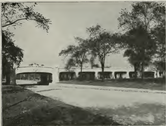
Fig. 16.—INDEPENDENCE BOULEVARD VIADUCT, BALTIMORE AND OHIO RAILWAY, CHICAGO
