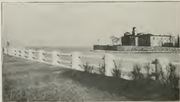
Fig. 15.—CONCRETE RAILING AROUND ENTRANCE TO JACKSON PARK HARBOR, CHICAGO
