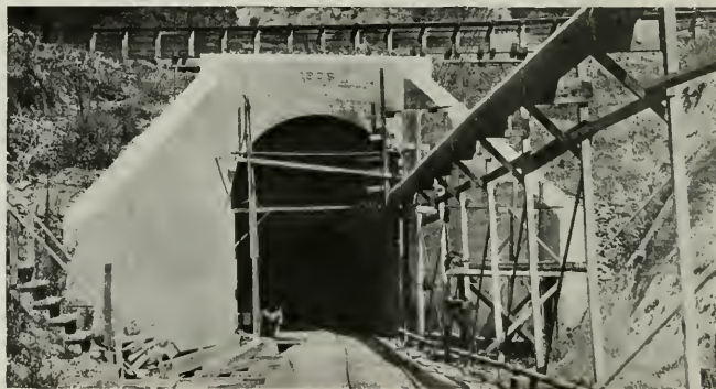
WESTERN PACIFIC RAILWAY TUNNEL PORTAL AND LINING
