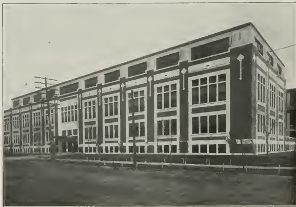
OFFICE BUILDING, PACKARD AUTOMOBILE COMPANY, BUFFALO, N. Y.
