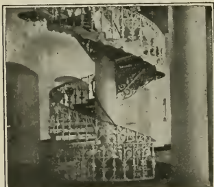
Circular Iron Stairs in Hall of Records, San Francisco Erected 1876
