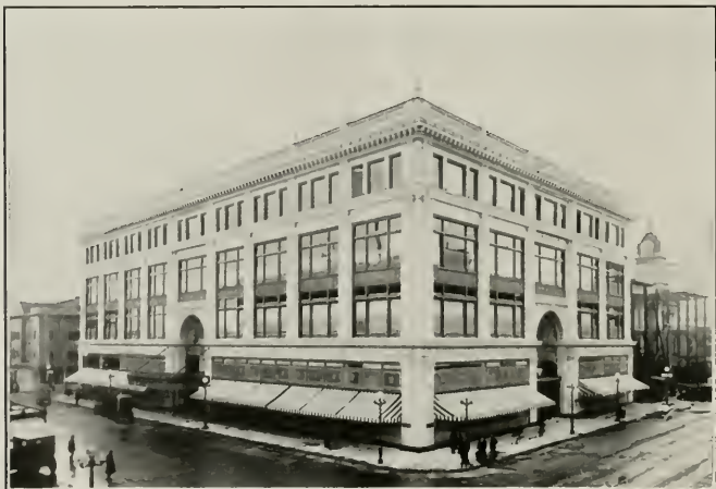
H. C. CAPWELL DEPARTMENT STORE BUILDING. OAKLAND
