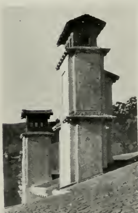
Terra Cotta Roof Covering of Mr. Taylor's Residence, Claremont Hills
