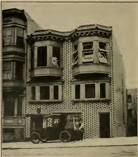
The above shows complete operation of installing Perfection Reversible Windows
