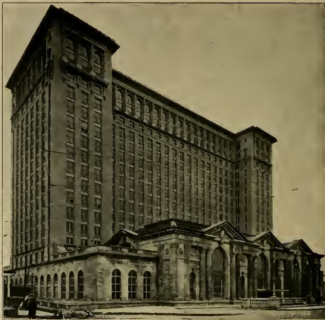
FRONT ELEVATION OF MICHIGAN CENTRAL RAILROAD STATION AND OFFICE BUILDING, DETROIT, MICHIGAN
