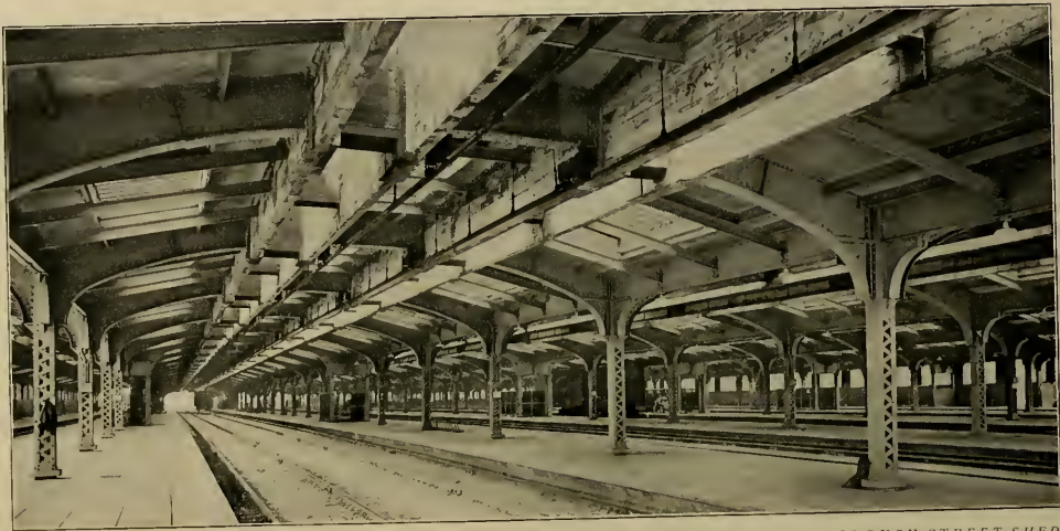
INTERIOR VIEW OF BUSH STREET SHED, MICHIGAN CENTRAL R. R. STATION, DETROIT, MICH.
