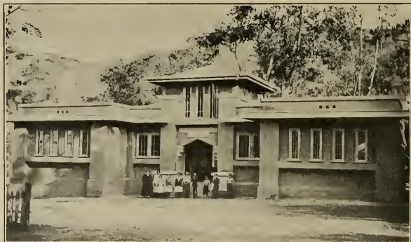
COMBINATION INDOOR AND OUTDOOR SCHOOL, SANTA CLARA COUNTY, CALIFORNIA Wolfe & Wolfe, Architects
