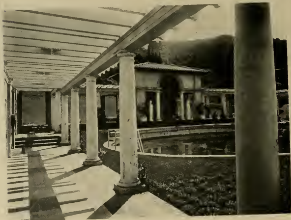
PERGOLAS AND PATIO, COUNTRY HOUSE OF HON. JAS. D. PHELAN William Curlett & Son and C. E. Gottschalk, Architects
