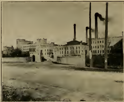
These mills of the Buffalo Cereal Company, Buffalo, New York, are built entirely of concrete. Foundations waterproofed with Hercules Waterproofing and Strengthening Compounds. Grain bins waterproofed with Hercules Liquid Waterproofing.
