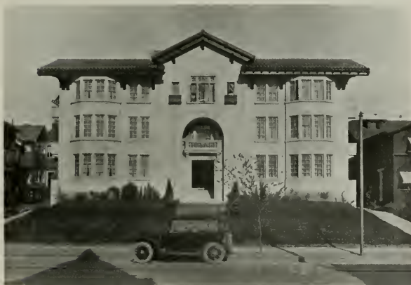
CHANNING APARTMENTS, BERKELEY, CALIFORNIA W. H. Ratcliff, Jr., Architect
