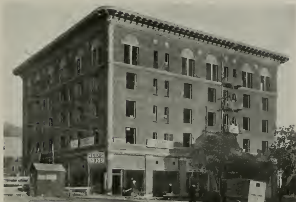
CAMBRIDGE APARTMENTS, BERKELEY, UNDER CONSTRUCTION W. H. Ratcliff, Jr., Architect
