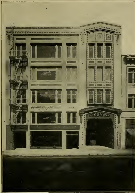
EDWARD D. SILENT BUILDING, LOS ANGELES Hunt & Burns, Architects
