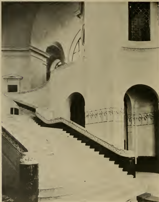
STAIRCASE, CITY HALL, OAKLAND, CALIFORNIA PALMER, HORNBOSTEL & JONES, ARCHITECTS
