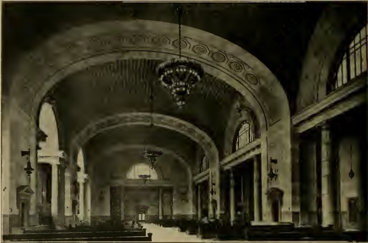
VIEW OF EAST PORTION OF MAIN WAITING ROOM, MICHIGAN CENTRAL RAILWAY STATION
