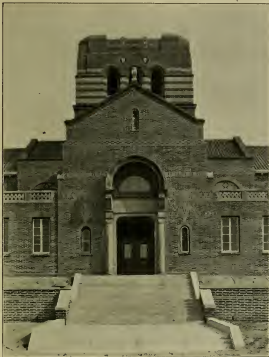
ENTRANCE—SANTA MONICA HIGH SCHOOL ALLISON & ALLISON, ARCHITECTS
