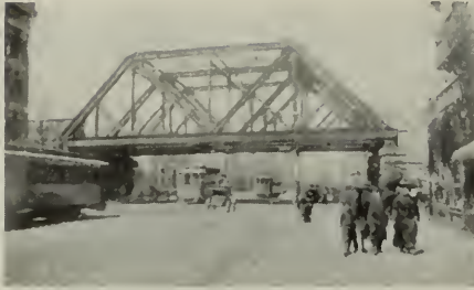
NEW YORK CENTRAL RAILROAD BRIDGE OVER STATE STREET, HARTFORD
