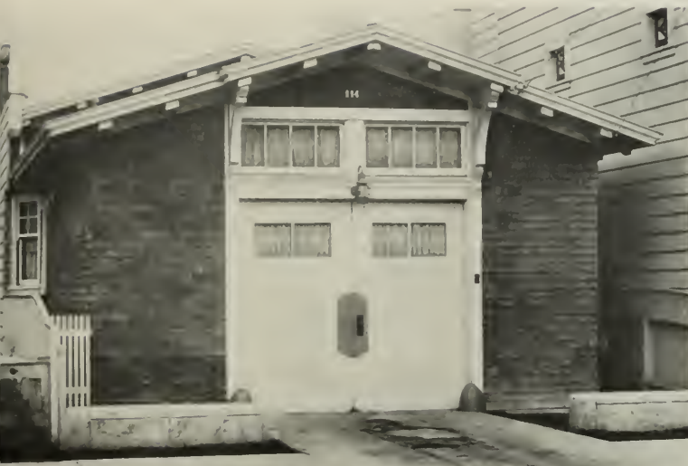
Garage with chauffeur's apartments in rear, for Mr. Frederick Hohwiesner, San Francisco Nathaniel Blaisdell, Architect
