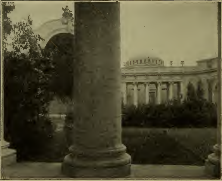
INTERIOR VIEW, COURT OF FOUR SEASONS Henry Bacon, Architect
