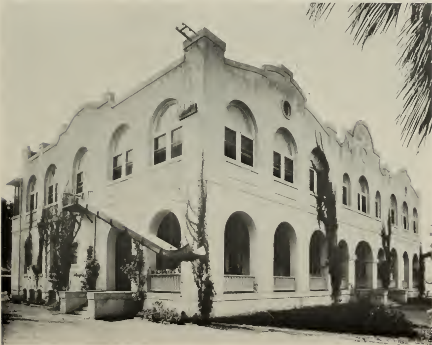
FRESNO COUNTY ORPHANAGE, FRESNO, CALIFORNIA Eugene Mathewson, Architect
