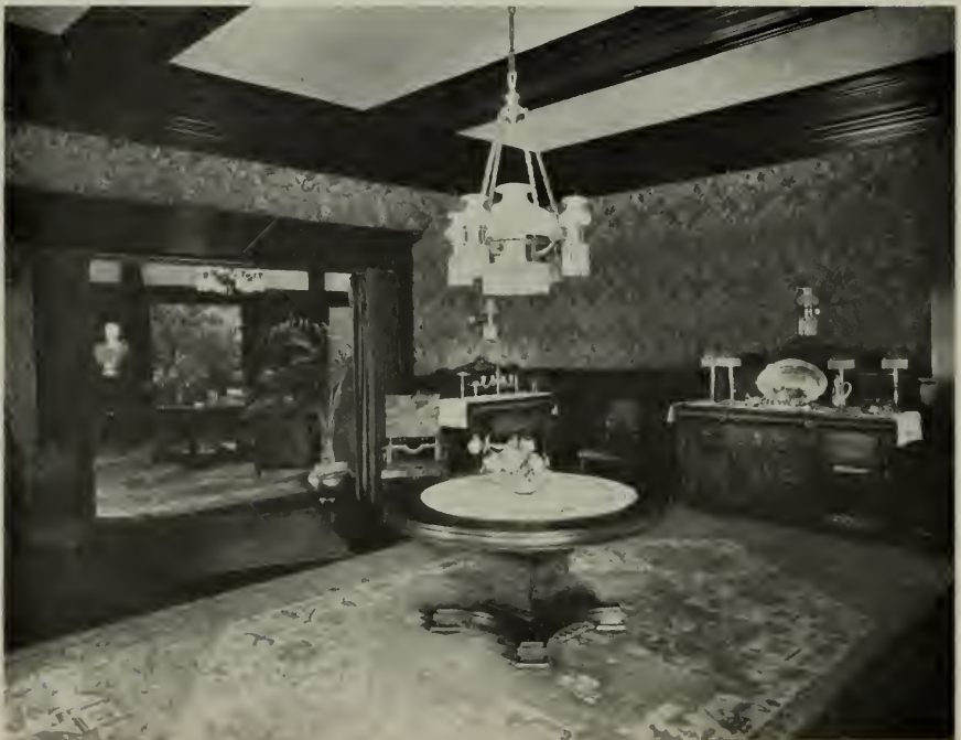
DINING ROOM, RESIDENCE OF HON. FRANK H. SHORT, FRESNO, CALIFORNIA Eugene Mathewson, Architect
