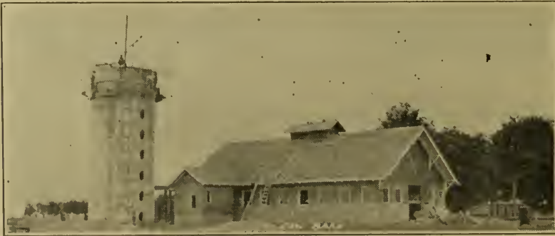
ALFARATA RANCH DAIRY AND SILO, MERCED. C. F. Wieland, Consulting Engineer.
