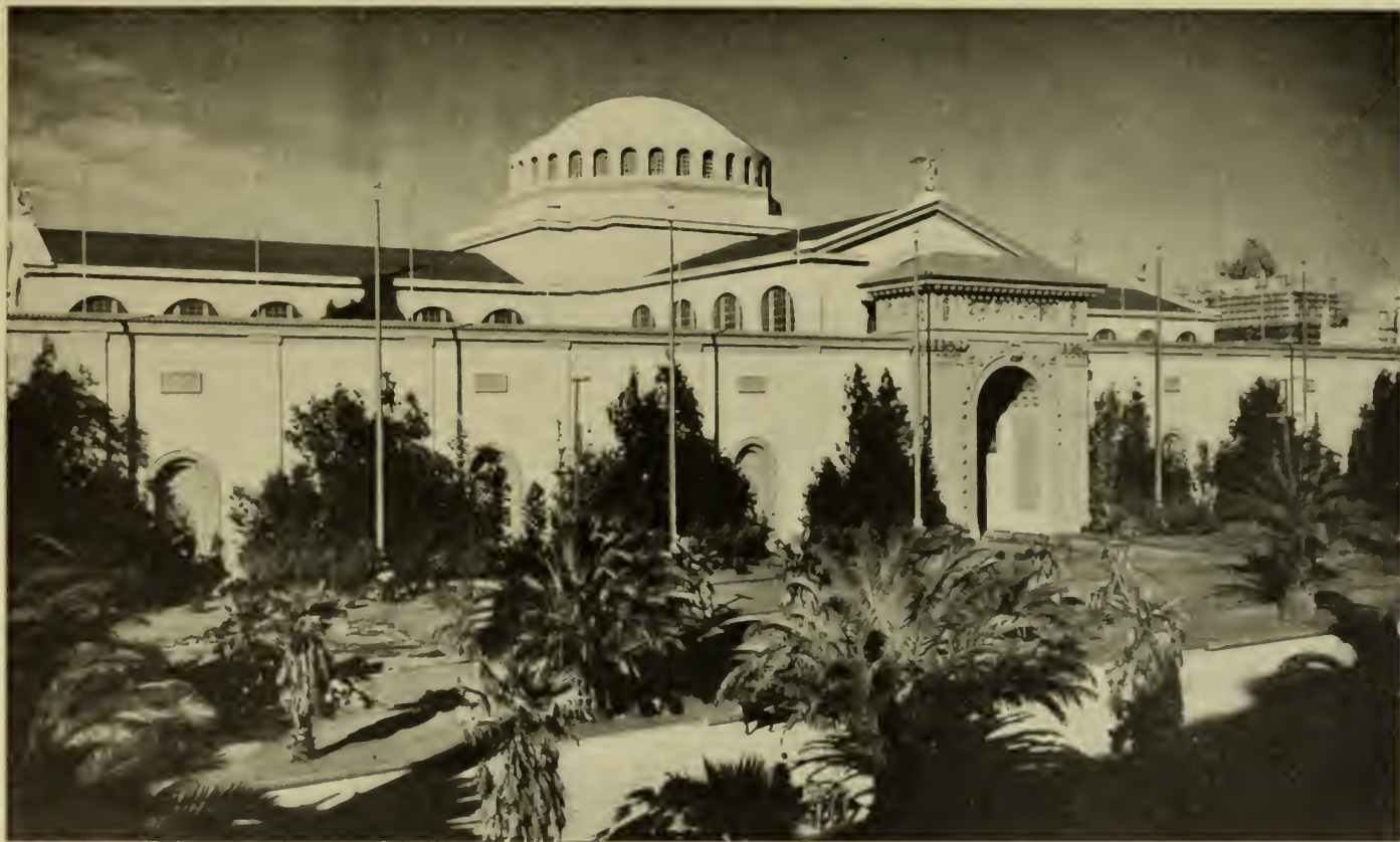
LIBERAL ARTS BUILDING, PANAMA-PACIFIC EXPOSITION BLISS & FAUVILLE, ARCHITECTS
