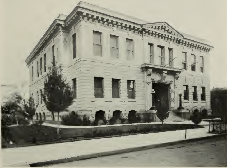
FRESNO CITY HALL, FRESNO, CALIFORNIA Eugene Mathewson, Architect
