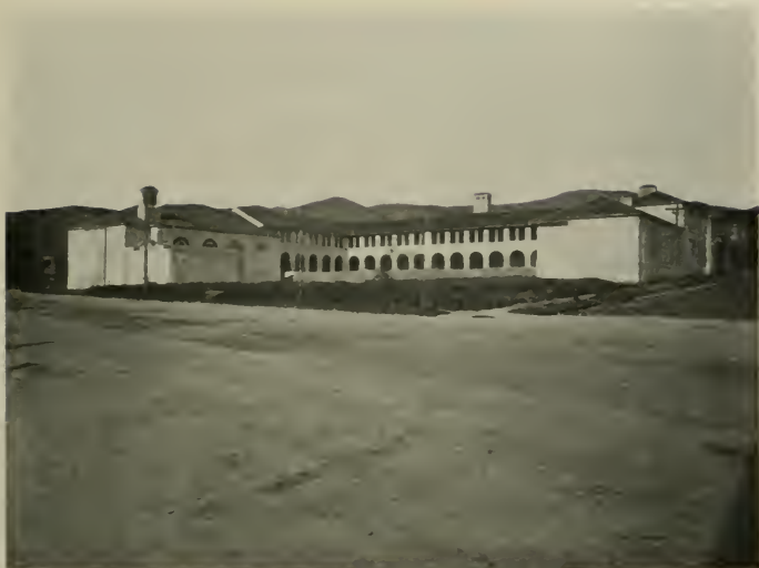
FRANCIS WILLARD SCHOOL BUILDING, BERKELEY
