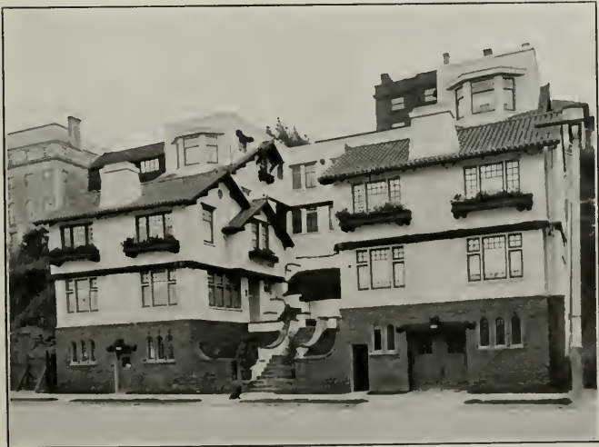
APARTMENTS FOR MR. A. B. HAMMOND AND DR. L. MACE, SAN FRANCISCO Henry C. Smith, Architect
