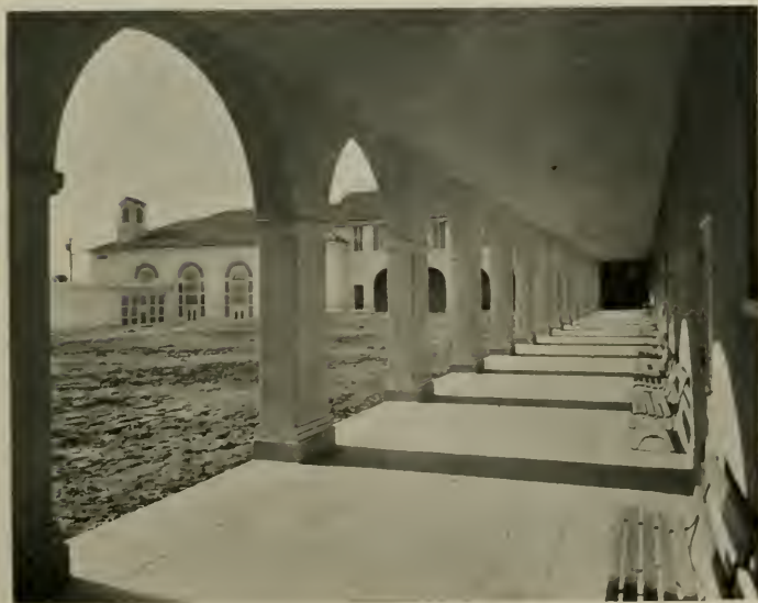
CORRIDOR, FRANCIS WILLARD SCHOOL BUILDING, BERKELEY
