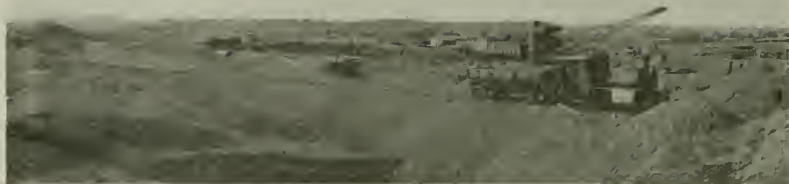
PLANT OF THE GRANT ROCK AND GRAVEL COMPANY ON THE SAN JOAQUIN RIVER,
