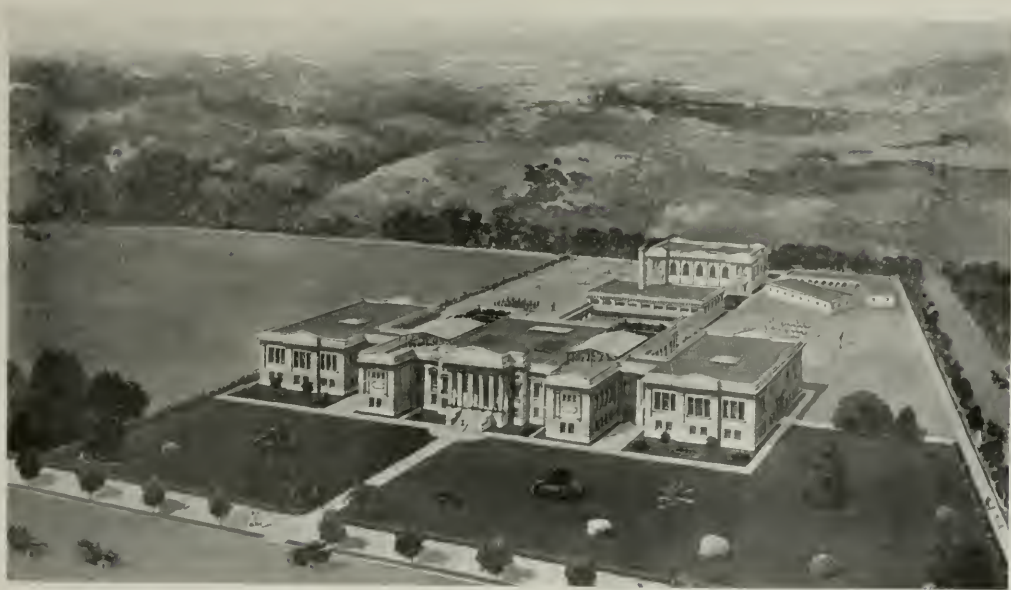
BIRDSEYE VIEW, POLYTECHNIC HIGH SCHOOL GROUP, HAYWARD HENRY C. SMITH, ARCHITECT
