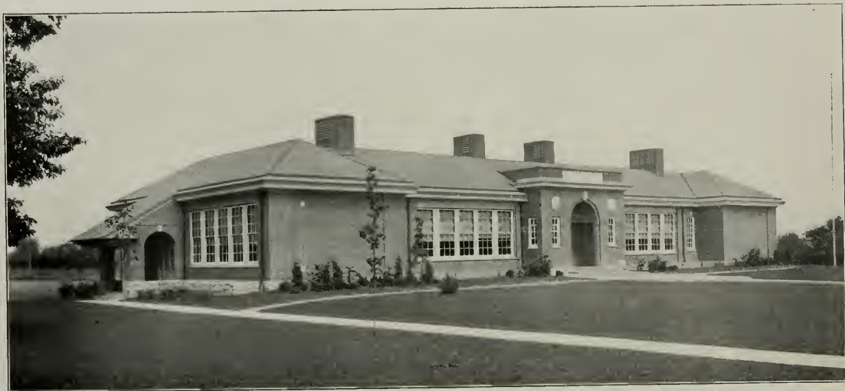
GRAMMAR SCHOOL BUILDING, ROSEMONT, PA. D. KNICKERBACKER BOYD, JOHN L. CONEYS, AND VICTOR D. ABEL, ARCHITECTS
