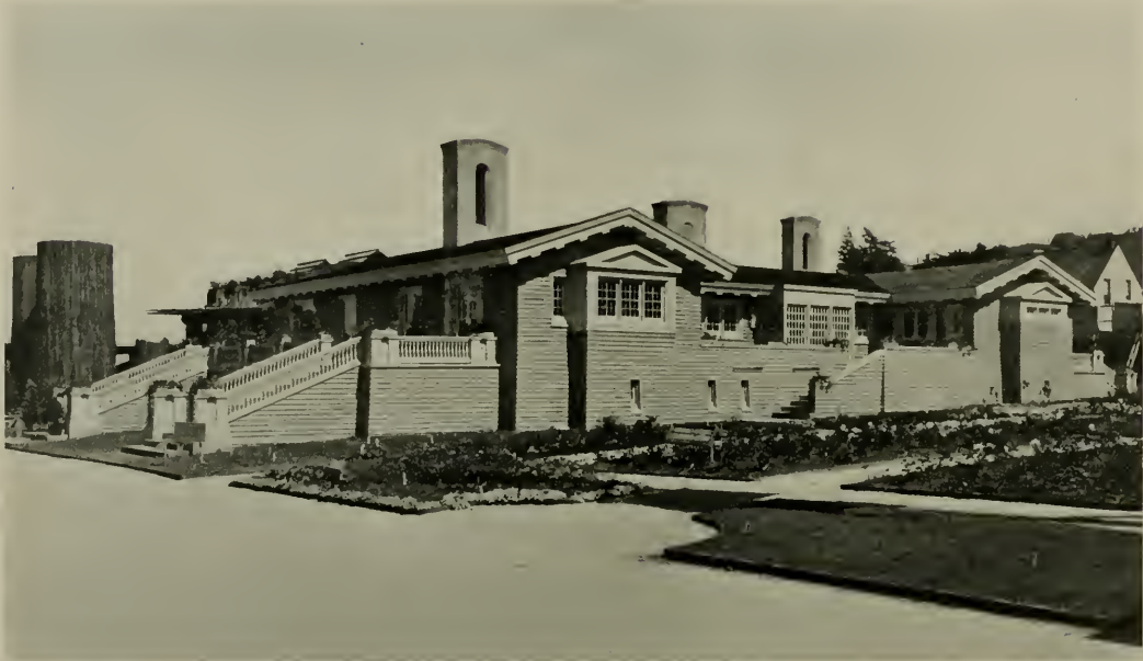
HOME OF REDWOOD AT THE RECENT EXPOSITION, NOW BEING DUPLICATED IN LOS GATOS FOOTHILLS LOUIS C. MULLGARDT, ARCHITECT
