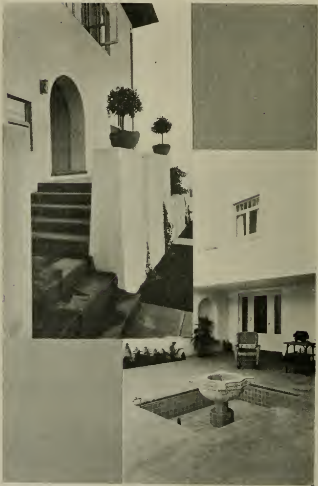
ENTRANCE DETAIL AND PATIO TO SOUTHERN CALIFORNIA MISSION HOME IRVING J. GILL, ARCHITECT
