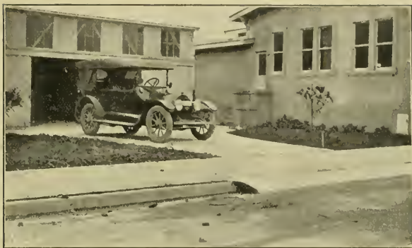
CORRUGATED IRON CULVERT FOR GARAGE APPROACH
