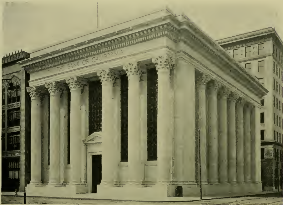
THE BANK OF CALIFORNIA, SAN FRANCISCO BLISS & FAVILLE, ARCHITECTS
