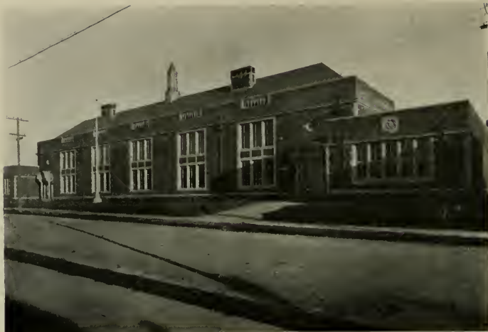
NORTH ELEVATION, EDISON SCHOOL BUILDING, BERKELEY W. H. Ratchiff, Jr., Architect
