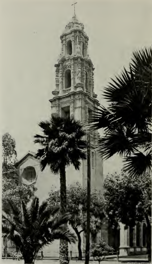
FIRST CONGREGATIONAL CHURCH, RIVERSIDE MYRON HUNT, ARCHITECT
