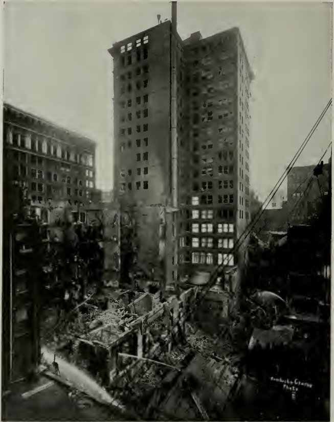
SHOWING THE EFFICACY OF GOOD FIRE WALLS, METAL WINDOW FRAMES AND WIRE GLASS
