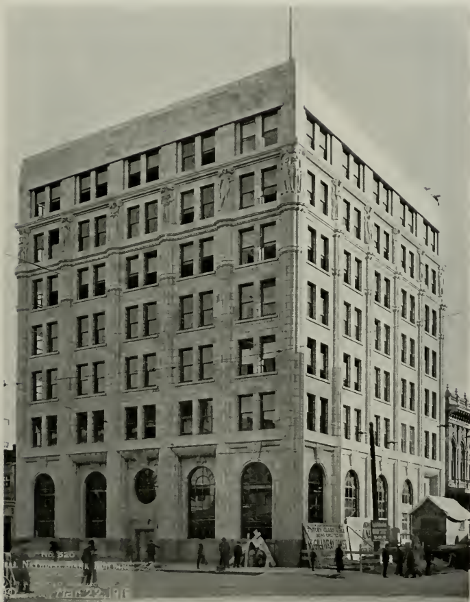
CAPITAL NATIONAL BANK, SACRAMENTO R. A. HEROLD, ARCHITECT Exterior of granite glazed terra cotta by Steiger Terra Cotta and Pottery Works
