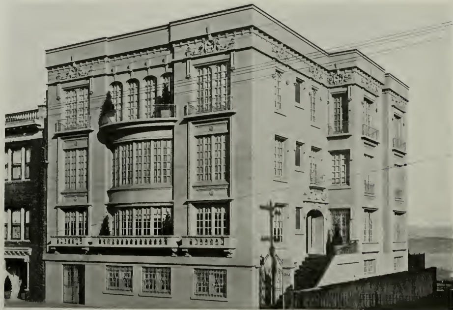
BROWNLEE APARTMENTS, SAN FRANCISCO HENRY C. SMITH, ARCHITECT
