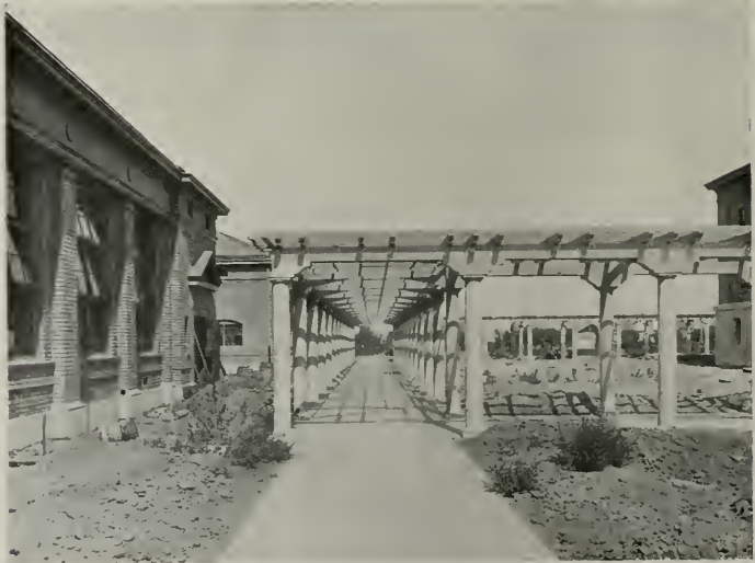
PERGOLA CONNECTING LODI HIGH SCHOOL GROUP Stone & Wright, Architects
