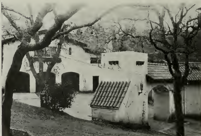
GARAGE COURT, W. B. WELLMAN RESIDENCE, LOS ALTOS Henry C. Smith, Architect
