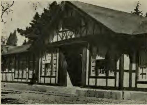
An Entrance Detail, John Muir School, Berkeley
