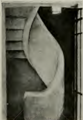
Spiral concrete staircase.
