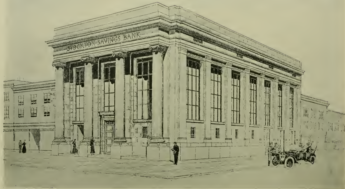
STOCKTON SAVINGS BANK, STOCKTON CHARLES W. DICKEY, ARCHITECT
