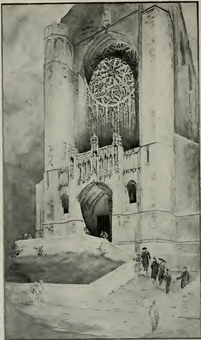
ENTRANCE DETAIL, ST. PATRICK'S CHURCH, BISBEE, ARIZONA ALBERT C. MARTIN, ARCHITECT
