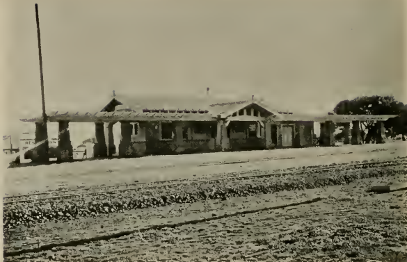
DEPOT AT LOS ALTOS, CALIFORNIA Designed by Architectural Bureau, Southern Pacific Company
