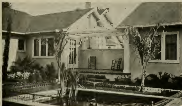
ENTRANCE TO HOUSES 5 AND 6—NOTE ARRANGEMENT OF BACK YARDS
