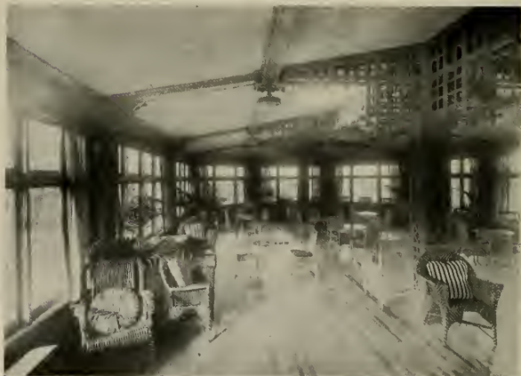
SUN PORCH, HOTEL WHITCOMB, SAN FRANCISCO Wright & Rushforth, Architects
