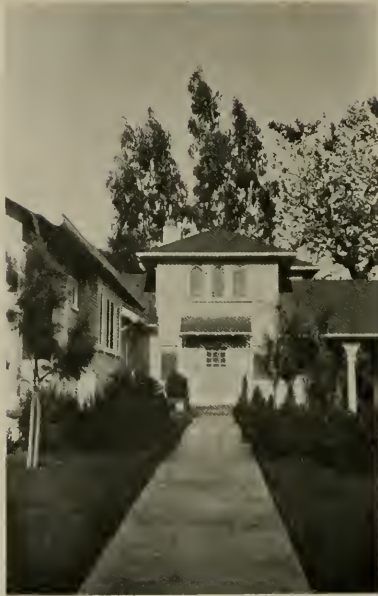
VISTA TO ENTRANCE OF HOUSE 7, COURT 2
