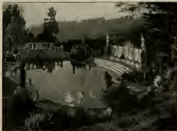
CONCRETE SWIMMING TANK, ESTATE OF MR. J. F. CARLSTON, REDWOOD CANYON, CALIFORNIA
