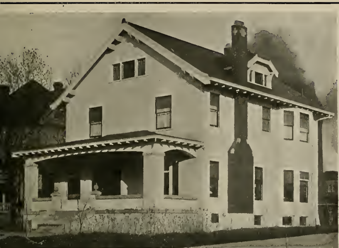
Typical Residence in which Armcro Iron Spiral Lath is used as a Base for Stucco
