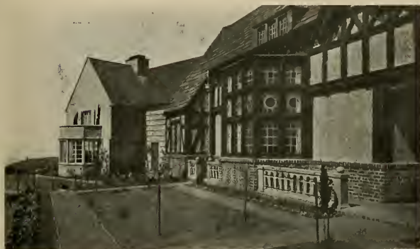
THE SAME COTTAGE, REBUILT AND ENLARGED, NOW THE PROPERTY OF PROF. A. U. POPE, CRAGMONT Wood & Simpson, Architects
