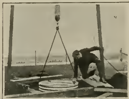
A completed job.
