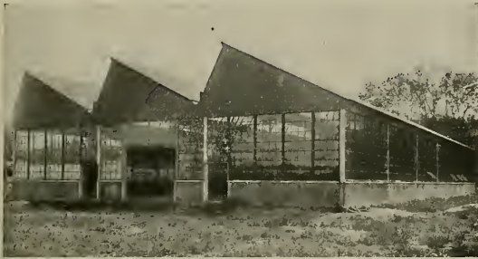
New "Oaylight Factory" of the Farm Engineering Company, Sand Springs, Oklahoma. C. M. Pritchard, Architect, Tulsa, Oklahoma. Armco (American Ingot) Iron Roofing and Siding Employed
