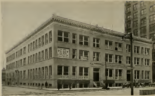
CARMEN-JOHNSON BUILDING, SAN FRANCISCO PAINTED WITH GOLDEN STATE BRICK AND CEMENT COATING
