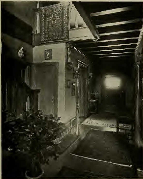
ENTRANCE HALL AND STAIRWAY, RESIDENCE AND STUDIO OF MR. HAIG PATIGIAN, SAN FRANCISCO WARD & BLOHME, ARCHITECTS
