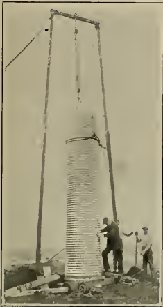
Showing a simple but efficient derrick for handling curbing.
