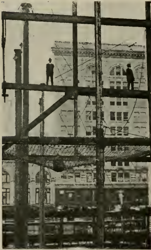
Safety Net Used to Protect Structural Workers on New California Theatre
