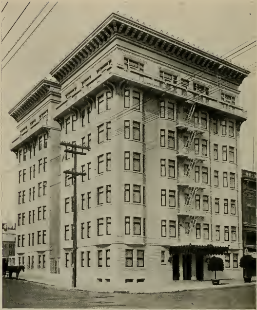
McKENZIE APARTMENTS, VAN NESS AVENUE AND BUSH STREET, SAN FRANCISCO
