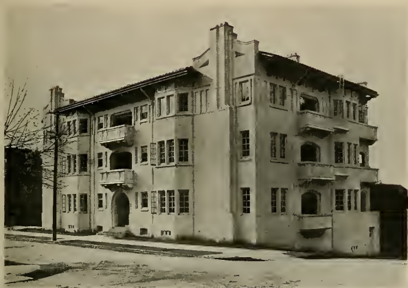
GLEN GARRY APARTMENTS, BERKELEY W. H. Ratcliff, Jr., Architect
