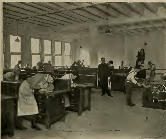
CORNER OF CABINET AND JOINER SHOP, COGSWELL POLYTECHNICAL COLLEGE
