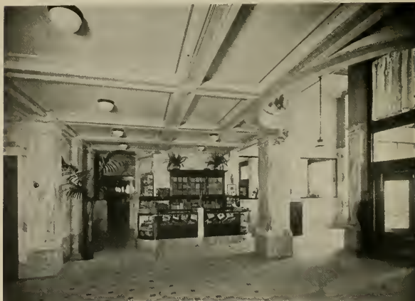
LOBBY, NEAR ENTRANCE, HOTEL WHITCOMB, SAN FRANCISCO Wright & Rushforth, Architects
