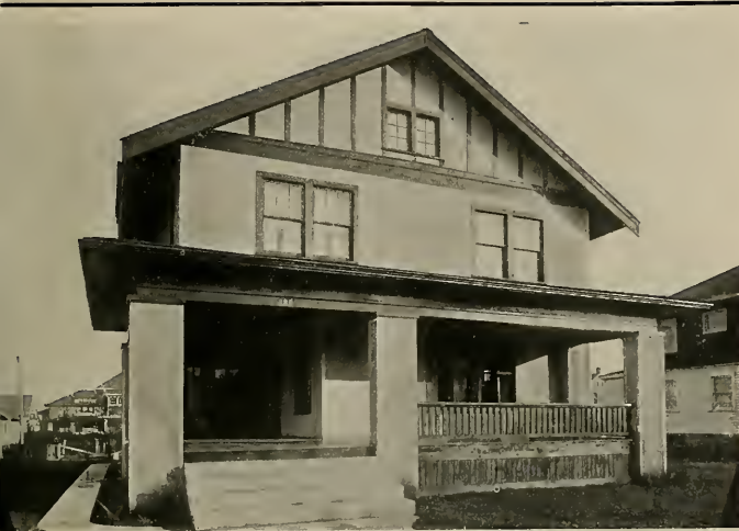
THE BRAIN RESIDENCE AT SPRINGFIELD, OHIO. ARMCO IRON SPIRAL LATH EMPLOYED AS BASE FOR STUCCO
