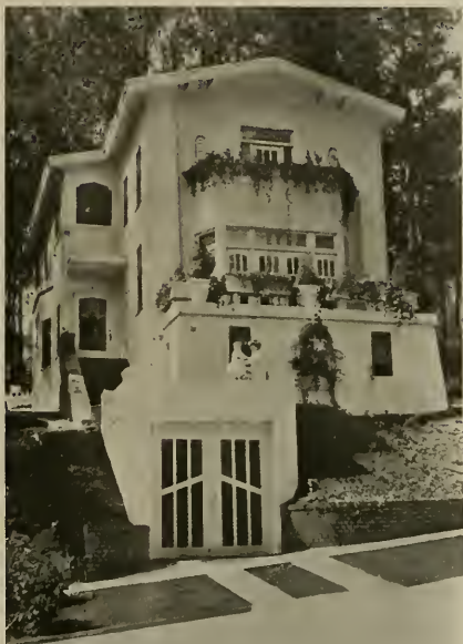
RESIDENCE OF MR. E. C. DUNCAN, FOREST HILL, SAN FRANCISCO Heiman-Schwartz, Architects
