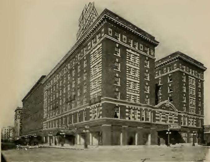
Hotel Orlando, Decatur, Illinois, Holmes & Flinn, Chicago, Architects. All Sheet Metal Work of ARMCO Iron.
