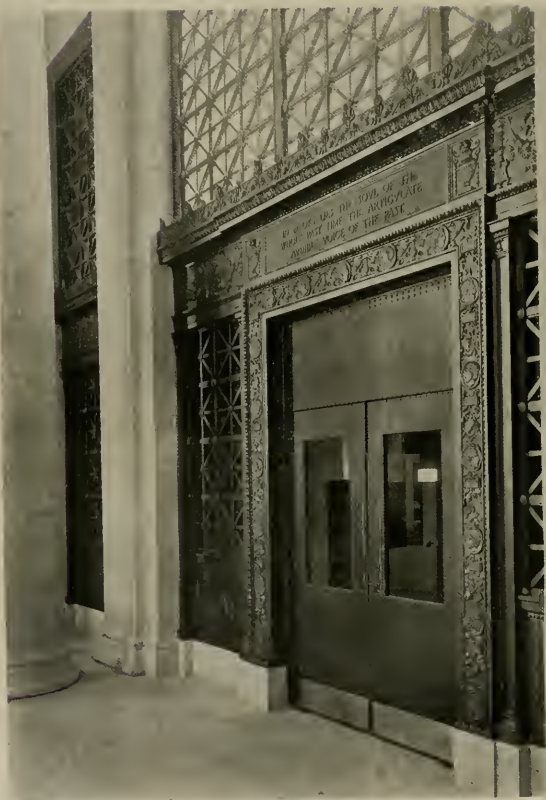
BRONZE SCREEN, DELIVERY ROOM, SAN FRANCISCO PUBLIC LIBRARY GEORGE W. KELHAM, ARCHITECT
