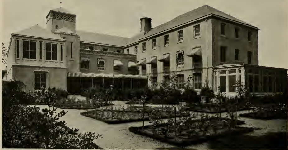
SLATE ROOF FOR HOSPITAL, SAN MATEO, CALIFORNIA LEWIS P. HOBART, ARCHITECT
