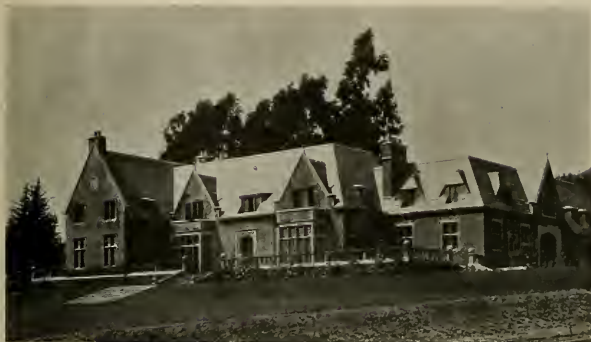
SLATE ROOF ON TUDOR RESIDENCE, NEAR LOS ANGELES Morgan, Walls & Morgan, Architects
