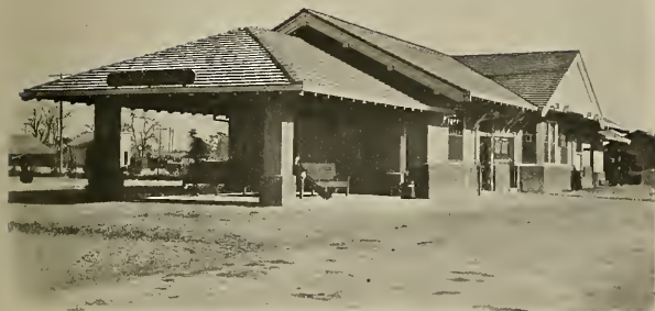
DEPOT AT TURLOCK, CALIFORNIA Designed by Architectural Bureau, Southern Pacific Company
