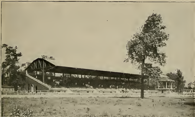
Grand Stand at the Hamilton Fair Grounds, Hamilton, Ohio. The Roofing is Corrugated "Armco" Iron
