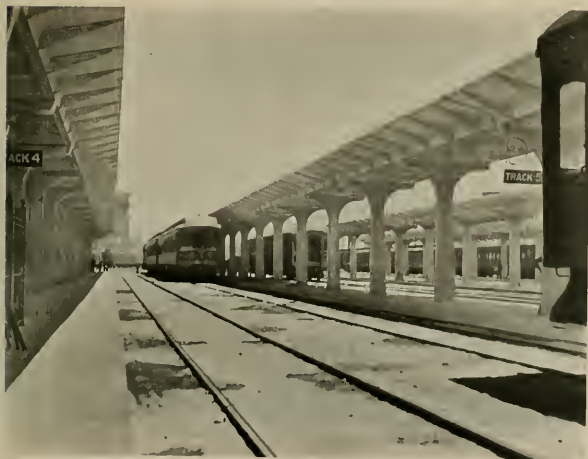
UMBRELLA SHEDS AND TRACKS, CENTRAL STATION, LOS ANGELES
