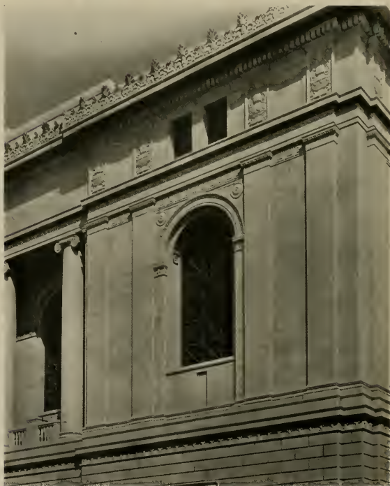
ELEVATION, WEST FACADE AND DETAIL, SAN FRANCISCO PUBLIC LIBRARY GEORGE W. KELHAM, ARCHITECT
