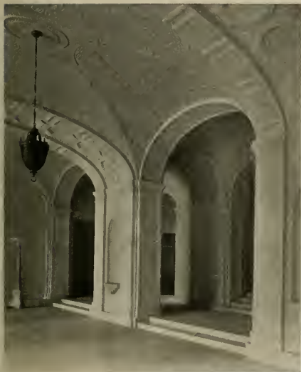
ENTRANCE HALL, SAN FRANCISCO PUBLIC LIBRARY
