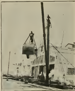
Delivering Plastering Sand by Boat
