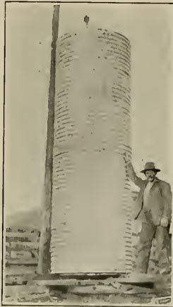
"Armeo" Iron Galvanized, Corrugated Well Curbing of 42" diameter being installed on ranch of Geo. C. Russell near Enterprise, Oregon.
