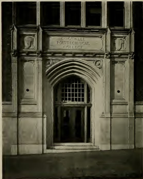
FOLSOM STREET ENTRANCE, COGSWELL POLYTECHNICAL COLLEGE, SAN FRANCISCO FREDERICK H. MEYER, ARCHITECT
