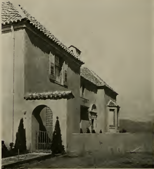
WEST ELEVATION, HOUSE OF MR. GEORGE W. KELHAM George W. Kelham, Architect
