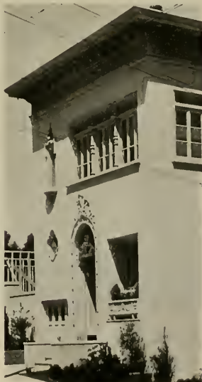
ENTRANCE DET. III, HOUSE OF MR. J. O. GANTNER SAN FRANCISCO Louis M. Upton, Architect
