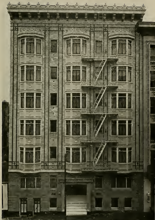
GEORGE BENNETT APARTMENT HOUSE, SAN FRANCISCO C. O. CLAUSEN, Architect
