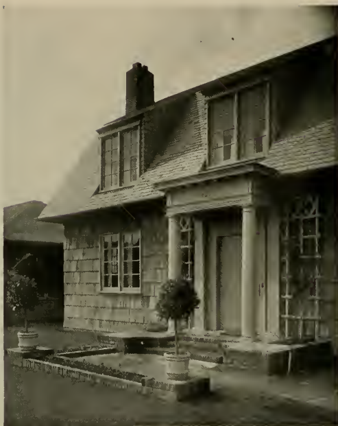
HOUSE OF MR. W. S. CRISMON, LOS ANGELES Arthur R. Kelly, Architect
