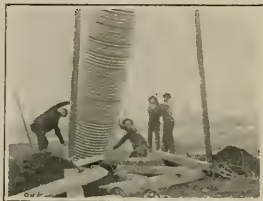
Hoisting a length of corrugated well curbing into position for lowering.
