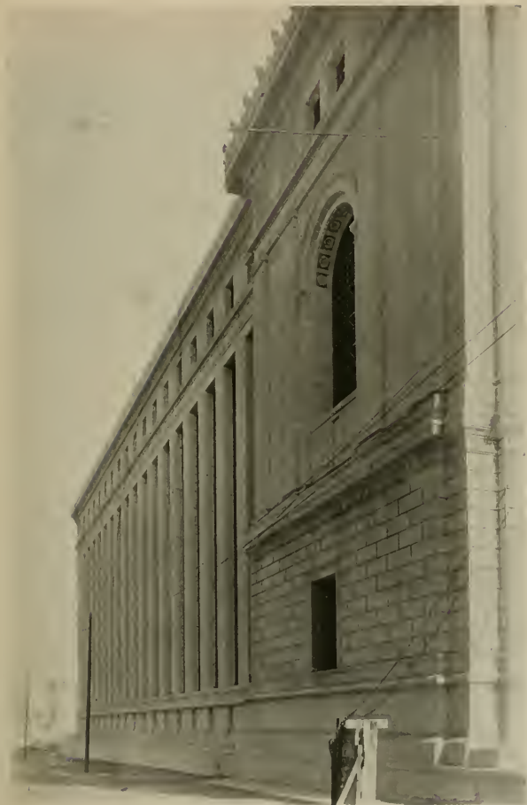
McALLISTER STREET FACADE, SAN FRANCISCO PUBLIC LIBRARY GEORGE W. KELHAM, ARCHITECT
