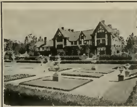
House of Mrs. D. T. Murphy, Hillsborough, Cal.
