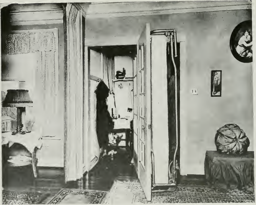
PORTAL BED WITH DOOR WIDE OPEN, SHOWING THREE-FOOT ENTRANCE TO DRESSING CLOSET.
