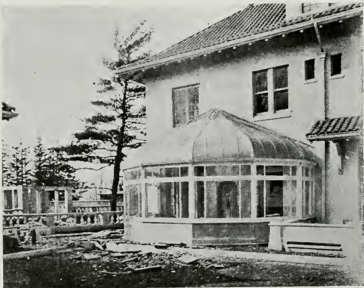
Showing how a conservatory may be adapted to this type of stucco house. Harold Hill Blossom designed the tiled fountain in this greenhouse in Brookline, Mass., which adds the final charm to the room.
