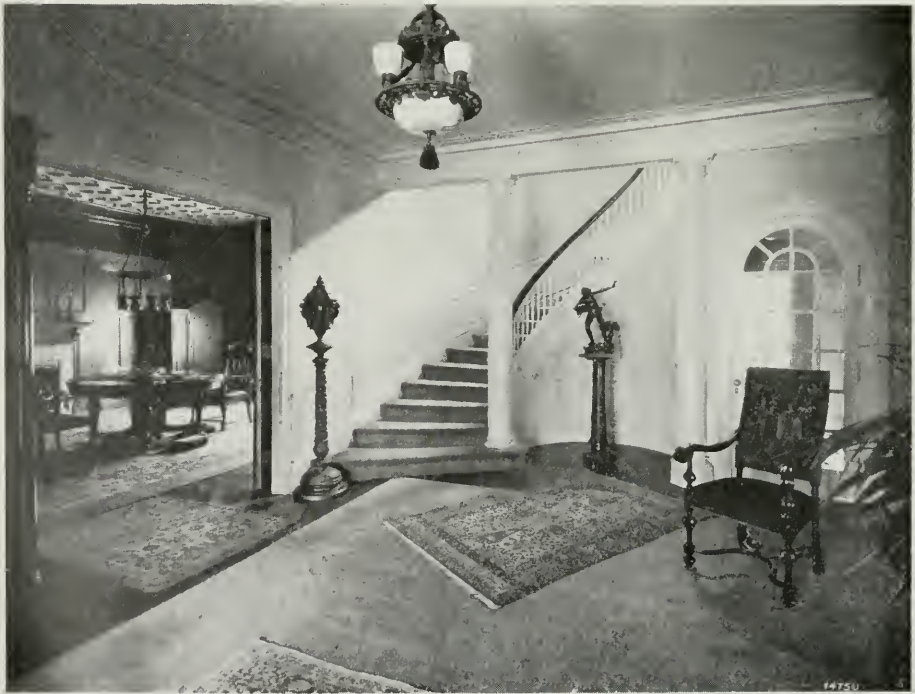
INTERIOR, THE ABE MEIER HOUSE, PORTLAND, OREGON A. E. Doyle, Architect
