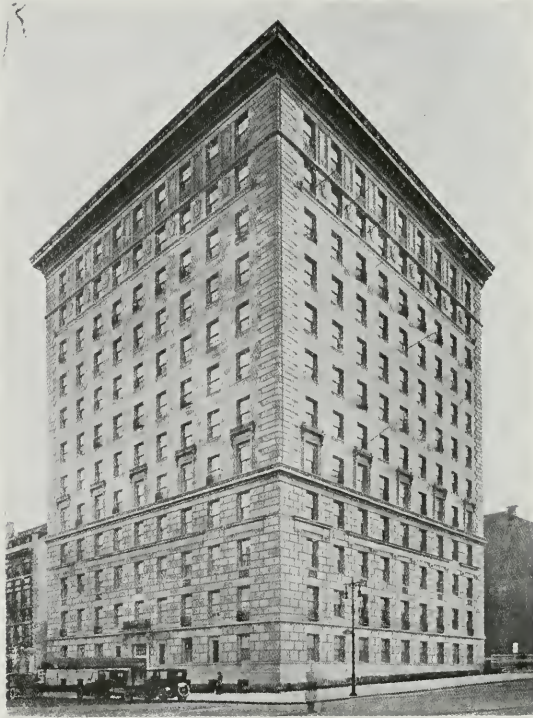
APARTMENT BUILDING, FIFTH AVE., NEW YORK CITY. . . Awarded Gold Medal by New York Chapter, A. I. A., for multiple dwellings over six stories high. J. E. R. Carpenter, Architect.
