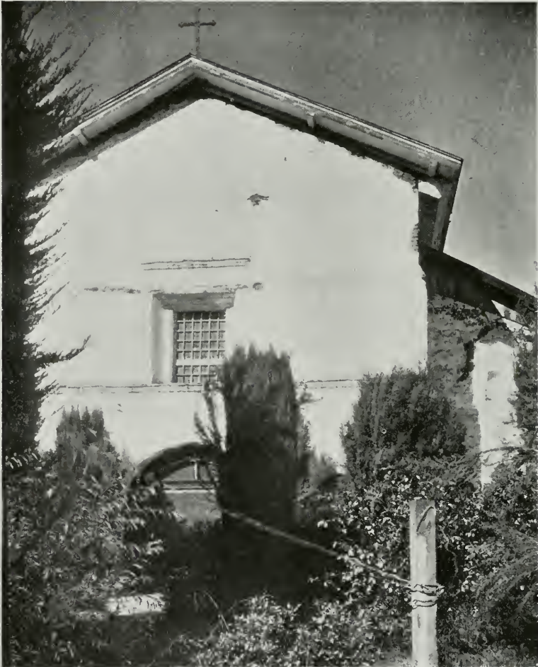
FACADE OF CHURCH, SAN JUAN BAUTISTA MISSION
