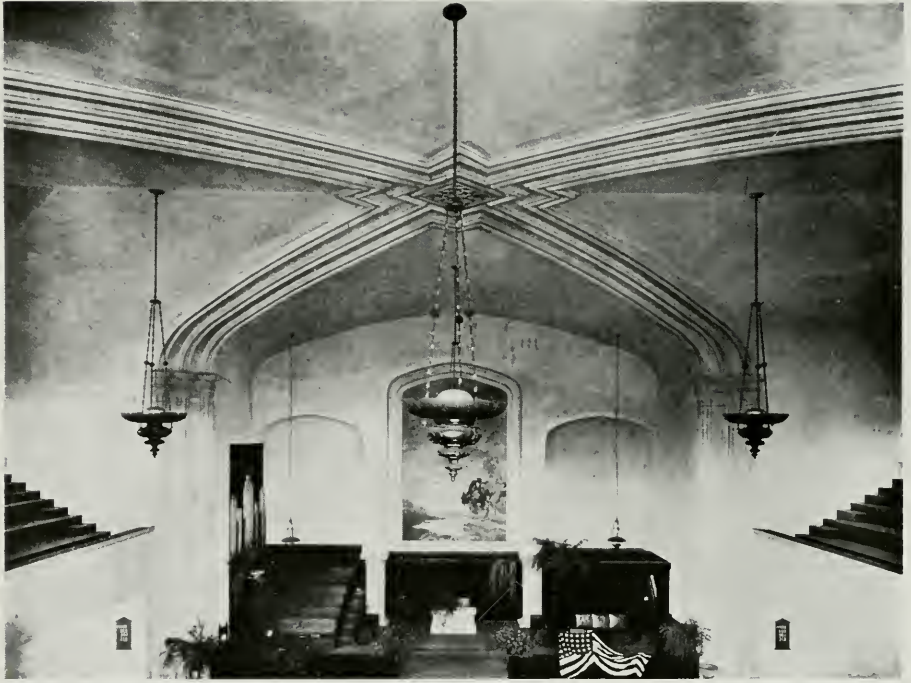
CHANCEL, PLYMOUTH CHURCH, OAKLAND William Knowles, Architect
