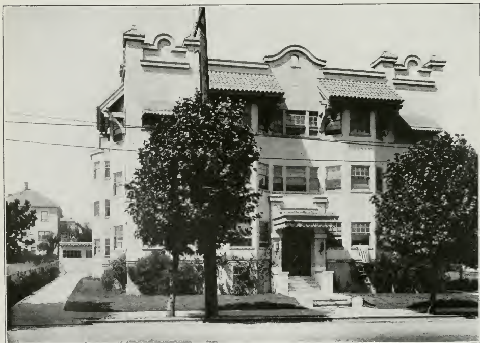
LENNOX APARTMENTS, OAKLAND Alvin Stern, Architect
