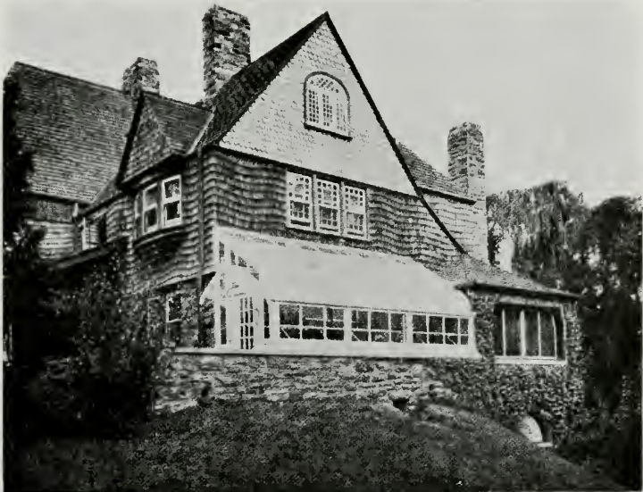
An excellent type of modern conservatory construction. The most noticeable features are the curved glass connecting the roof and sides, and the high eaves.
