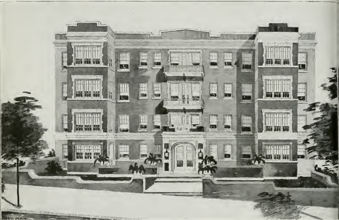
CLIFTON APARTMENTS, NASHVILLE, TENN. Marr & Holman, Architects
