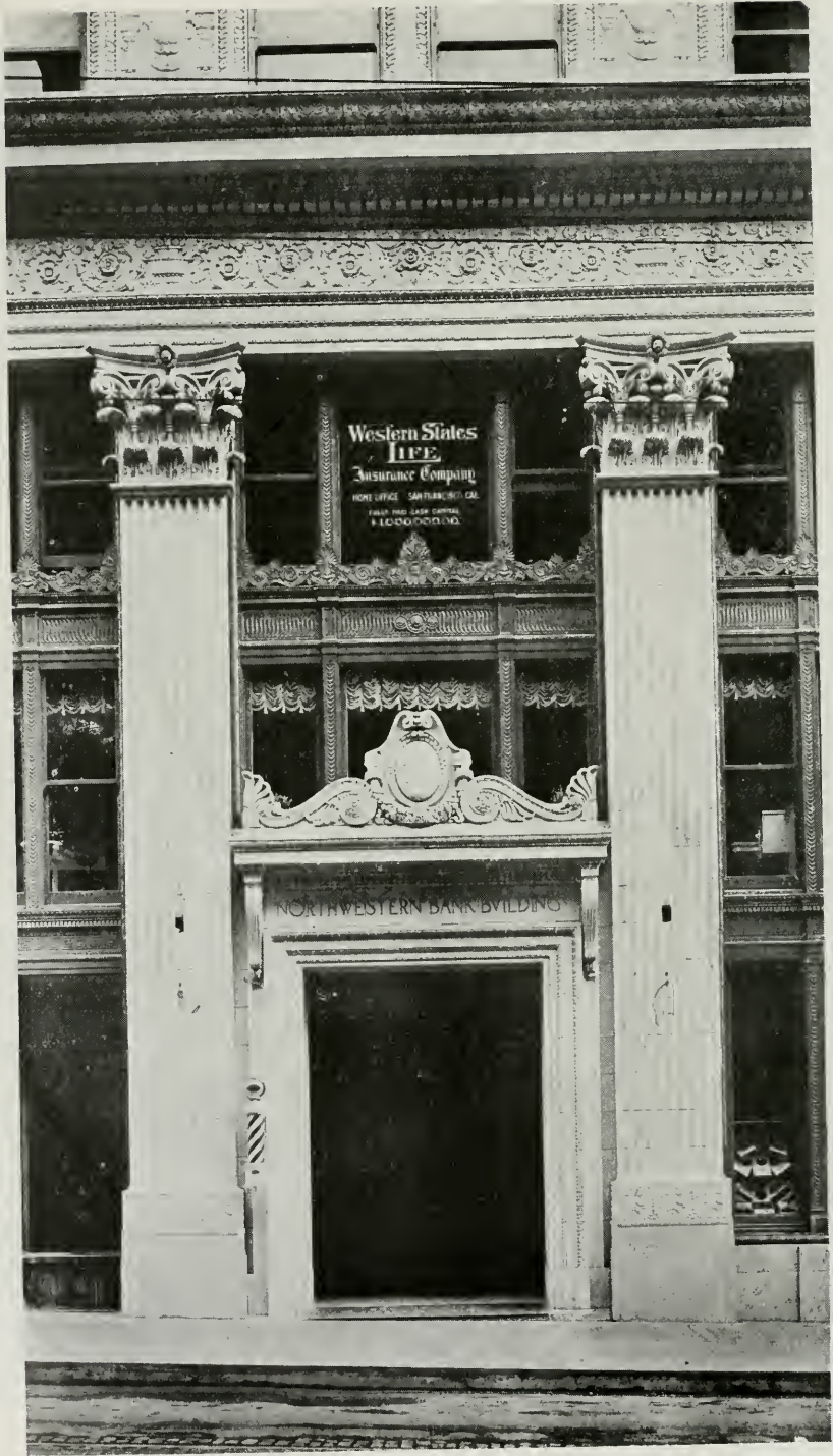
ENTRANCE, NORTH WESTERN NATIONAL BANK BUILDING PORTLAND, OREGON. A. E. DOYLE, ARCHITECT
