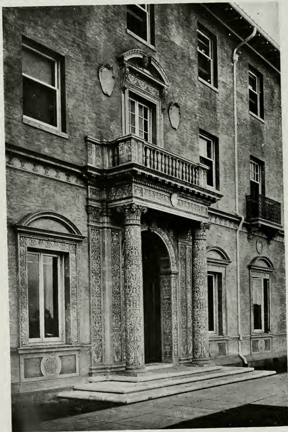
ENTRANCE, DORMITORY FOR WOMEN LELAND STANFORD JR. UNIVERSITY GEORGE W. KELHAM, ARCHITECT
