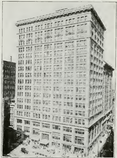
102 sets of Ideal Fixtures for two-speed doors comprise the elevator door equipment of the Union Trust Building at Cincinnati, Ohio.
