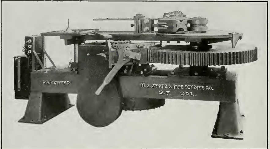
U. S. POWER PIPE BENDING MACHINE, 3 INCH CAPACITY MODEL, MOTOR-DRIVEN
