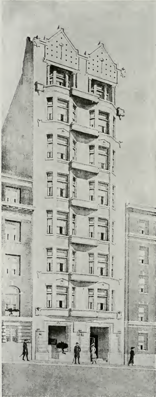
APARTMENT HOUSE FOR MR. A. W. WILSON, SAN FRANCISCO C. A. MEUSSDORFFER, ARCHITECT
