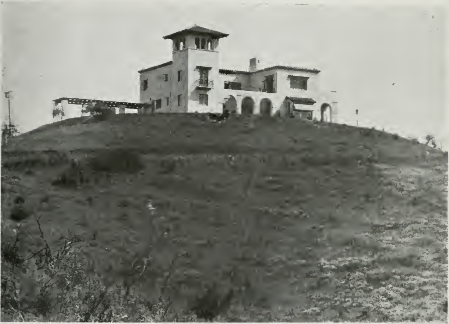
RESIDENCE OF MR. O. W. ROBERTSON, OJAI (Inspired by the community improvements) Mead & Requa, Architects
