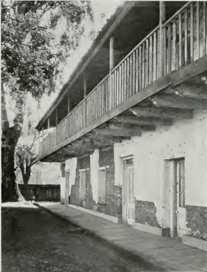
CASTRO HOUSE, SAN JUAN
