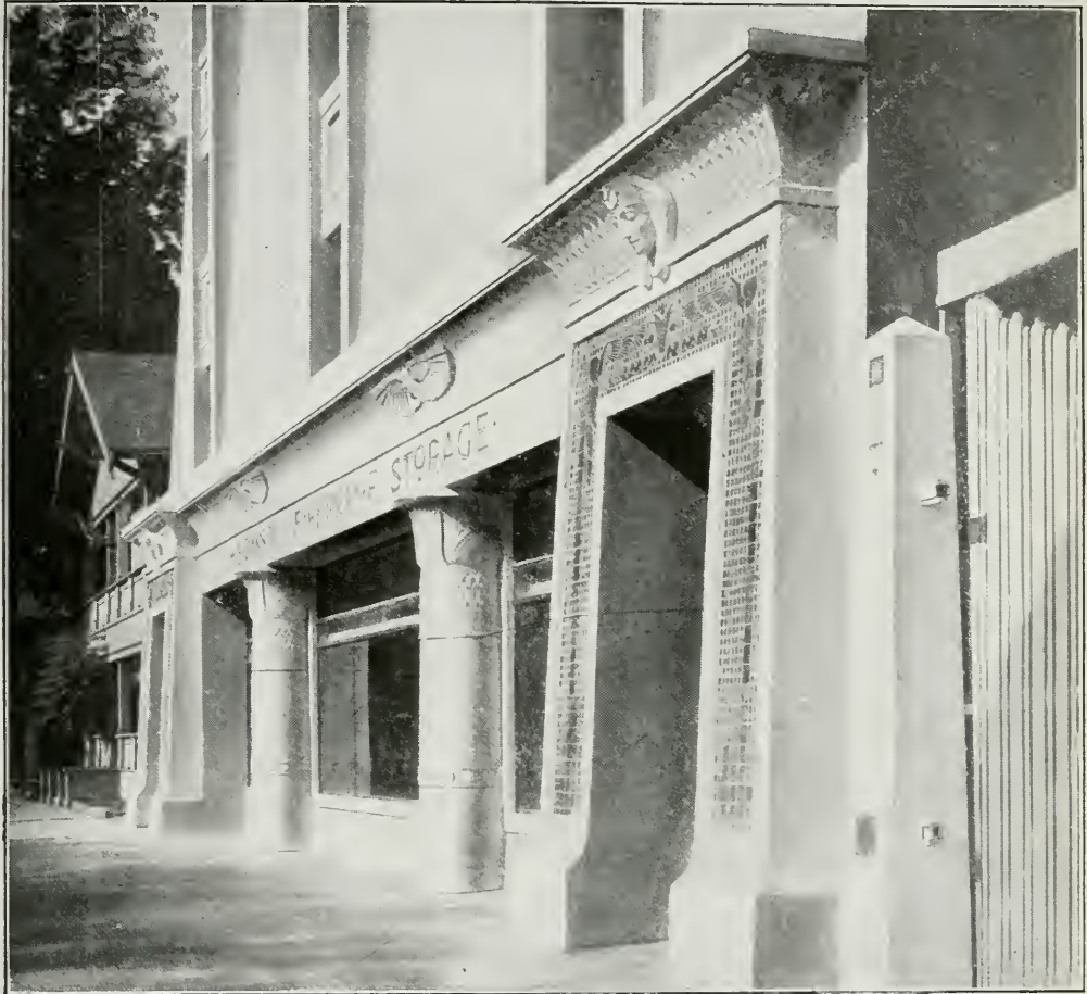
H. S. Dawson Storage Warehouse, Stockton, Cal., Glenn Allen, Architect
