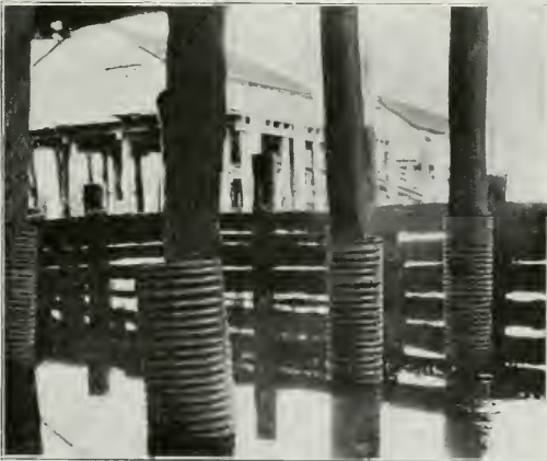
Armco Iron Corrugated Culvert Pipe used by the Bay City (Oregon) Fish and Storage Co., to protect its piers from the destructive Teredo.
