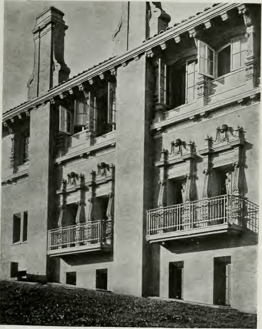
DETAIL OF SIDE, PRESIDENT'S HOUSE LELAND STANFORD JR. UNIVERSITY LOUIS CHRISTIAN MULLGARDT, ARCHITECT
