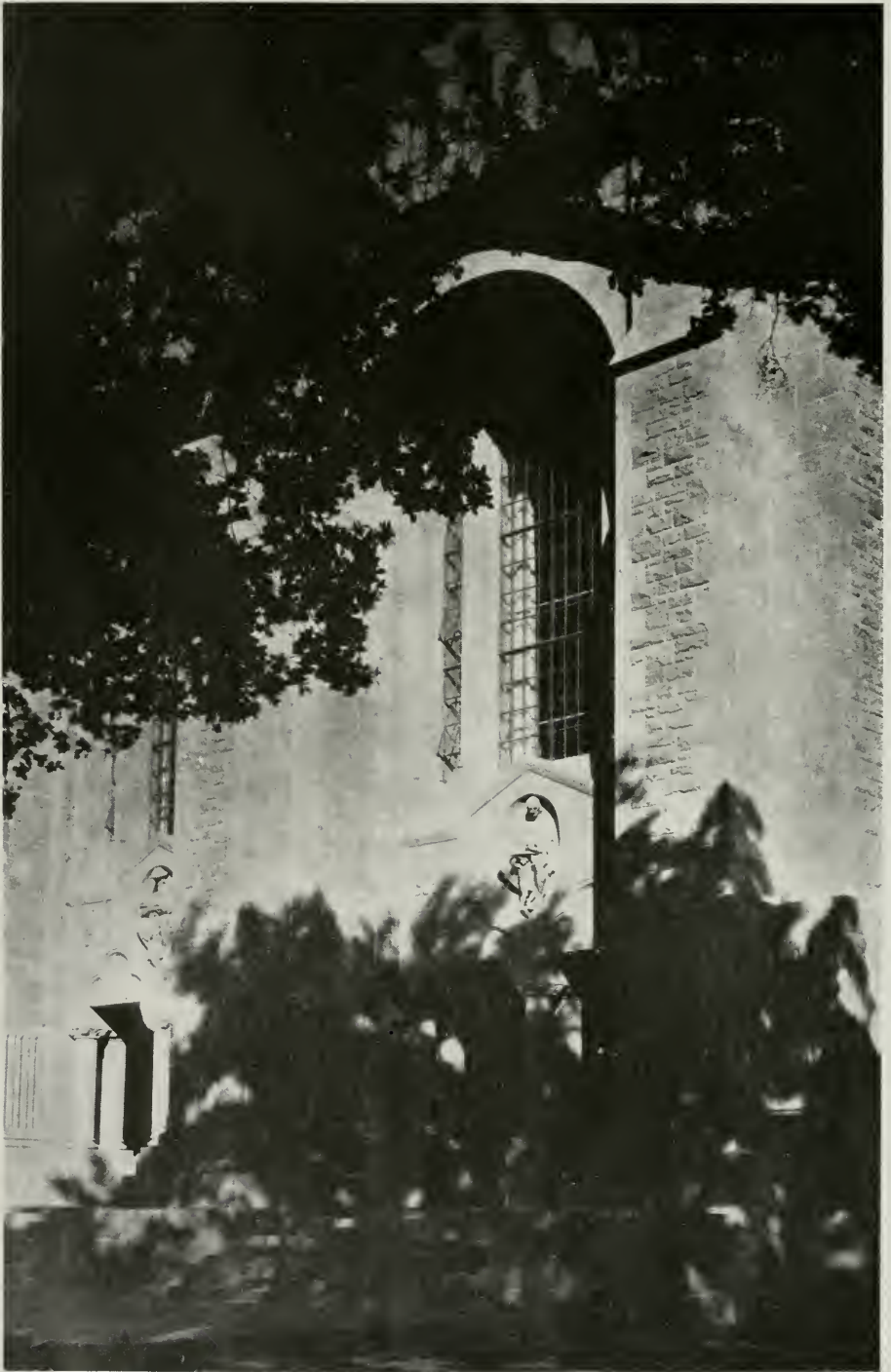
LIBRARY, LELAND STANFORD JR. UNIVERSITY BAKEWELL & BROWN, ARCHITECTS
