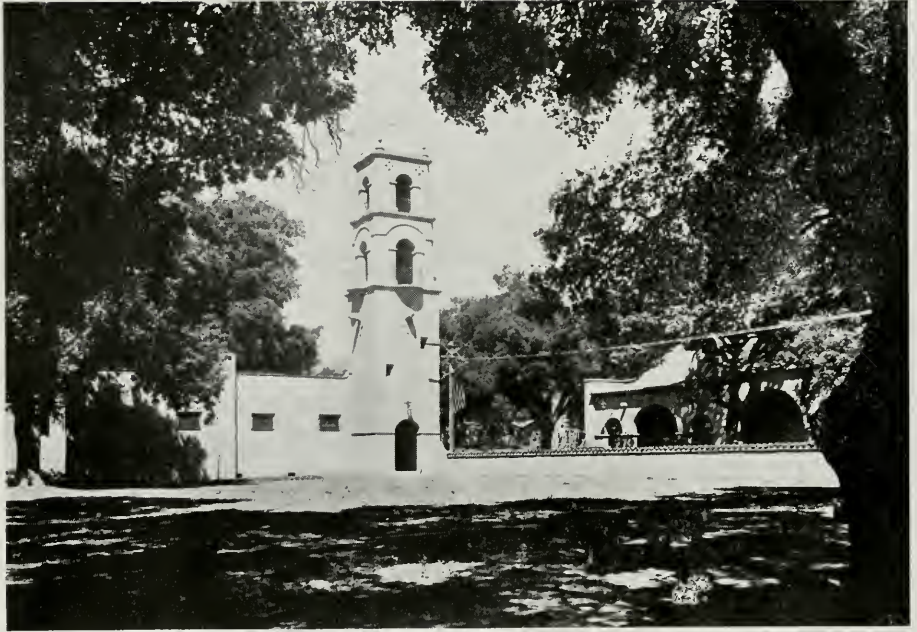
POST OFFICE AND TOWER, CIVIC IMPROVEMENT FOR OJAI, CALIFORNIA Mead & Requa, Architects
