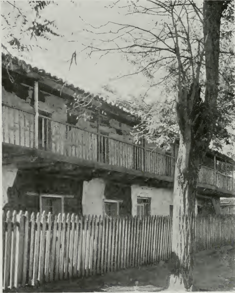
CASTRO HOUSE, SAN JUAN
