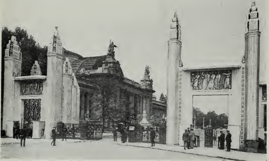
THE MAIN ENTRANCE GRILLE M. Brandt, Iron Worker
