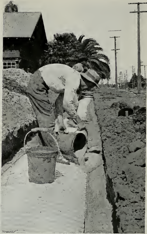
(Fig. 2) SHOWING METHOD OF INSURING A PERFECTLY SOLID BEARING AT THE BASE OF PART CIRCLE ARCHES.
