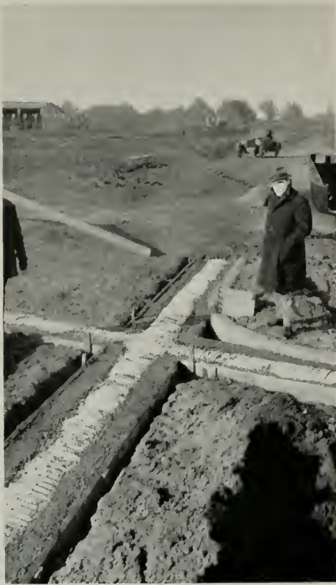
(Fig. 6) PART CIRCLE CULVERT AT INTERSECTION OF CALIFORNIA AND BAKER STREETS, BAKERSFIELD
