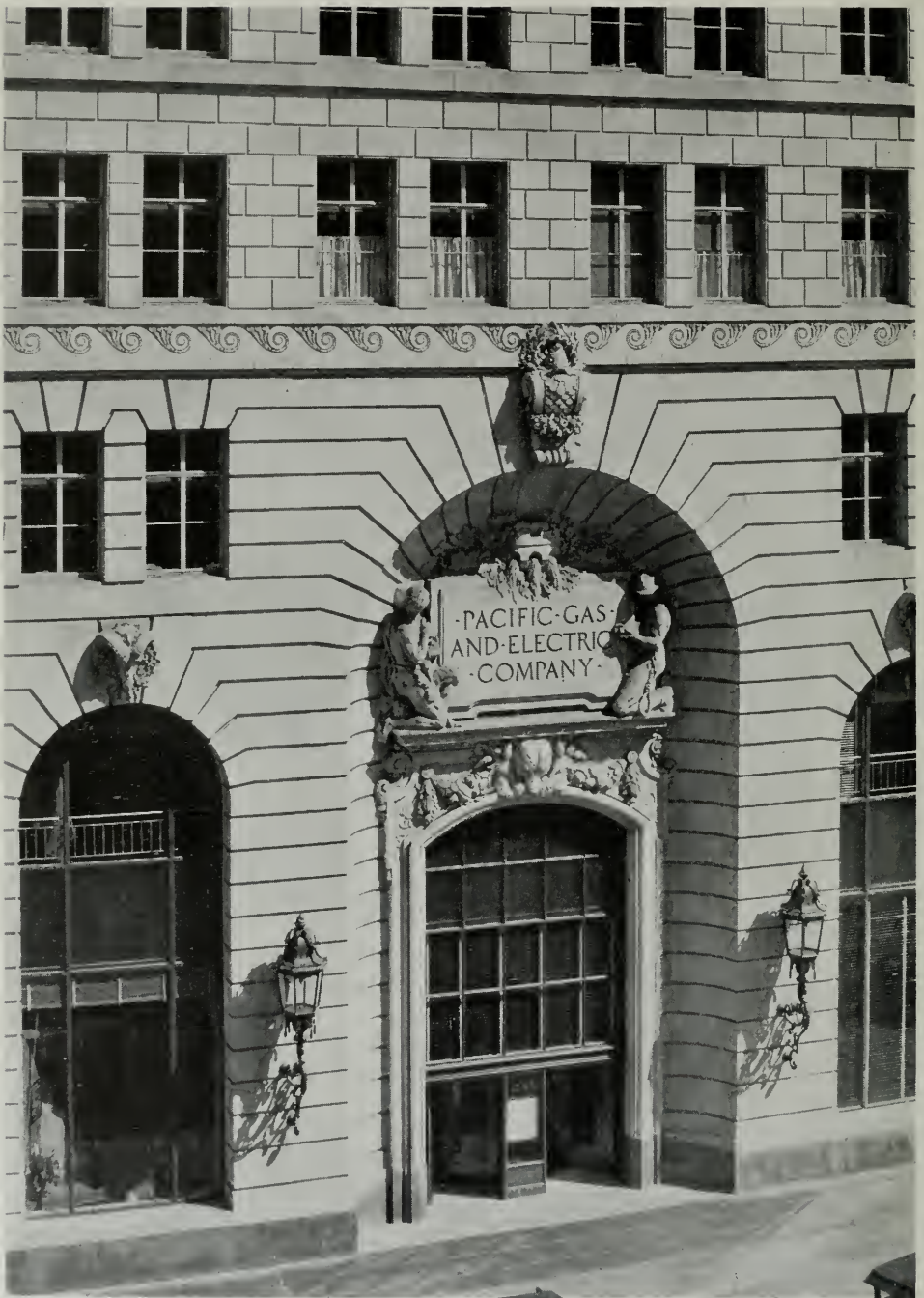
DETAIL MAIN ENTRANCE, P. G. & E. BUILDING BAKEWELL AND BROWN, ARCHITECTS
