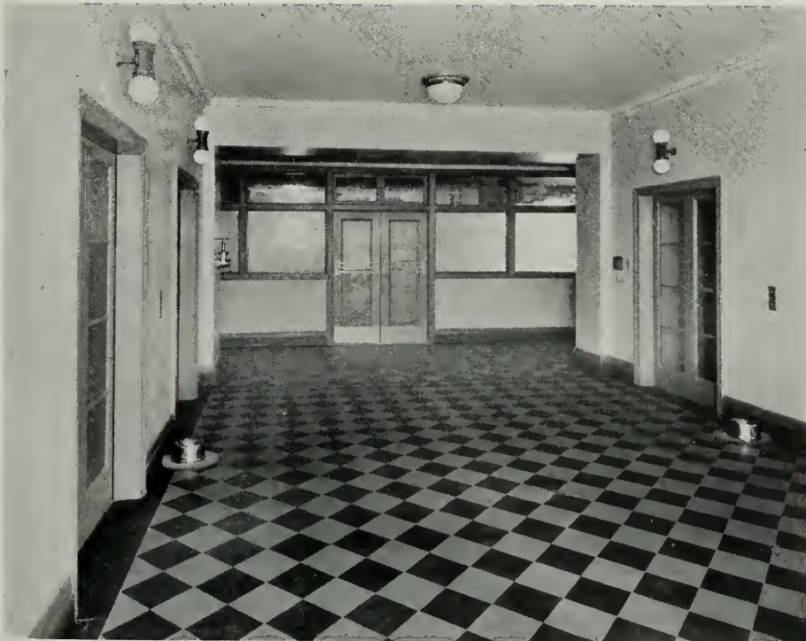
CORRIDORS AND MAIN FLOOR OFFICES OF NEW P. G. & E. BUILDING, SAN FRANCISCO, ARE LAID WITH BONDED FLOORS COLONIAL BUFF TREADLITE TILE
