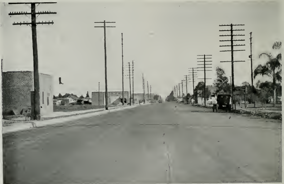
(Fig. 8) GARVEY AVENUE, MONTEREY PARK, AFTER IMPROVEMENTS SHOWN IN THE DRAWING (Page 123) WERE FINISHED Note smooth and uninterrupted surface
