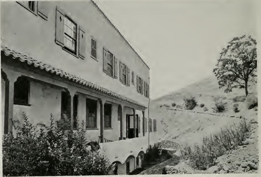
COVERED REAR ENTRANCE, ORINDA COUNTRY CLUB W. H. Crim, Jr., and Hamilton Murdock, Architects
