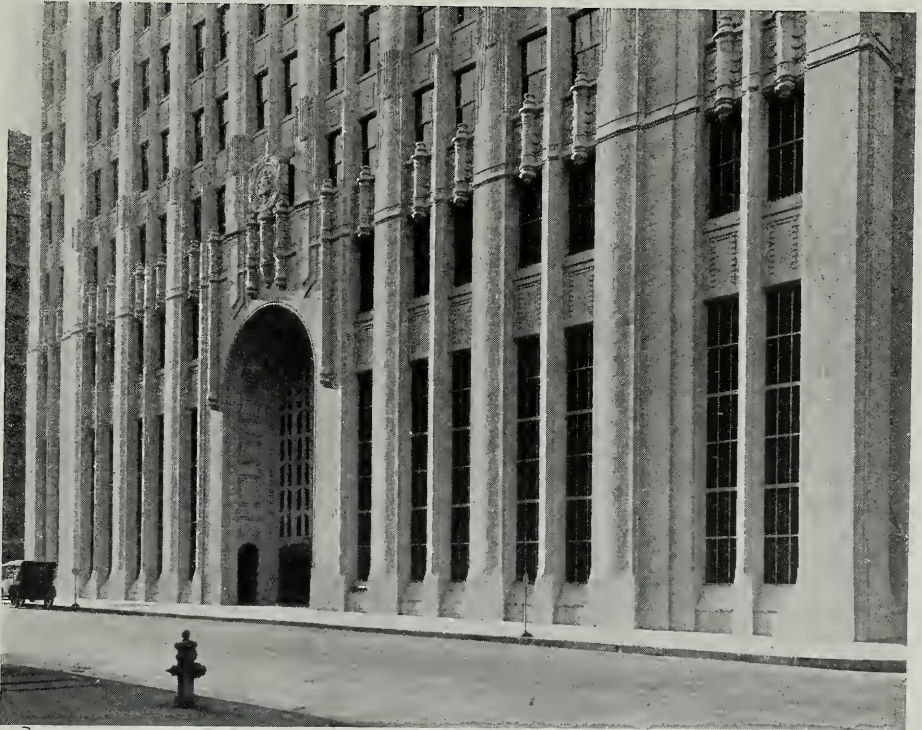
DETAIL BASE OF TELEPHONE BUILDING FROM NEW MONTGOMERY STREET J. R. Miller and T. L. Pflueger, A. A. Cantin, Associated Architects
