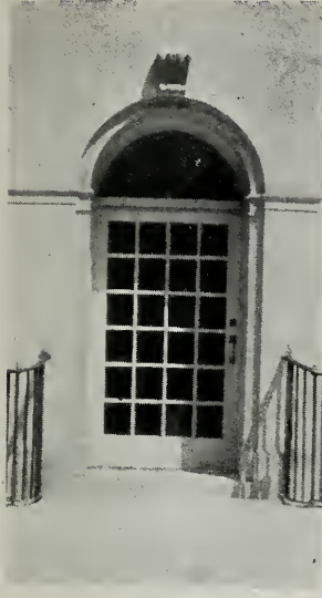
A French doorway with simple architectural treatment.
