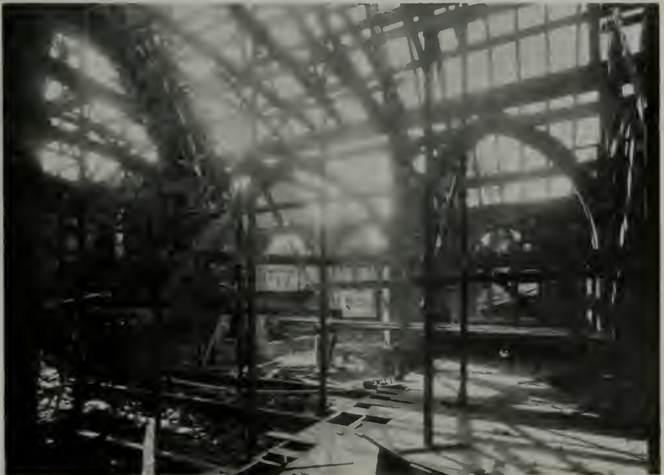
PROGRESS PICTURE, INTERIOR OF ST. PAUL'S CHURCH
