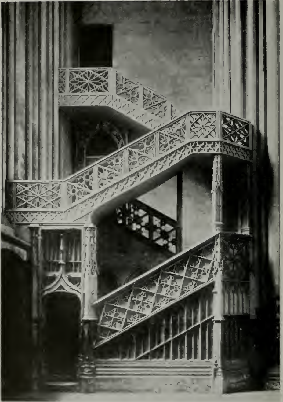
FIG. 1 STAIRWAY IN CATHEDRAL OF ROUEN
