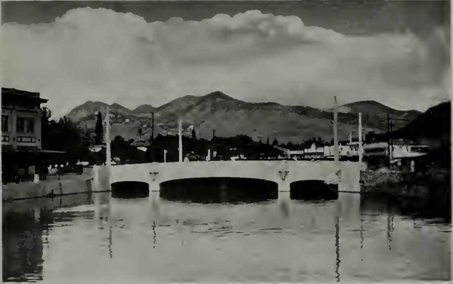
KING STREET BRIDGE, HONOLULU, H. T. Hart Wood, Architect
