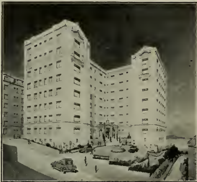
TOWNHOUSE APARTMENTS, LOS ANGELES Weir Electric Heaters Used Throughout
