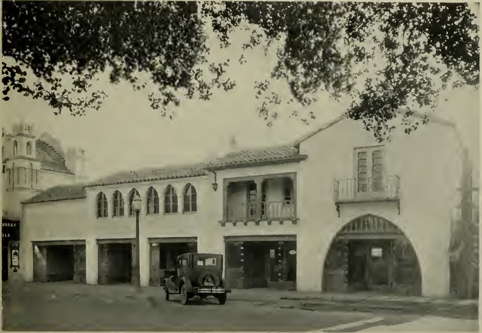
UNIVERSITY AVENUE SHOPS, PALO ALTO Birge N. Clark, Architect
