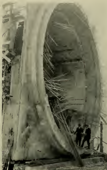
END OF COMPLETED CONCRETE SEGMENT Showing Collar and Inside Joint Lap Reinforcement
