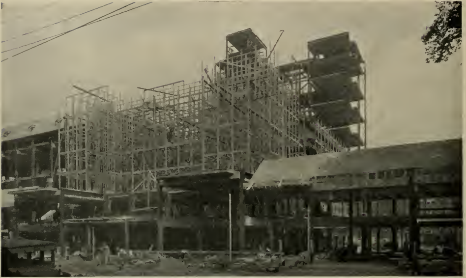
YALE UNIVERSITY LIBRARY, NEW HAVEN CONNECTICUT Arc Welded Construction Under Westinghouse Supervision
