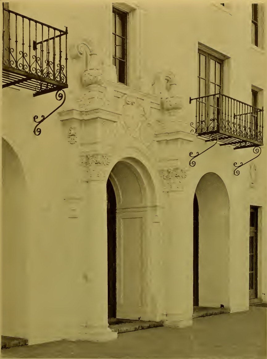
ENTRANCE DETAIL, CENTRAL DORMITORY, ST. MARY'S COLLEGE JOHN J. DONOVAN, ARCHITECT
