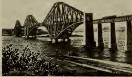
FIRTH OF FORTH BRIDGE
