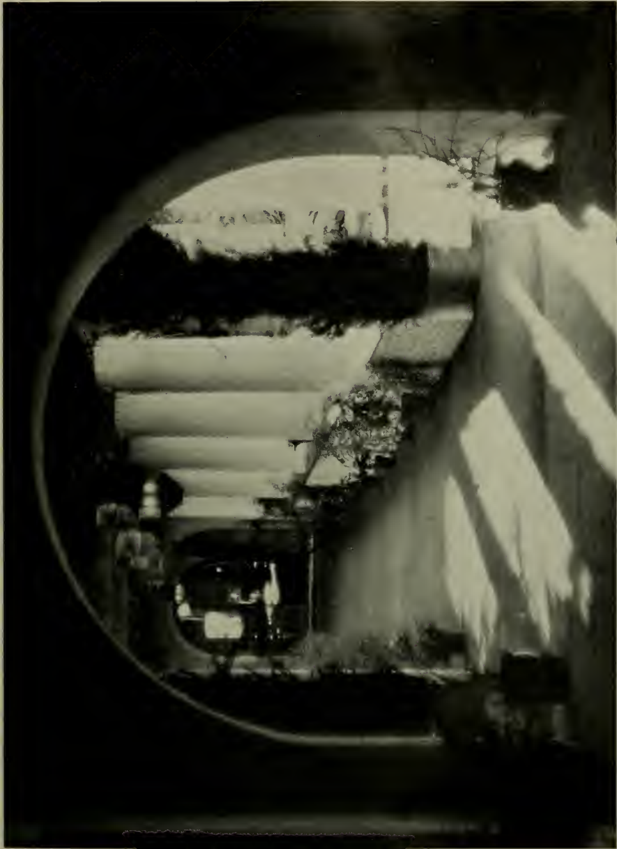
NORTH PATIO, SANTA BARBARA BILTMORE HOTEL REGINALD D. JOHNSON, ARCHITECT
