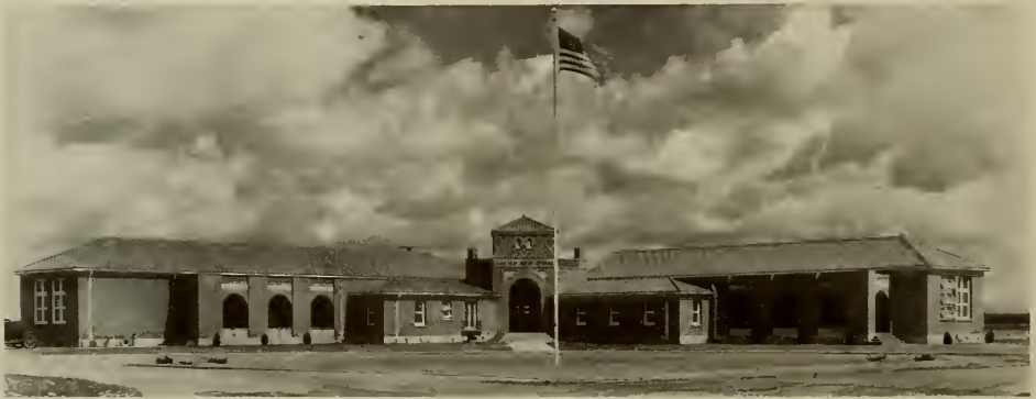
BEARDSLEY SCHOOL BUILDING, KERN COUNTY, CALIFORNIA Symmes and Cullimore, Architects
