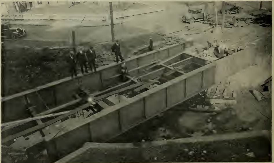
FIRST WELDED PLATE GIRDER BRIDGE, TURTLE CREEK, PENNSYLVANIA
