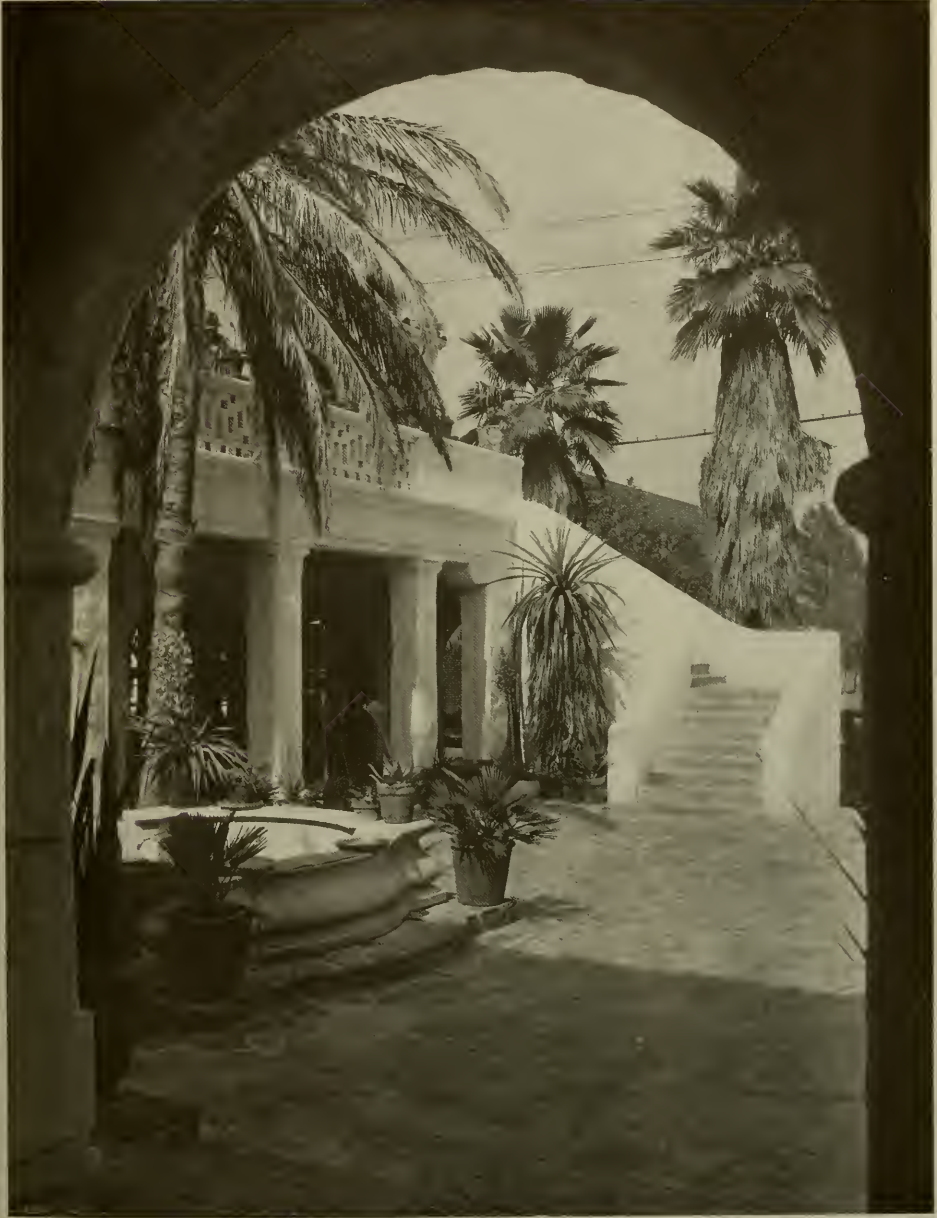
FOUNTAIN AND STAIRWAY, PASADENA COMMUNITY PLAYHOUSE, PASADENA ELMER GREY, ARCHITECT
