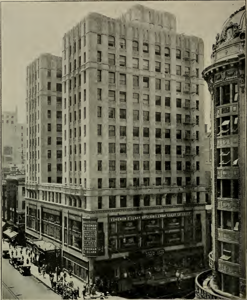
Foreman & Clark Building, Los Angeles, Cal. Cuslett & Beelman, Architects. J. V. McNeil Co., Builder. Variegated Indiana Limestone.
