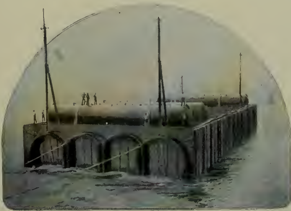
PICTURE SHOWS PROCESS CARRIED OUT IN BUILDING A PORTION OF THE NEW YORK SUBWAY THAT GOES UNDER THE HARLEM RIVER
