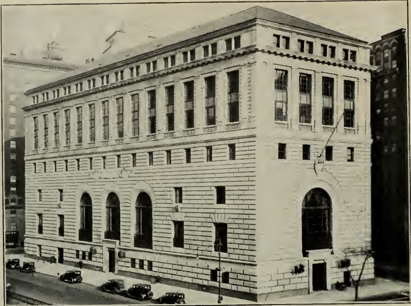
Central Savings Bank, New York City. York & Sawyer, Architects. Hegeman-Harris Co., Builders. Built of Variegated and Rustic Buff Indiana Limestone.
