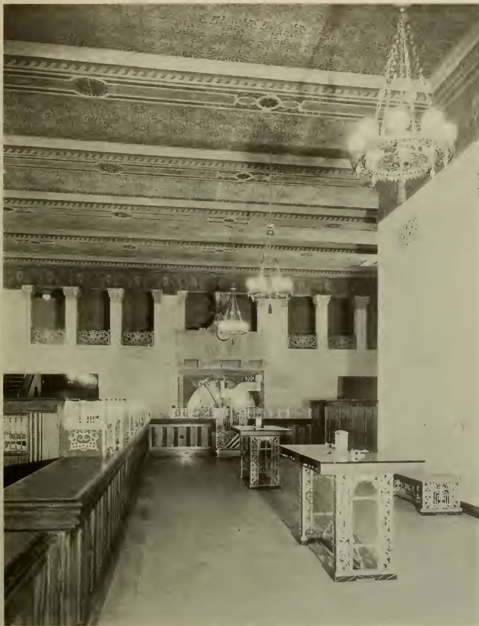
BANKING ROOM, SECURITY TRUST AND SAVINGS BANK, SAN PEDRO ALFRED F. PRIEST, ARCHITECT
