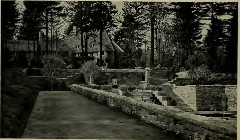
UPPER TERRACES, ESTATE OF M. LLOYD FRANK, PORTLAND, OREGON Herman Brookman, Architect
