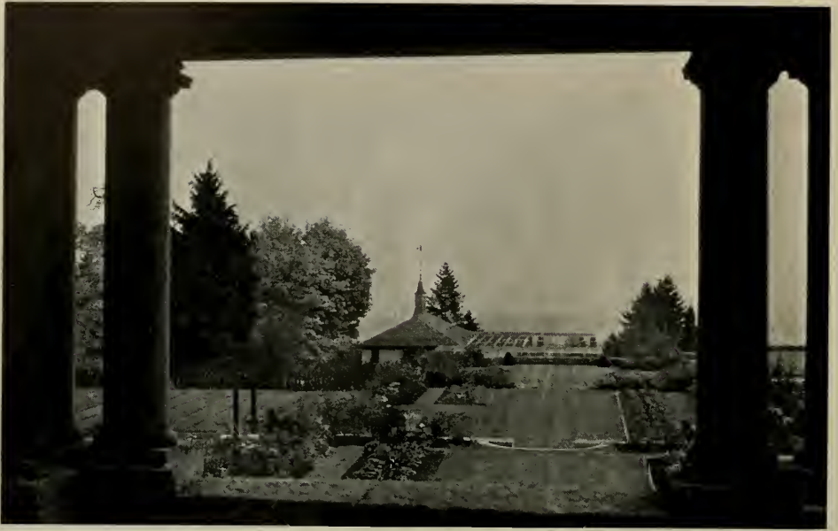
LOOKING FROM GAZABO TO BATH HOUSE, ESTATE OF M. LLOYD FRANK Herman Brookman, Architect
