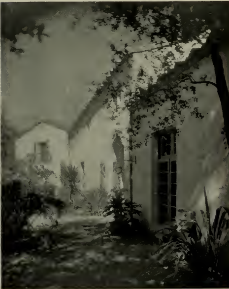
GARDEN VIEW, HOUSE OF F. Q. STANTON, FLINTRIDGE Stanton, Reed & Hibbard, Architects
